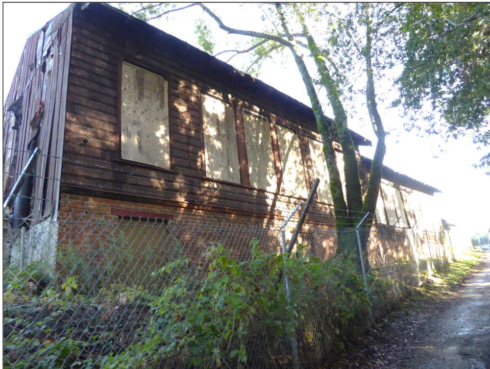
Photograph 6: West end of south wall showing wood shingle over brick veneer siding; camera facing northeast, December 17, 2018.
