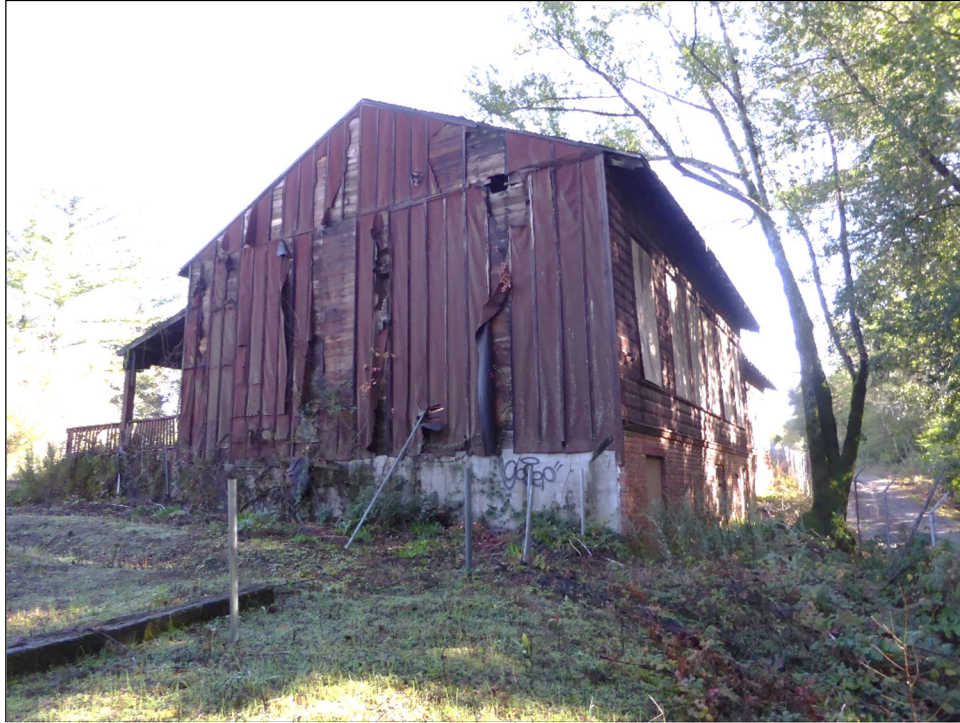
Photograph 5: West wall showing deteriorated siding; camera facing east, December 17, 2018.
