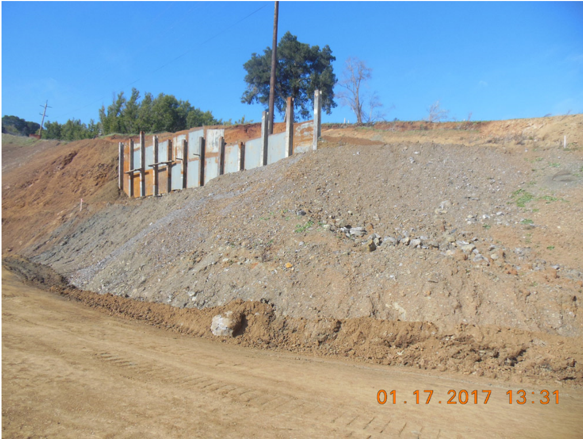
Photo 12 (taken 1-17-2017): Retaining wall on north high wall.
