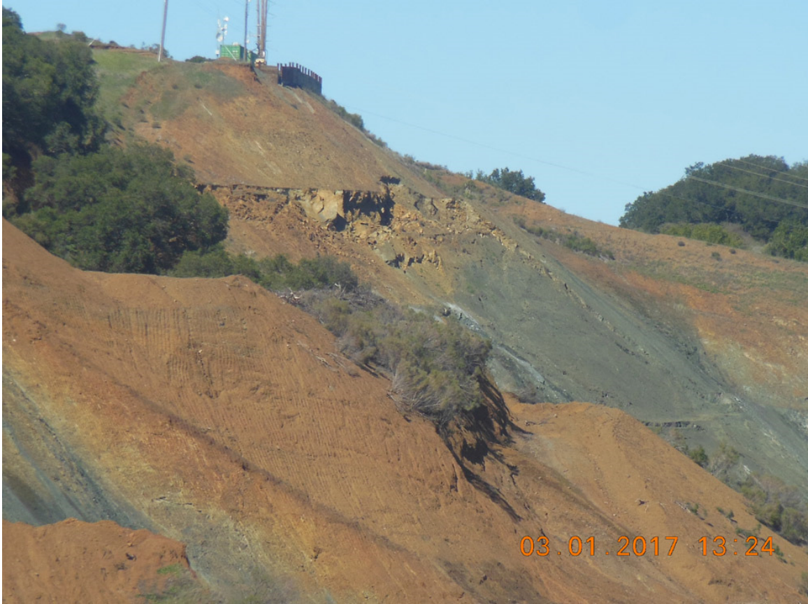
Photo 14 (taken 3-1-2017): Slope failure on western high cut wall.
