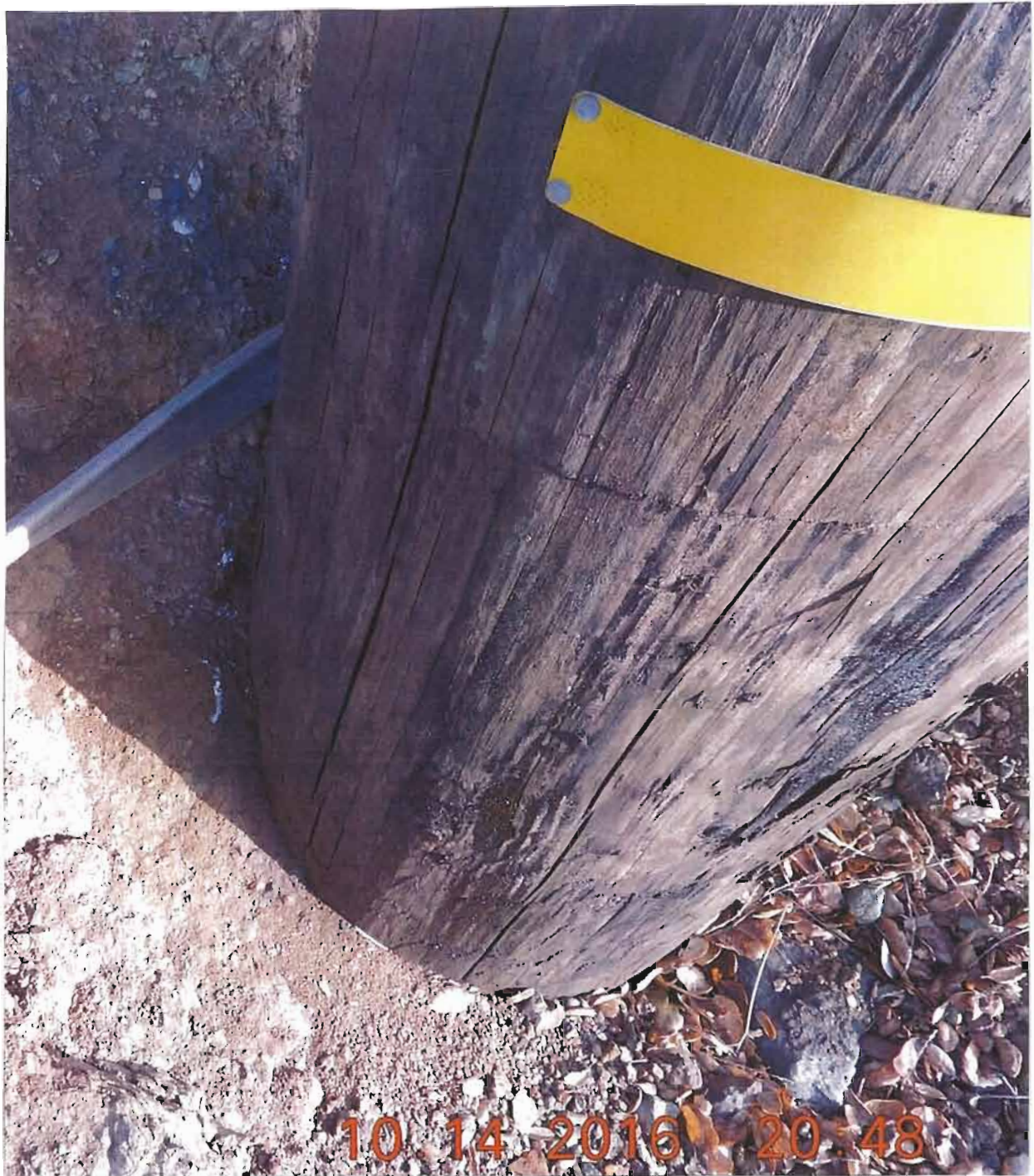
No Annular Void around Power Pole And No significant Tilt
