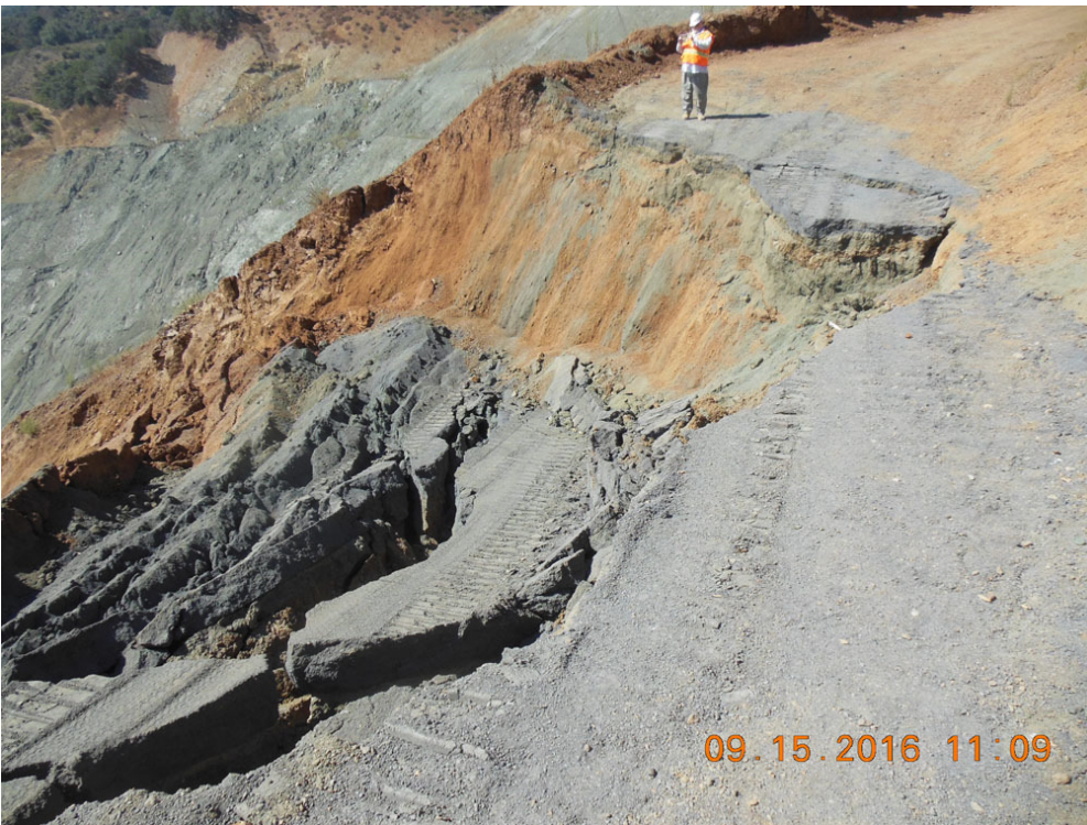
Photo 8 (taken 9-15-2016): Headscarp of failure on north high wall and perimeter road.
