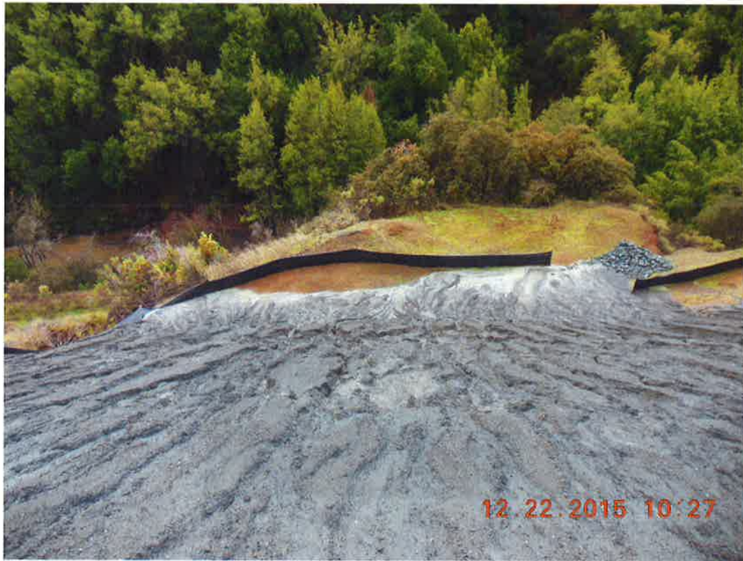
Erosion, runoff to Montebello Creek (Photo by S. Beams)
