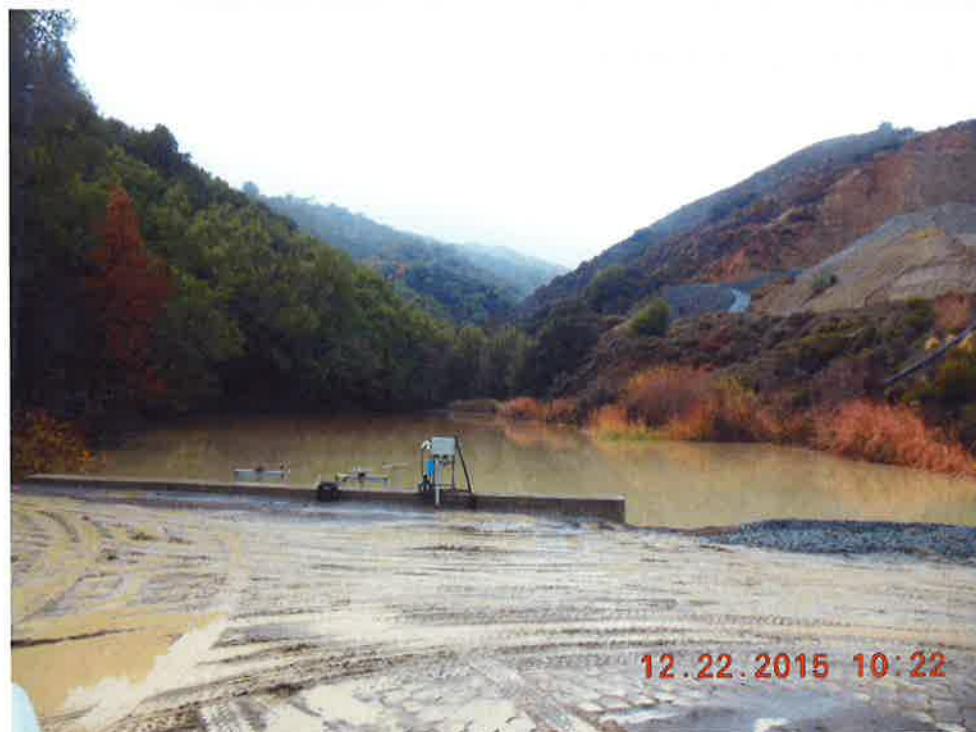
Upper Settling Basin, fill slope in distance. (Photo by S. Beams)
