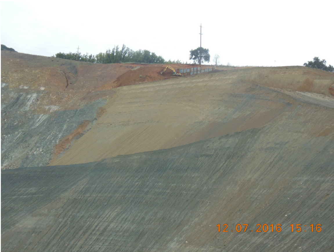
Photo 11 (taken 12-07-2016): Buttress fill below retaining wall on north high wall.
