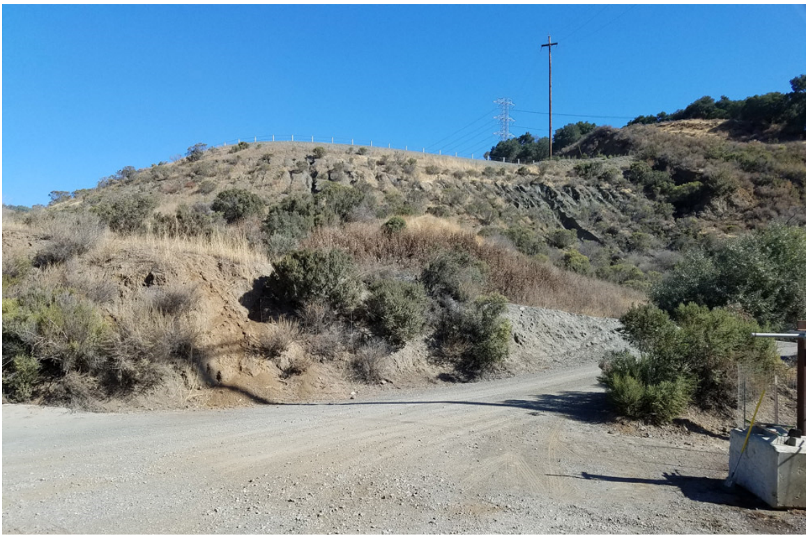
Photo 6 (taken 9-15-2016): Erosion rills on fill slope above main haul road.
