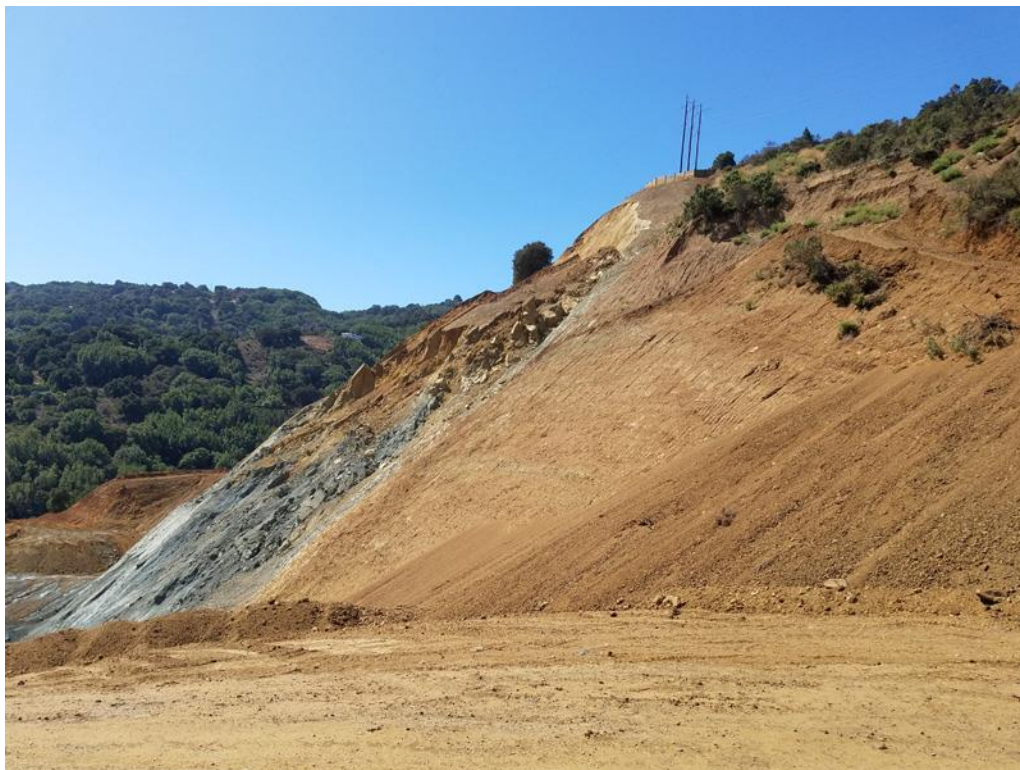
Photo 8 - Side view of Southwest Slope Failure (taken September 14, 2017)
