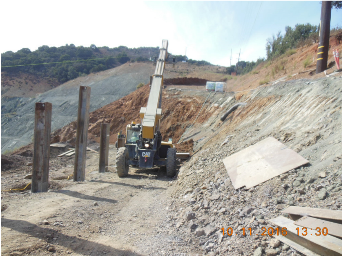
Photo 9 (taken 10-11-2016): Construction of retaining wall on north high wall.
