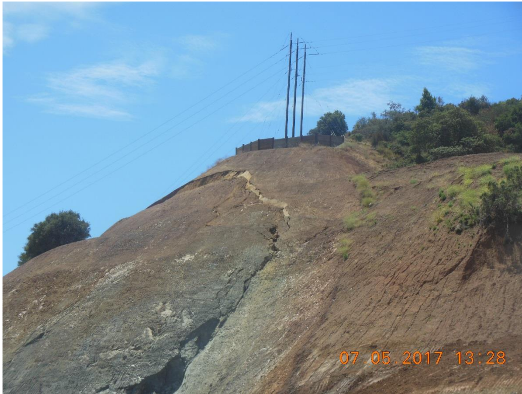
Photo 7 - Side view of Southwest Slope Failure (taken July 5, 2017)
