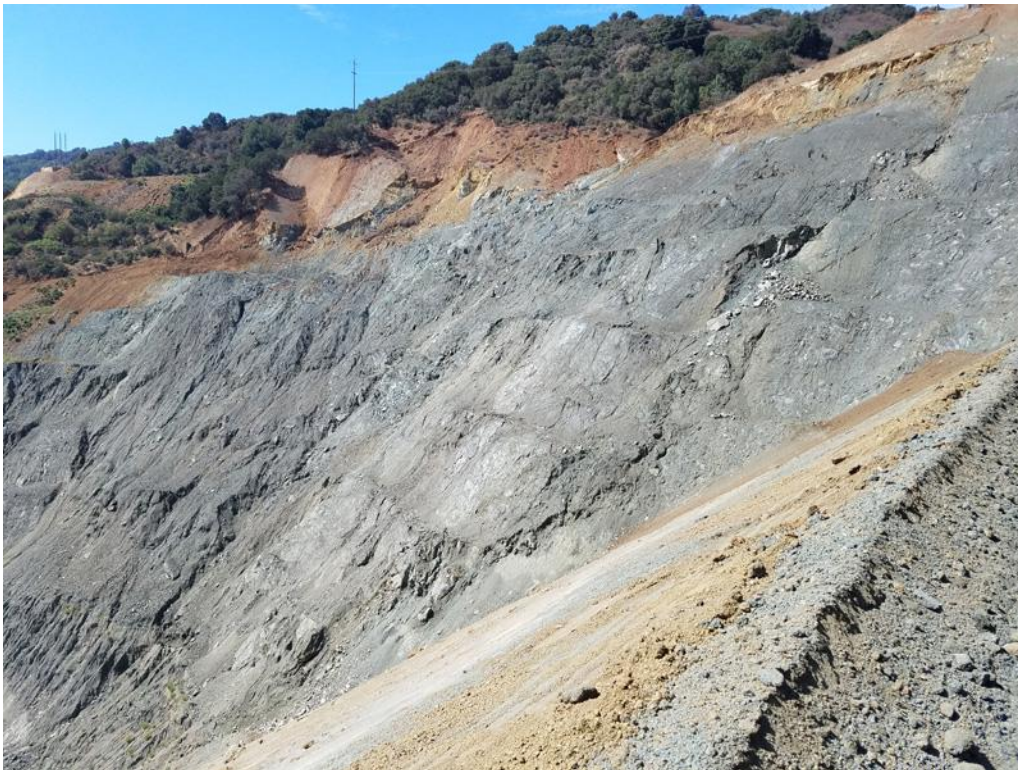
Photo 4 - Side view of Northwest Slope Failure (taken September 14, 2017)
