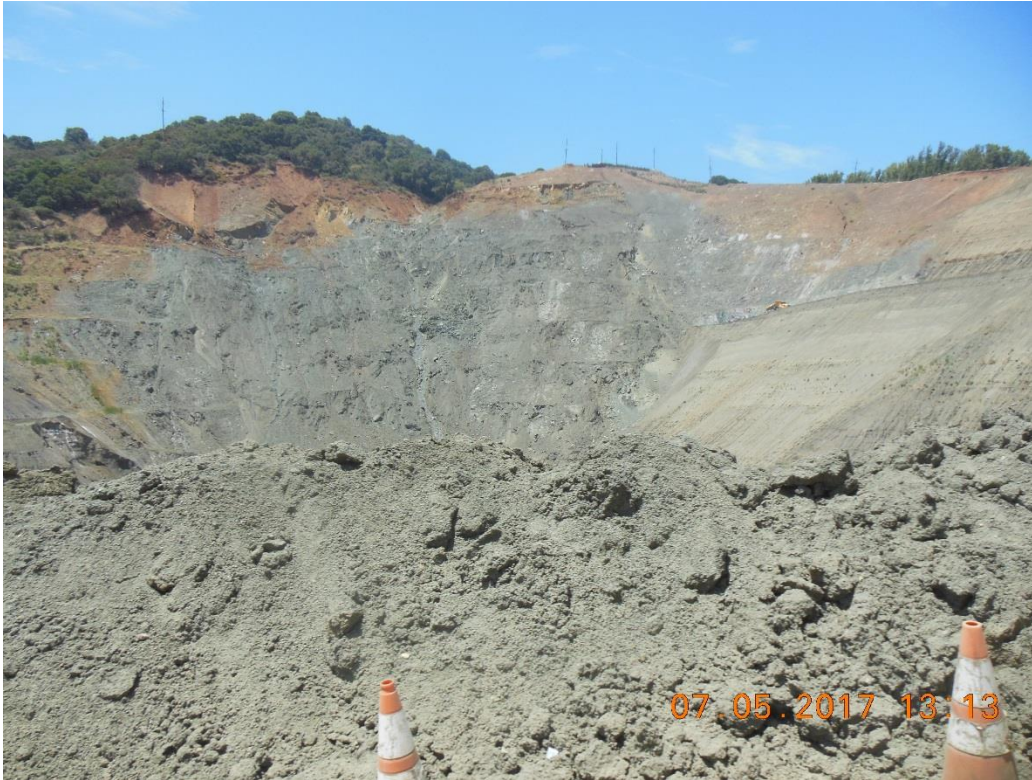
Photo 1 - Northwest Slope Failure (taken July 5, 2017)
