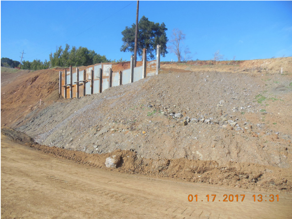
Photo 12 (taken 1-17-2017): Retaining wall on north high wall.
