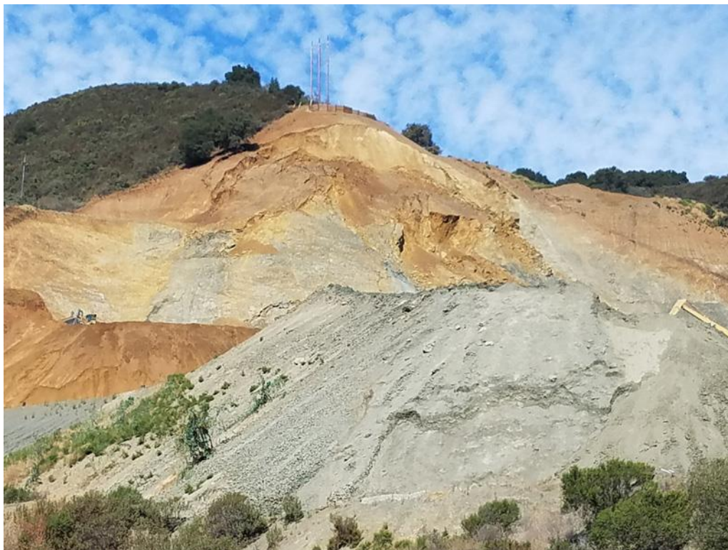
Photo 6 - Southwest Slope Failure (taken September 14, 2017)
