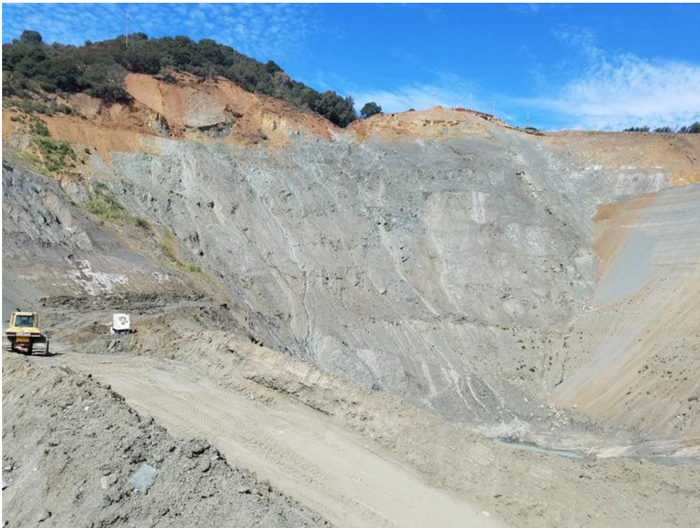
Photo 2 - Northwest Slope Failure (taken September 14, 2017)
