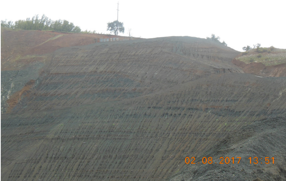
Photo 13 (taken 2-8-2017): Buttress fill below retaining wall on north high wall.
