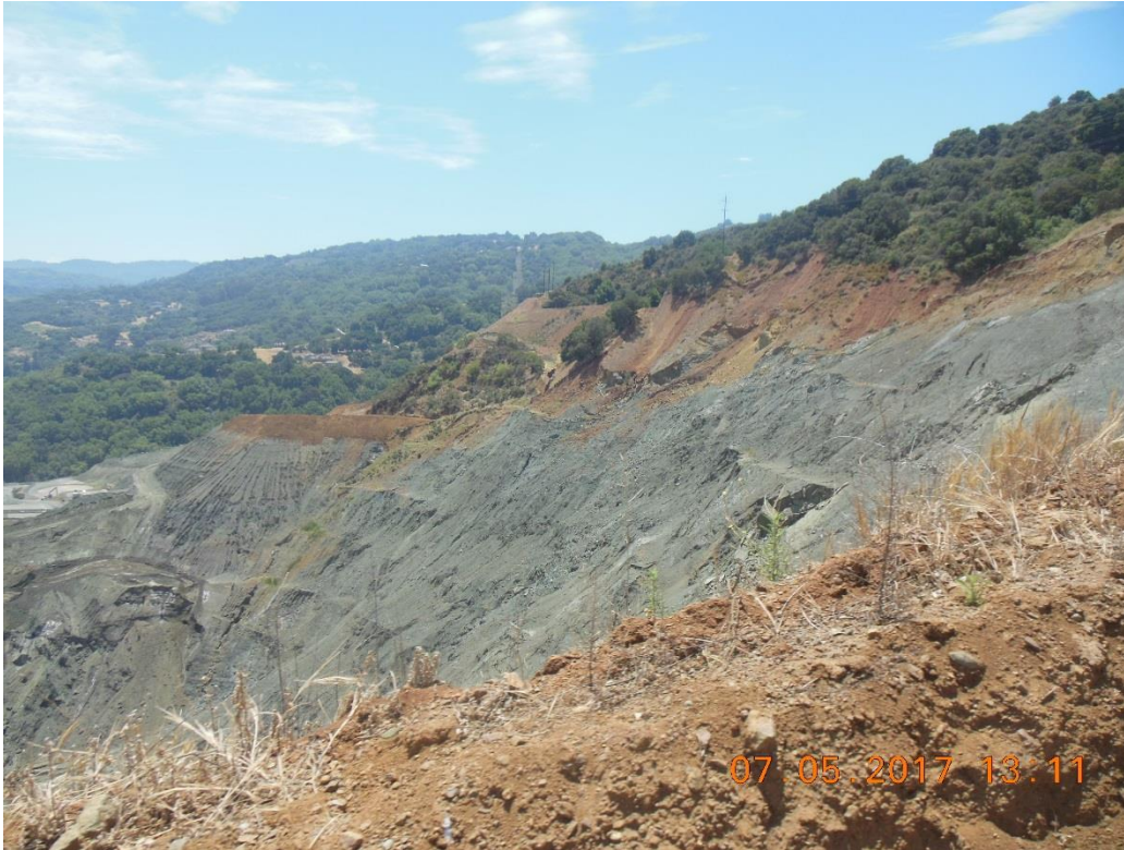
Photo 3 - Side view of Northwest Slope Failure (taken July 5, 2017)
