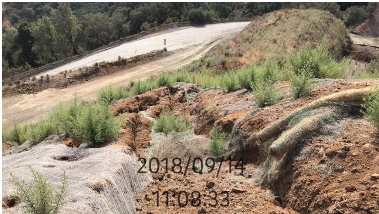
Photo 11: Ground crack on east-facing fill slope near northeastern corner of property. Haul road to Lehigh visible.
