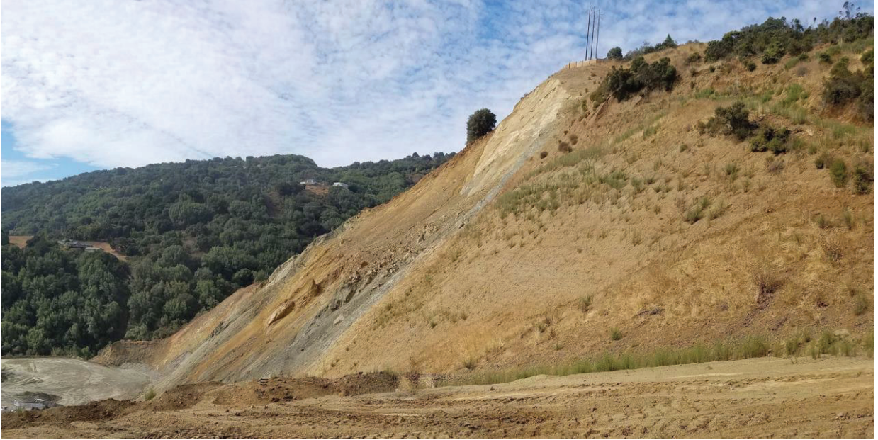
Photo 18: Slope failure on southwestern high cut wall, looking south. (Profile view)
