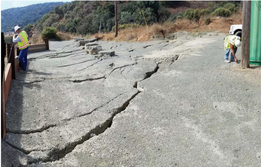
Photo 16: Ground cracks and subsidence at northwest property line.
