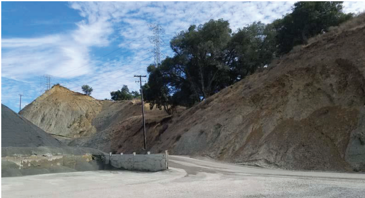
Photo 21: Shallow failures of cut slope along east side of Parcel B.
