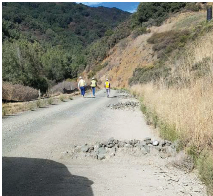
Photo 29: Check dams along road by northside of Rattlesnake Creek.
