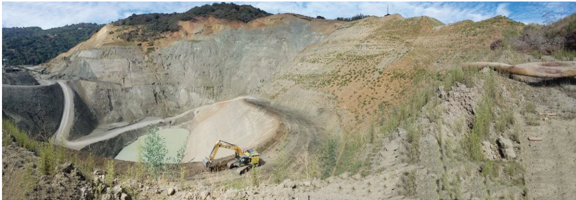
Photo 13: Buttress fill on north high wall. West side of pit visible on the left.
