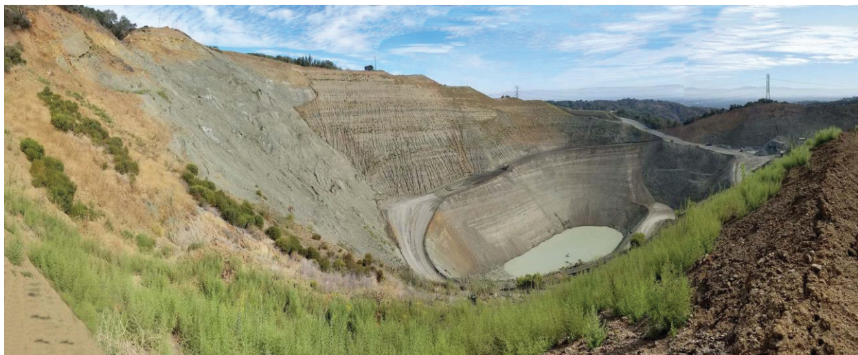
Photo 12: Buttress fill on north high wall. West side of pit visible on the left.
