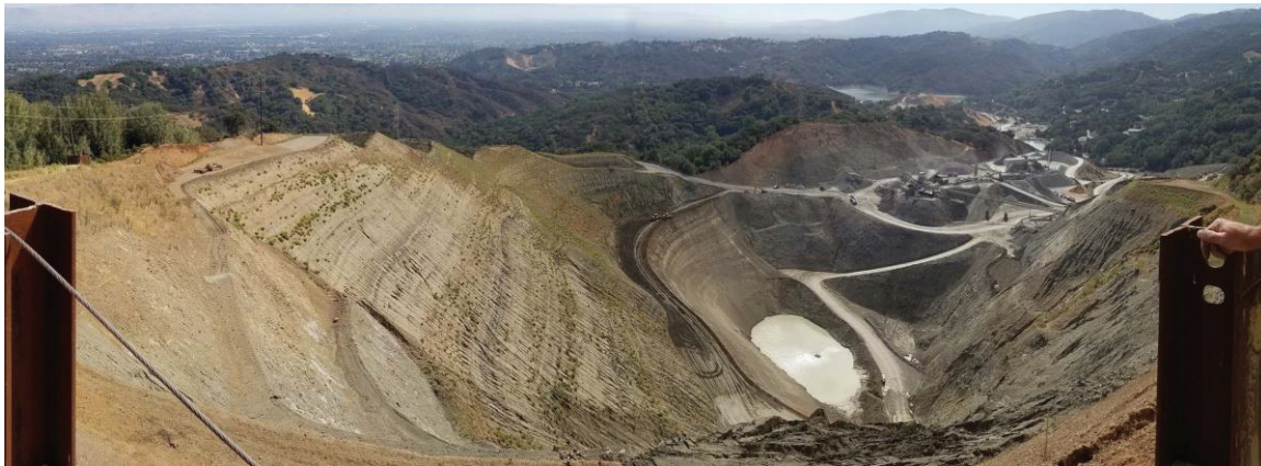
Photo 14: Panorama of buttress fill below retaining wall on northwest high wall.
