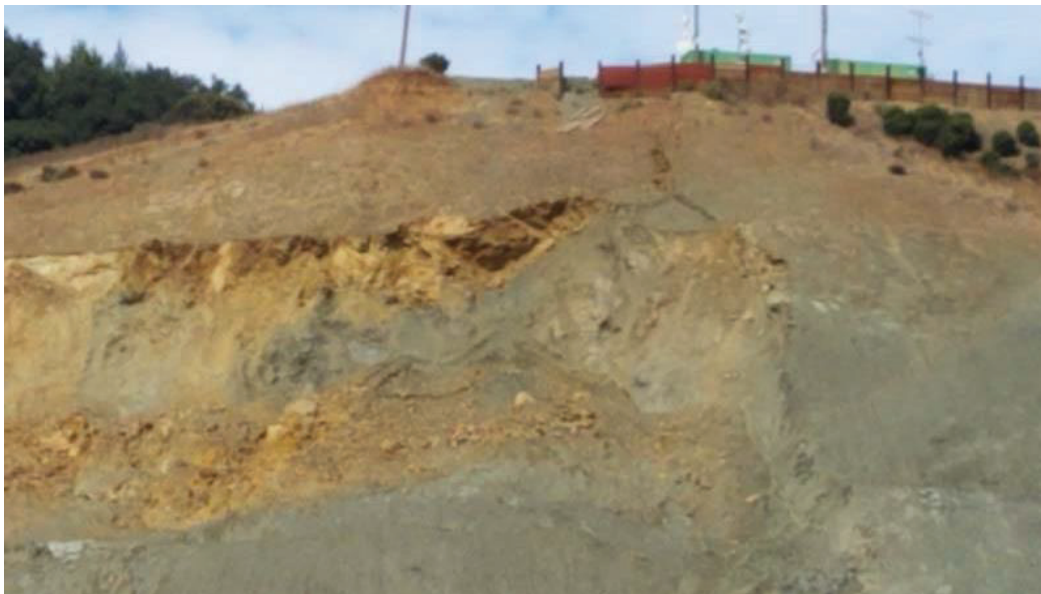
Photo 15: Slope failure on western high cut wall.
