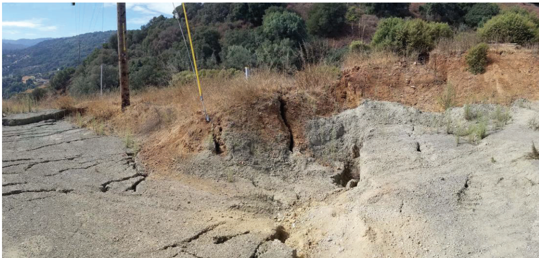
Photo 17: Ground cracks and headscarp beyond northwest property line.
