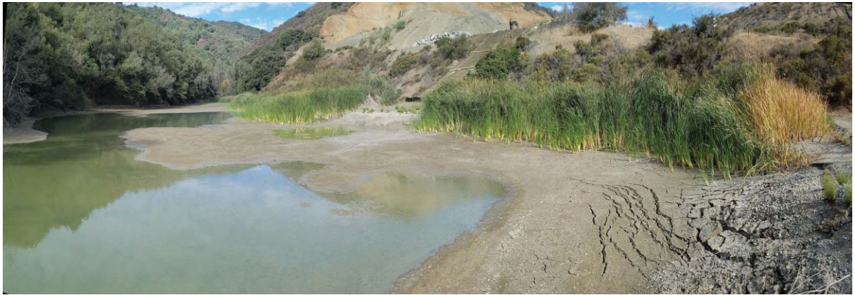
Photo 25: Upper Settling Basin showing area where discharge pipe was removed and straw wattles placed.
