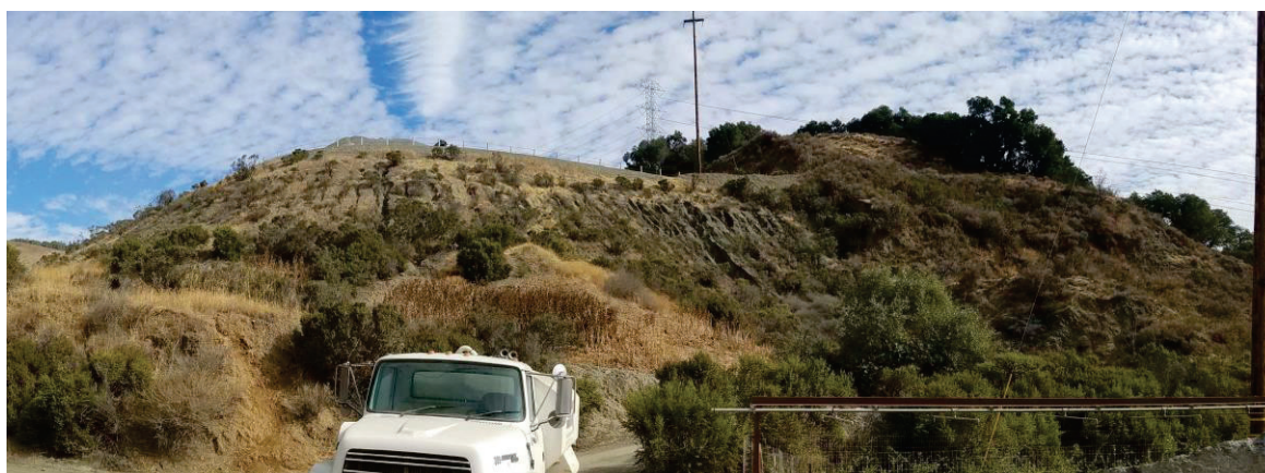
Photo 6: Erosion rills on fill slope above main haul road.
