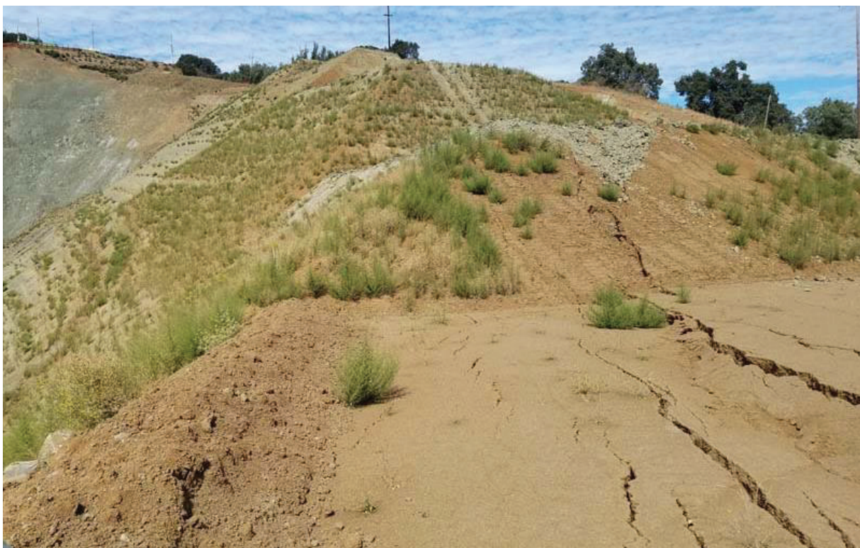
Photo 10: Ground crack on top of buttress fill of north high wall.
