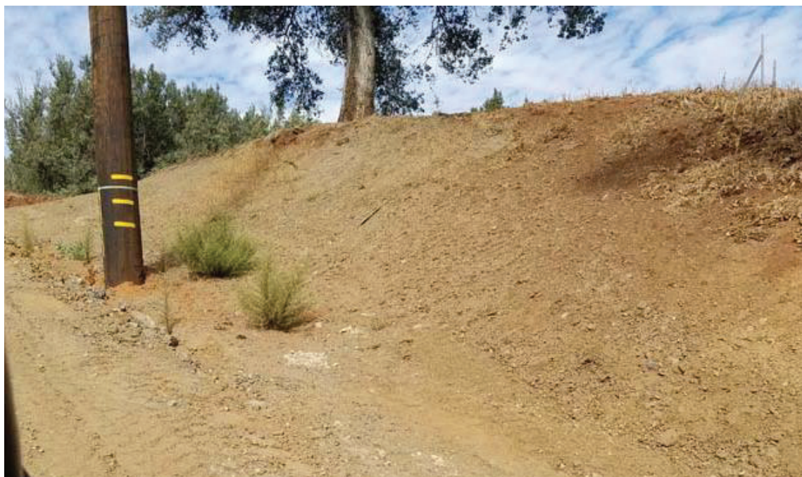
Photo 8: North perimeter road cut slope. Grading has obliterated the ground movement cracks observed in 2017.
