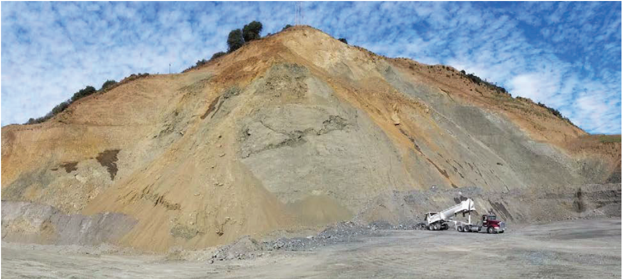
Photo 19: Slope failure on southwestern high cut wall, looking west. (Head-on view)
