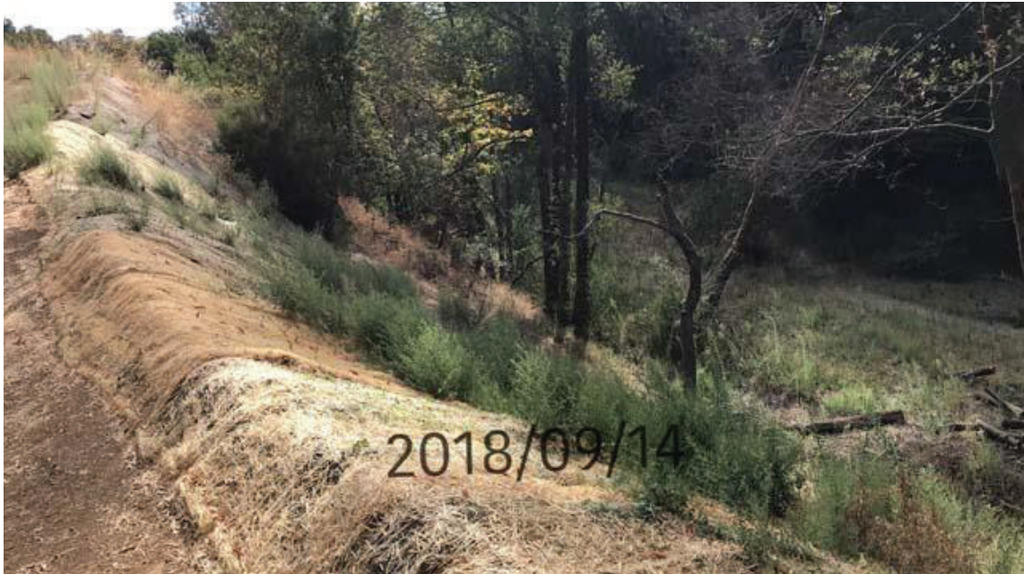
Photo 20: Regraded slope along the north side of Rattlesnake Creek.
