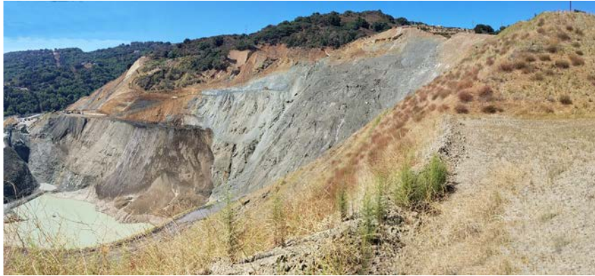
Photo 13: Buttress fill on north high wall. West side of pit visible on the left.
