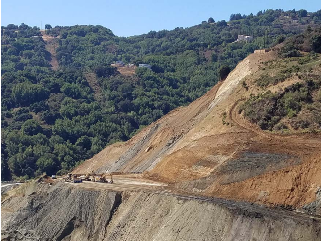
Photo 18: Slope failure on southwestern high cut wall, looking south. (Profile view)
