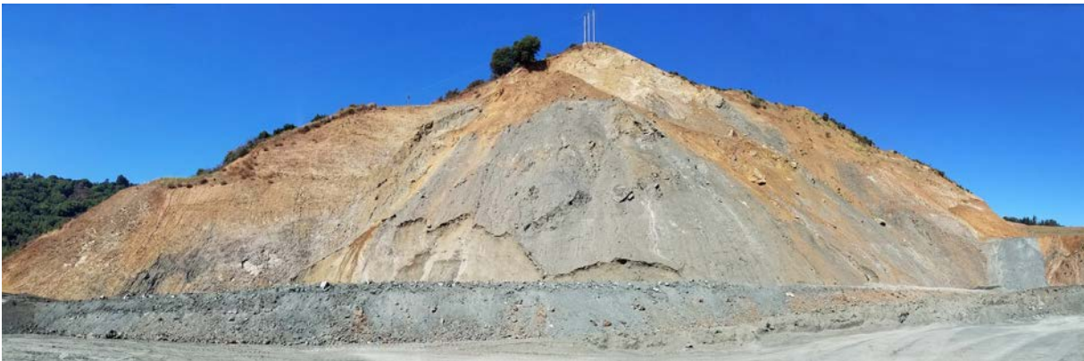
Photo 19: Slope failure on southwestern high cut wall, looking west. (Head-on view)
