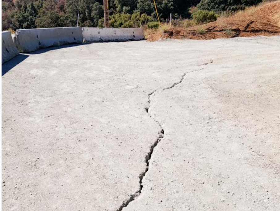
Photo 16: Ground cracks near northwest property line.
