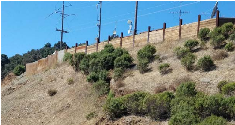
Photo 15: Slope failure on western high cut wall.
