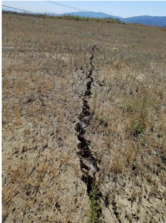
Photo 10: Ground crack on top of buttress fill of north high wall.
