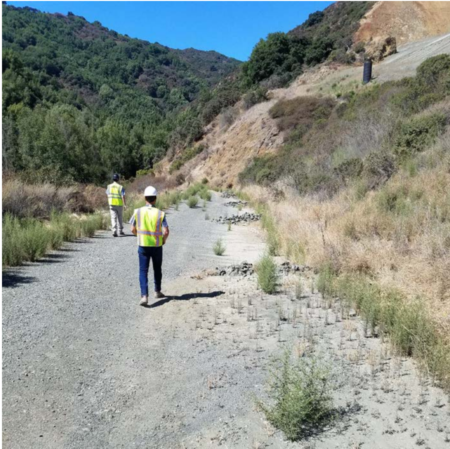
Photo 29: Check dams along road by northside of Rattlesnake Creek.
