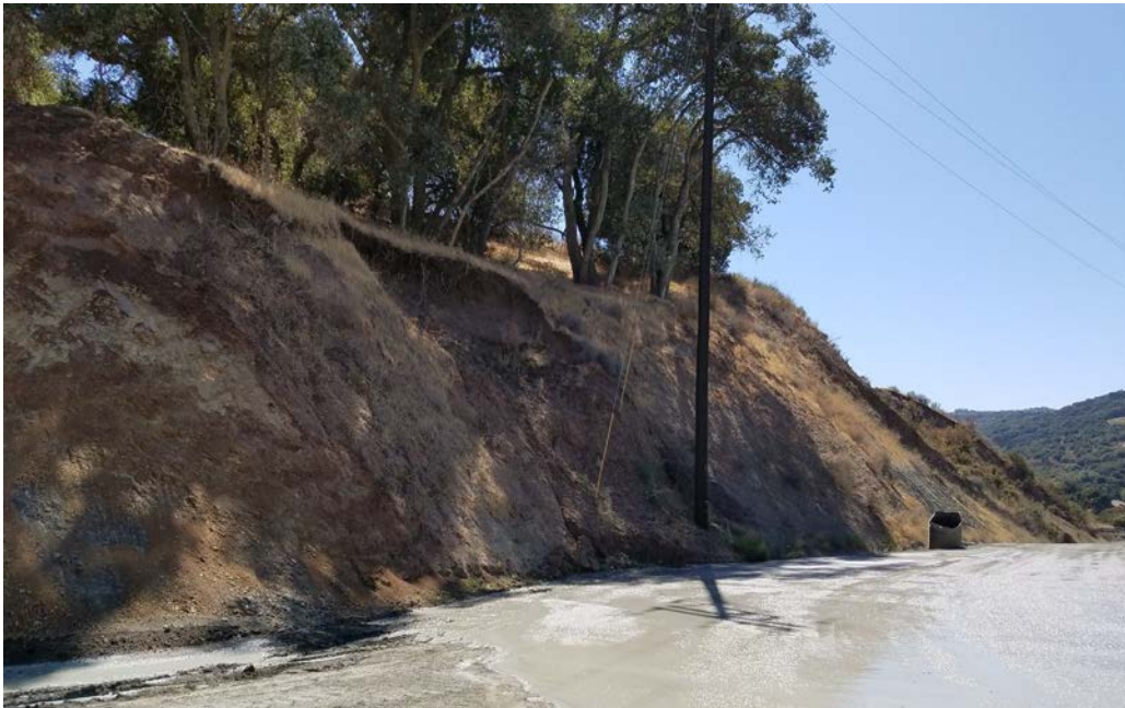
Photo 21: Shallow failures of cut slope along east side of Parcel B.
