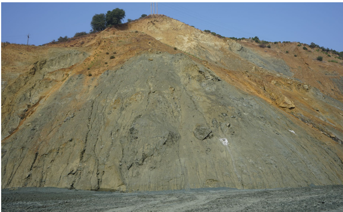
Photo 20: Slope failure on southwestern high cut wall, looking west. (Head-on view)
