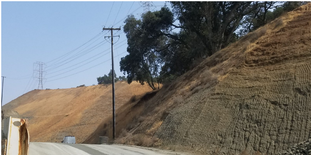
Photo 22: Shallow failures of cut slope along east side of Parcel B.
