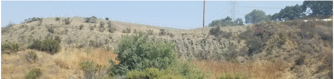
Photo 7: Erosion rills on fill slope above main haul road.
