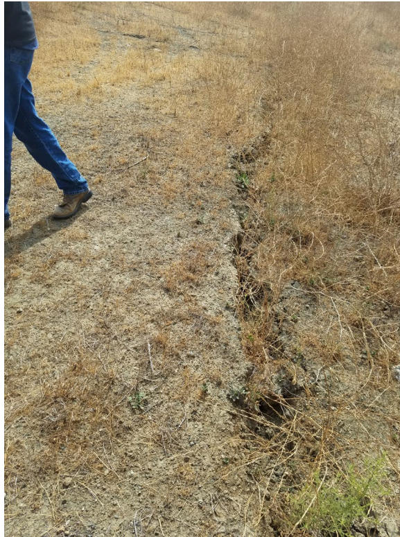
Photo 11: Ground crack on top of buttress fill of north high wall.
