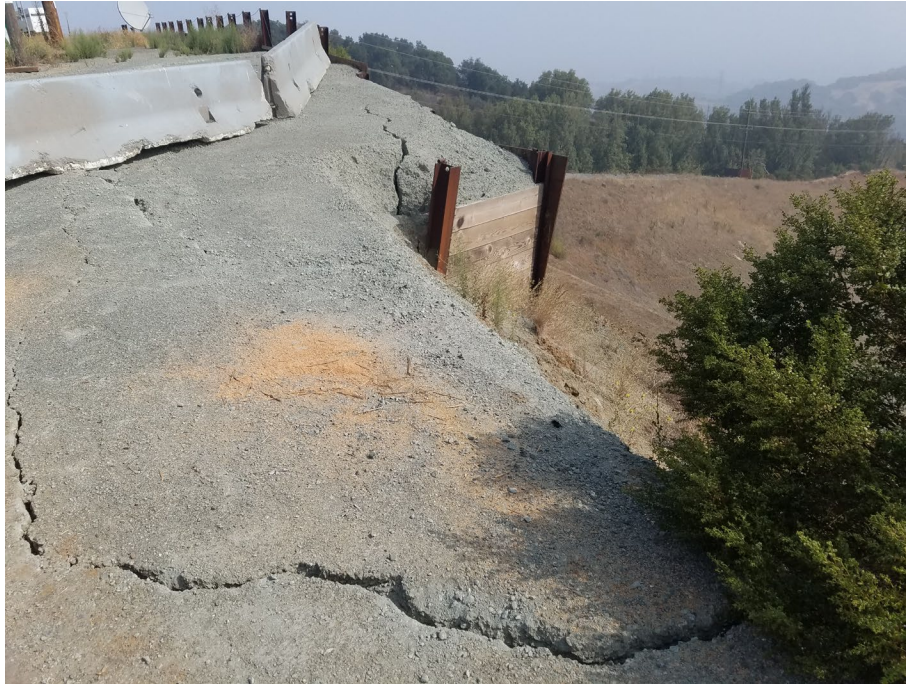
Photo 17: Ground cracks near northwest property line.
