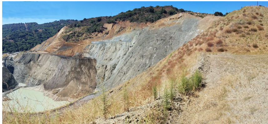
Photo 14: Buttress fill on north high wall. West side of pit visible on the left.
