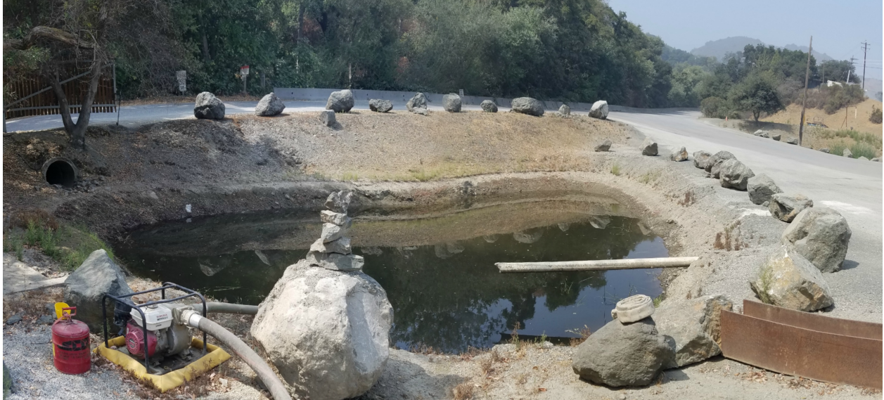
Photo 30: Settling basin near main entrance.
