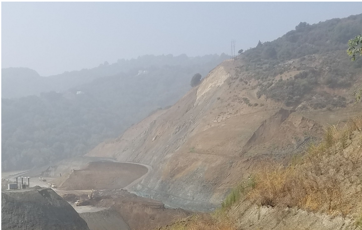
Photo 19: Slope failure on southwestern high cut wall, looking south. (Profile view)
