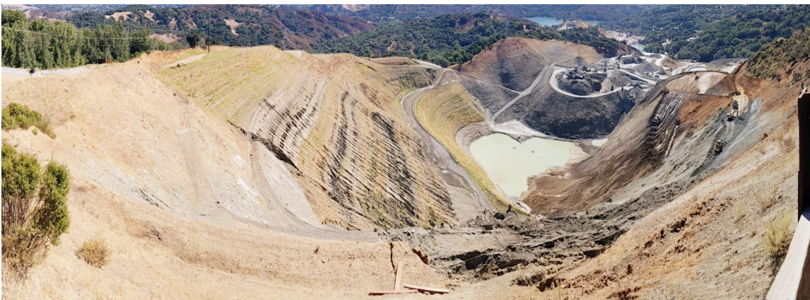
Photo 15: Panorama of buttress fill below retaining wall on northwest high wall.
