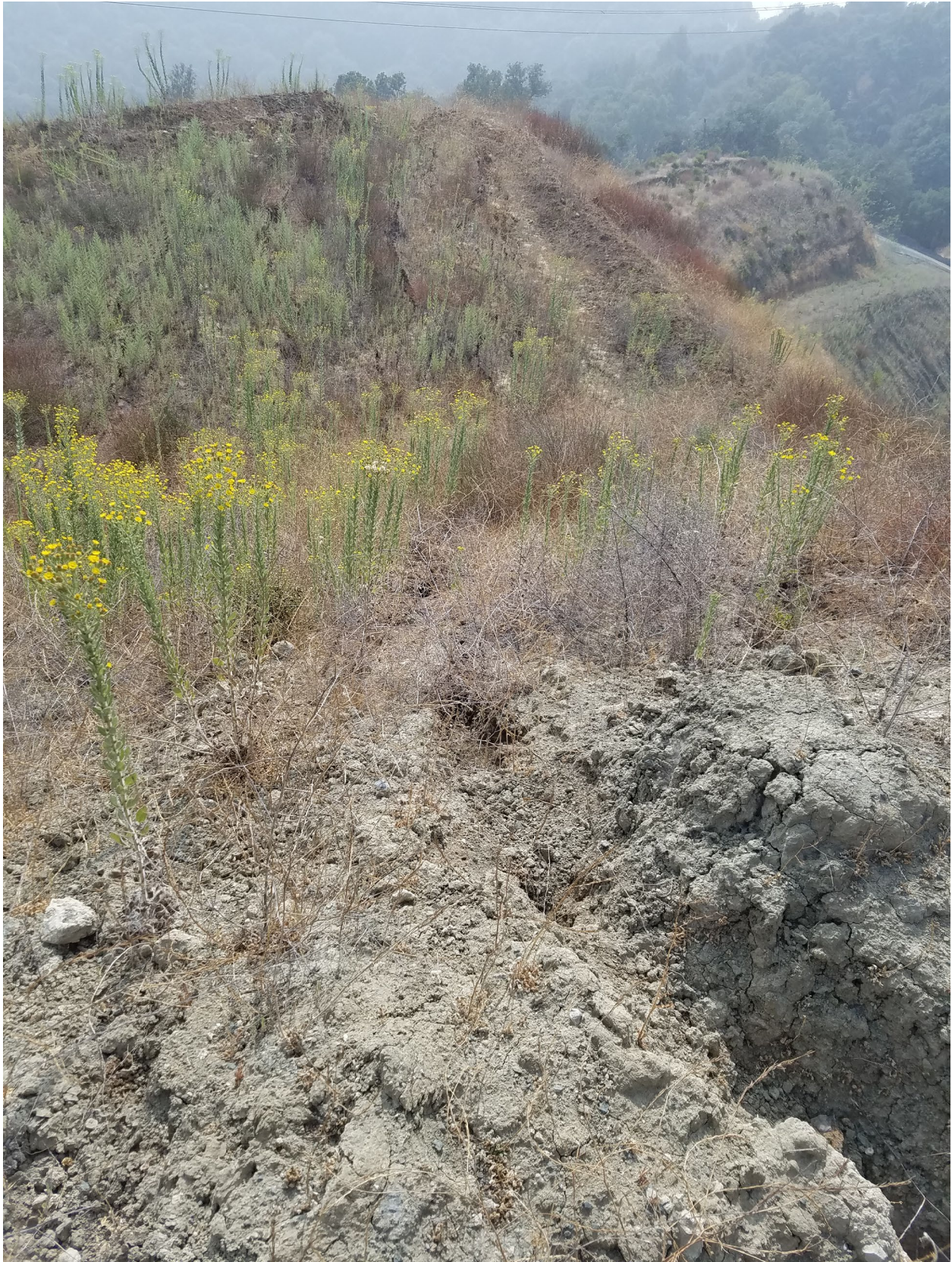
Photo 12: Ground crack on east-facing fill slope near northeastern corner of property.
