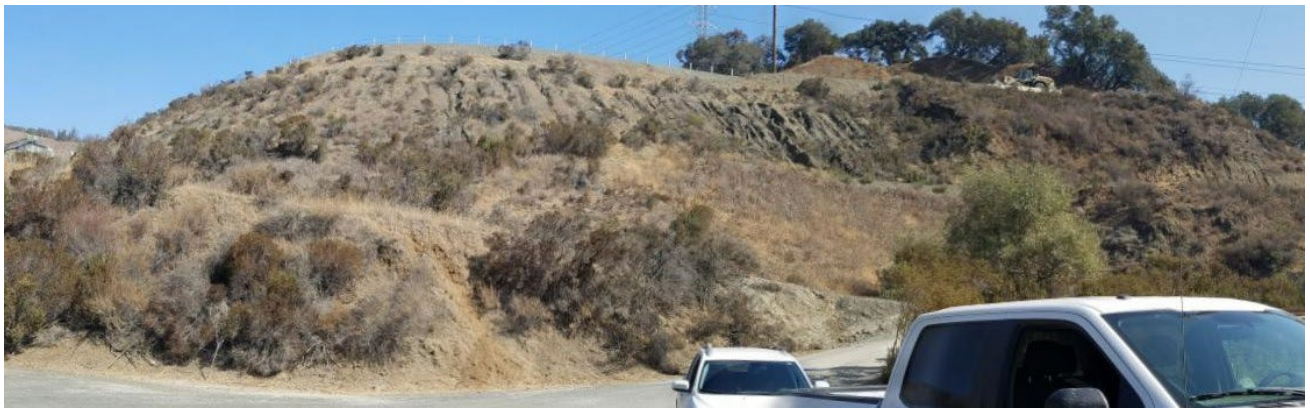
Photo 7: Erosion rills on fill slope above main haul road.
