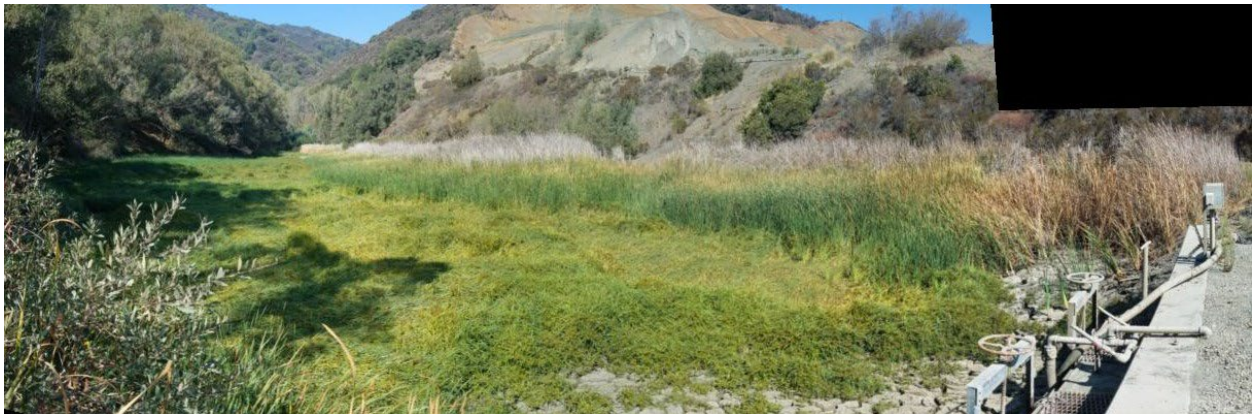
Photo 26: Upper Settling Basin.
