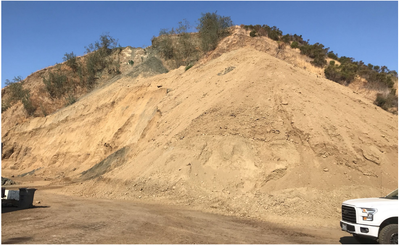
Photo 23: Dirt stockpile at eastern portion of Parcel A.
