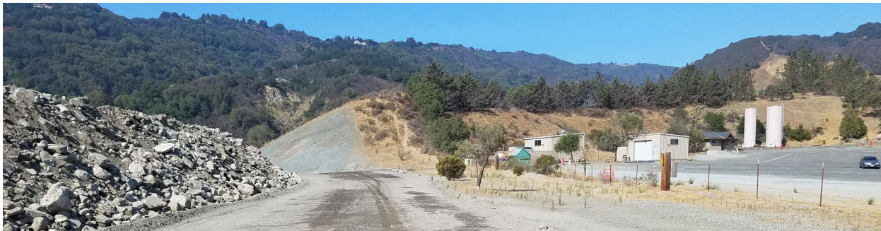
Photo 2: Repaired slope between Parcel A and gun club.
