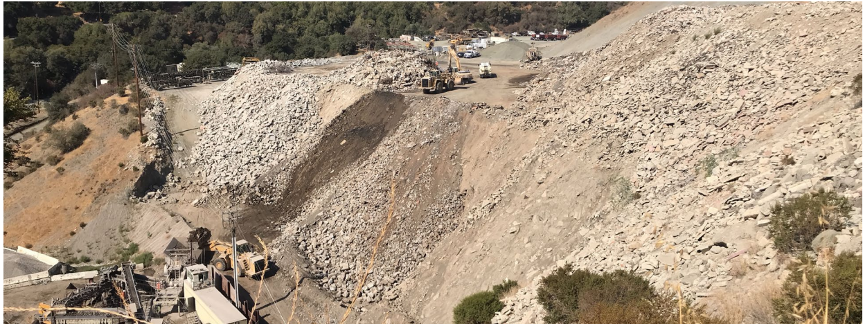
Photo 1: Recycling operation on Parcel A.
