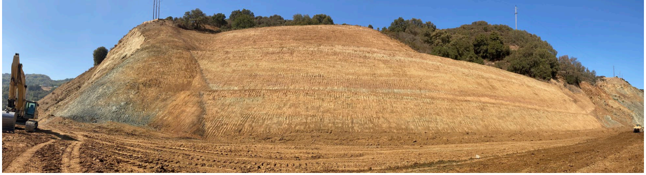
Photo 32: New cut slope along western part of property.
