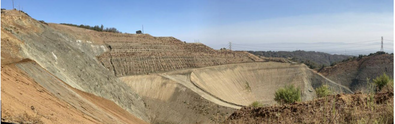
Photo 13: Buttress fill on north high wall.
