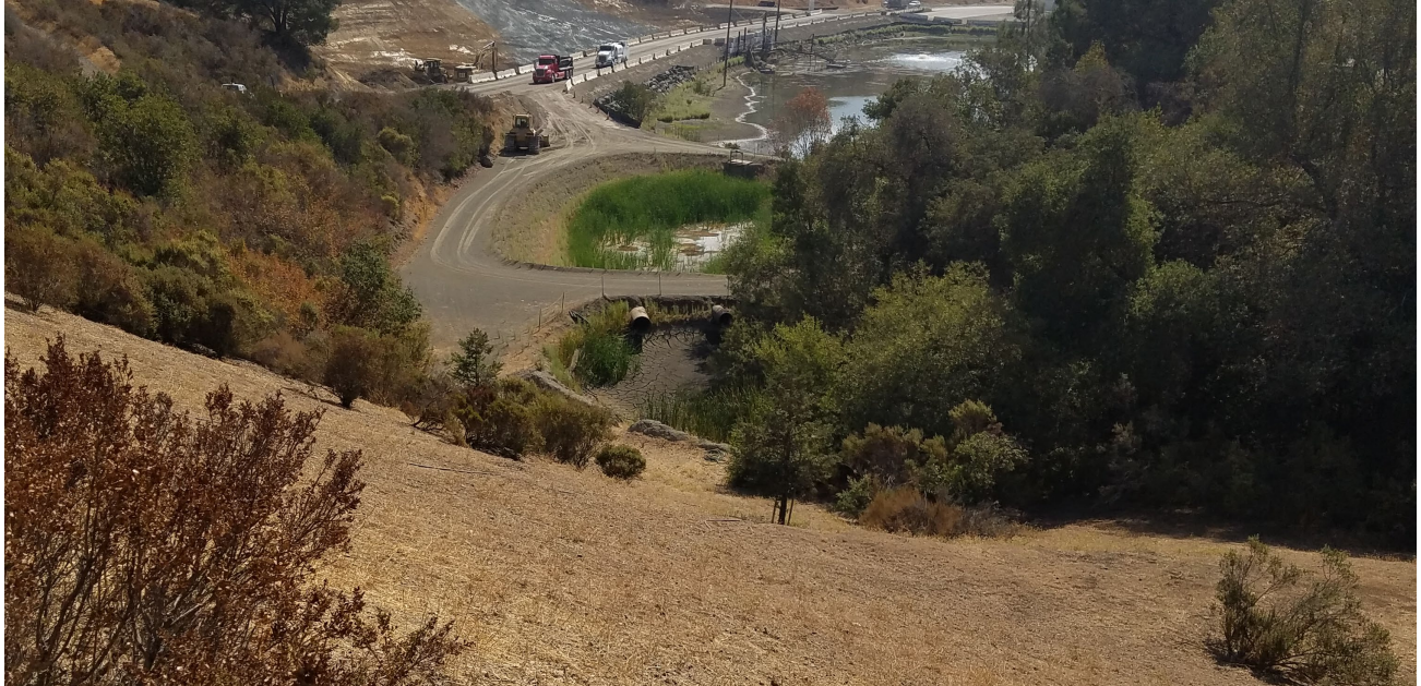
Photo 6: Face of dam between upper and middle settling basins.
