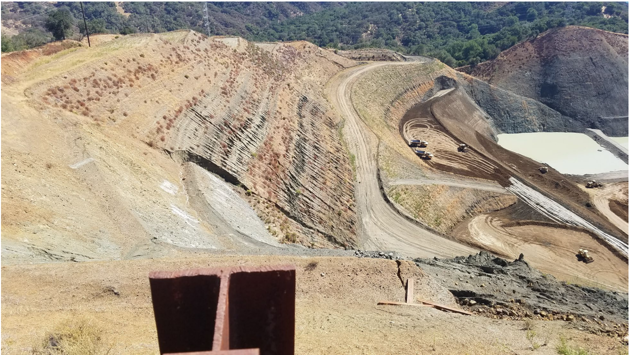
Photo 15: Panorama of buttress fill along north side of pit below retaining wall on northwest high wall.
