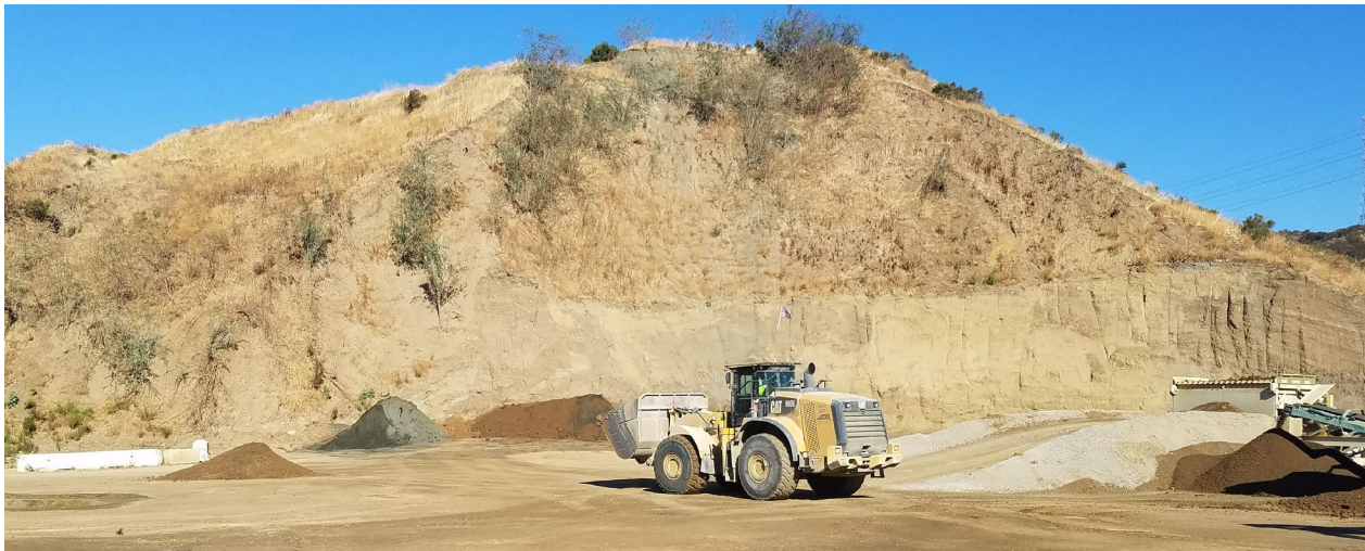
Photo 23: Dirt stockpile at eastern portion of Parcel A.
