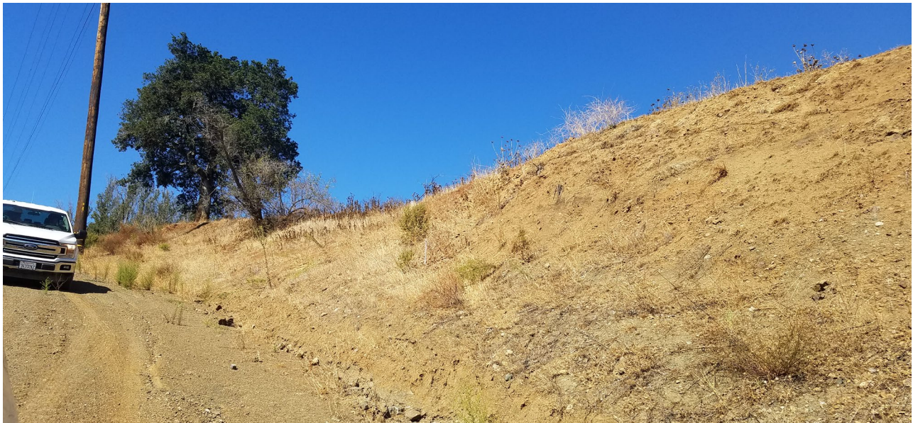
Photo 9: North perimeter road cut slope. No change in condition.
