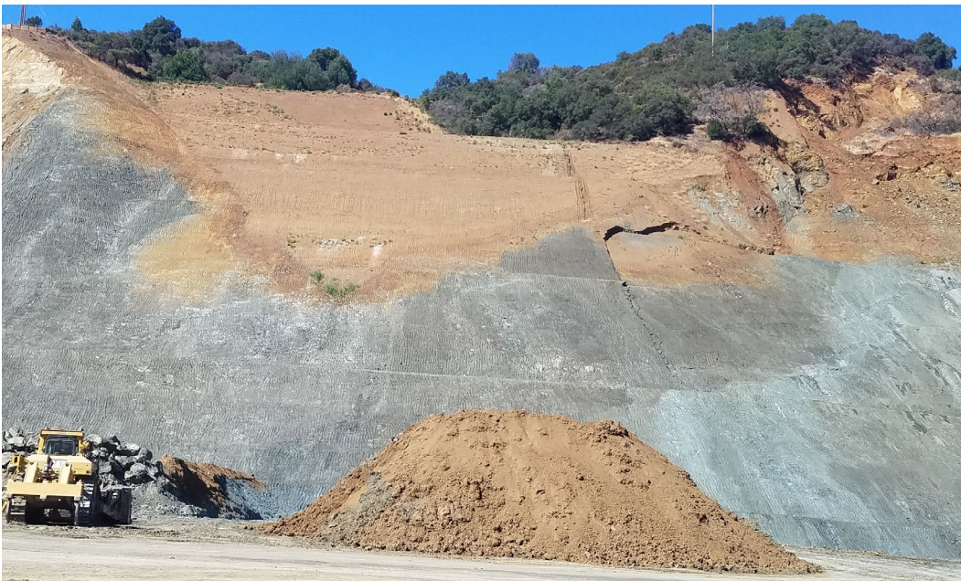
Photo 32: Final cut slope along western side of pit (center portion).
