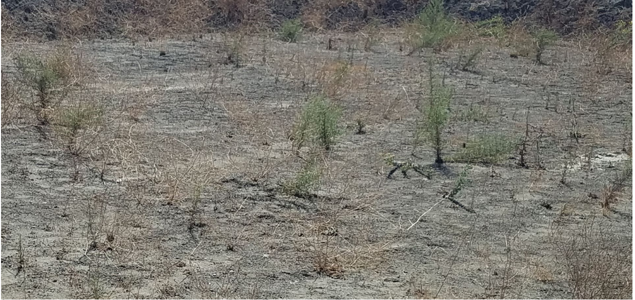
Photo 12: Location of former ground crack on east-facing fill slope near northeastern corner of property.
