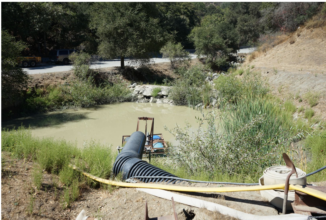
Photo 28: Drainage basin located west of office.
