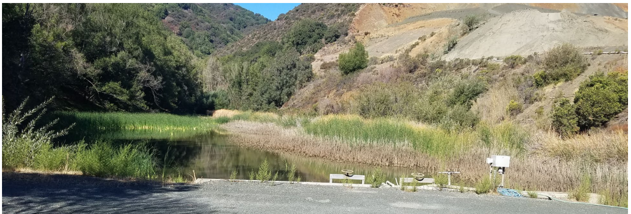
Photo 26: Former Upper Settling Basin; no longer receiving sediment from quarry operations.
