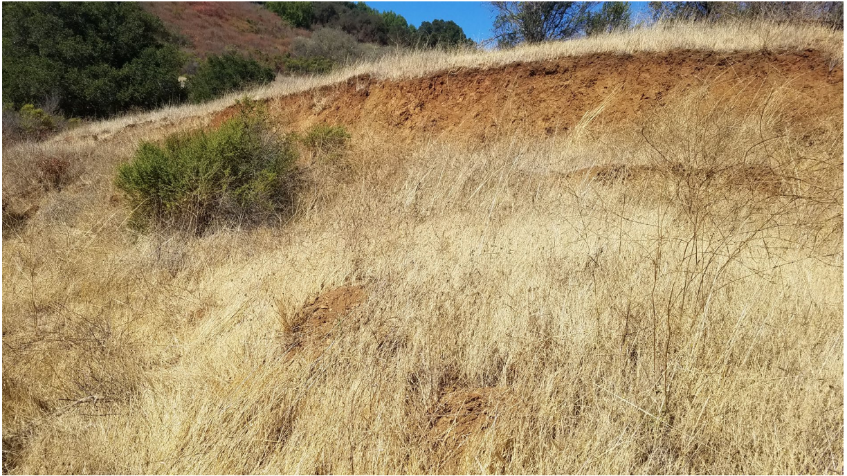
Photo 18: Ground cracks and headscarp beyond northwest property line.
