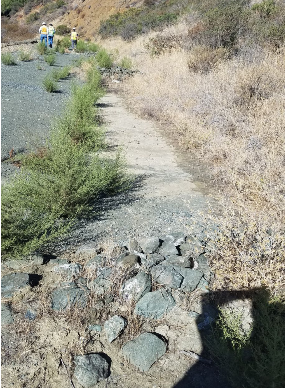
Photo 30: Check dams along road by north side of Rattlesnake Creek.
