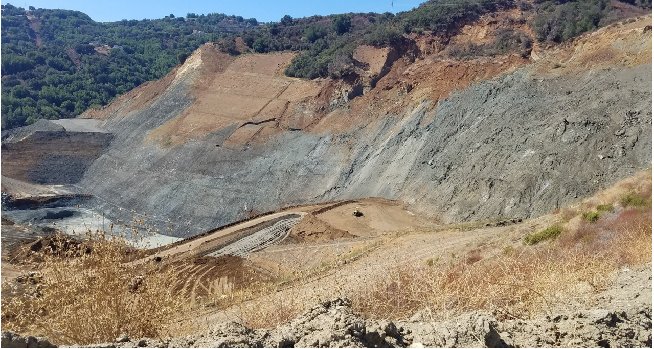
Photo 14: High wall along west side of pit.
