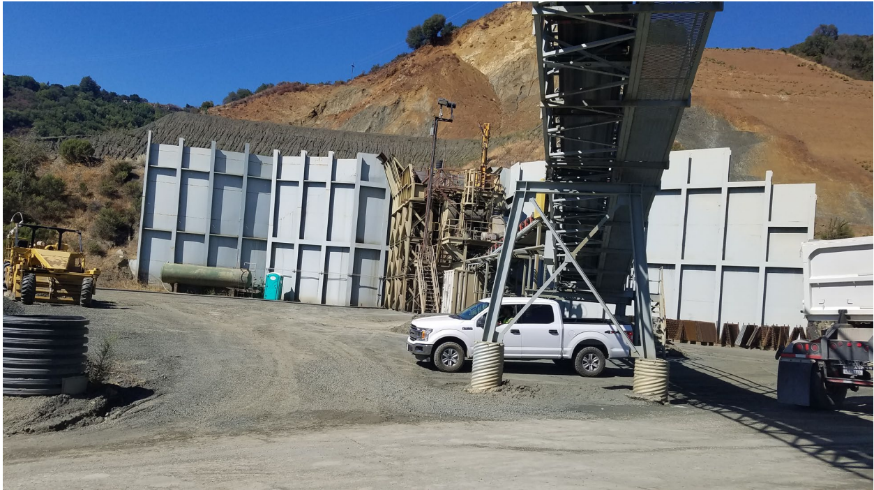
Photo 8: Relocated rock crusher.
