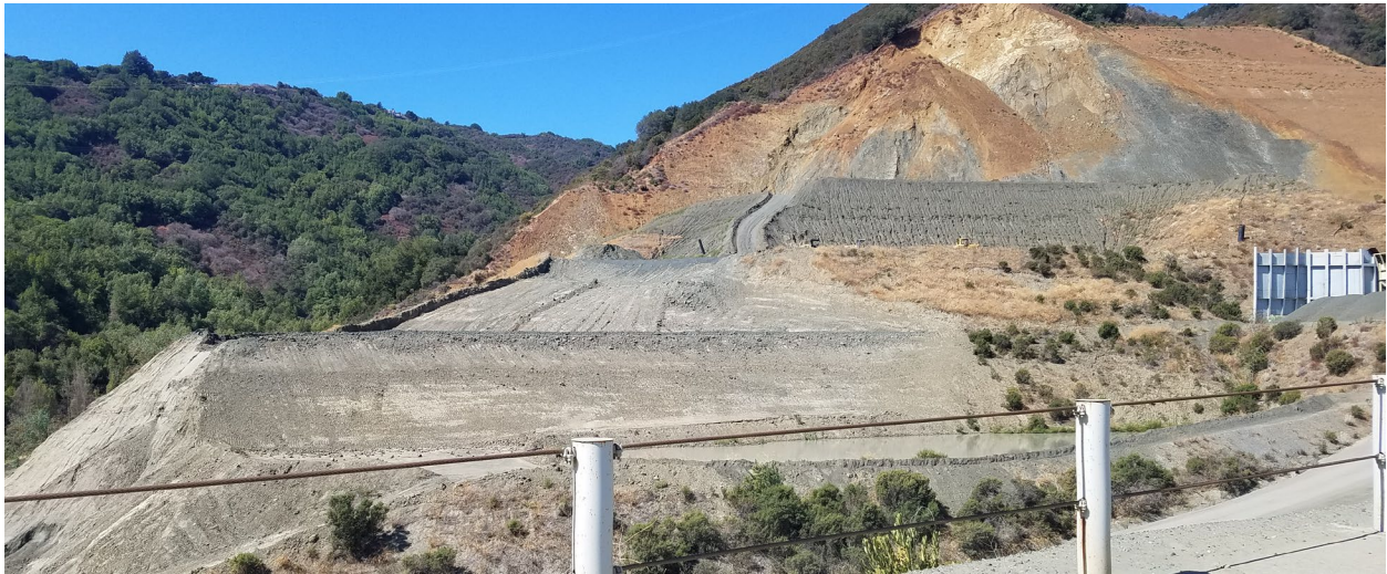
Photo 27: Regraded fill slope along west side of Pand 5..
