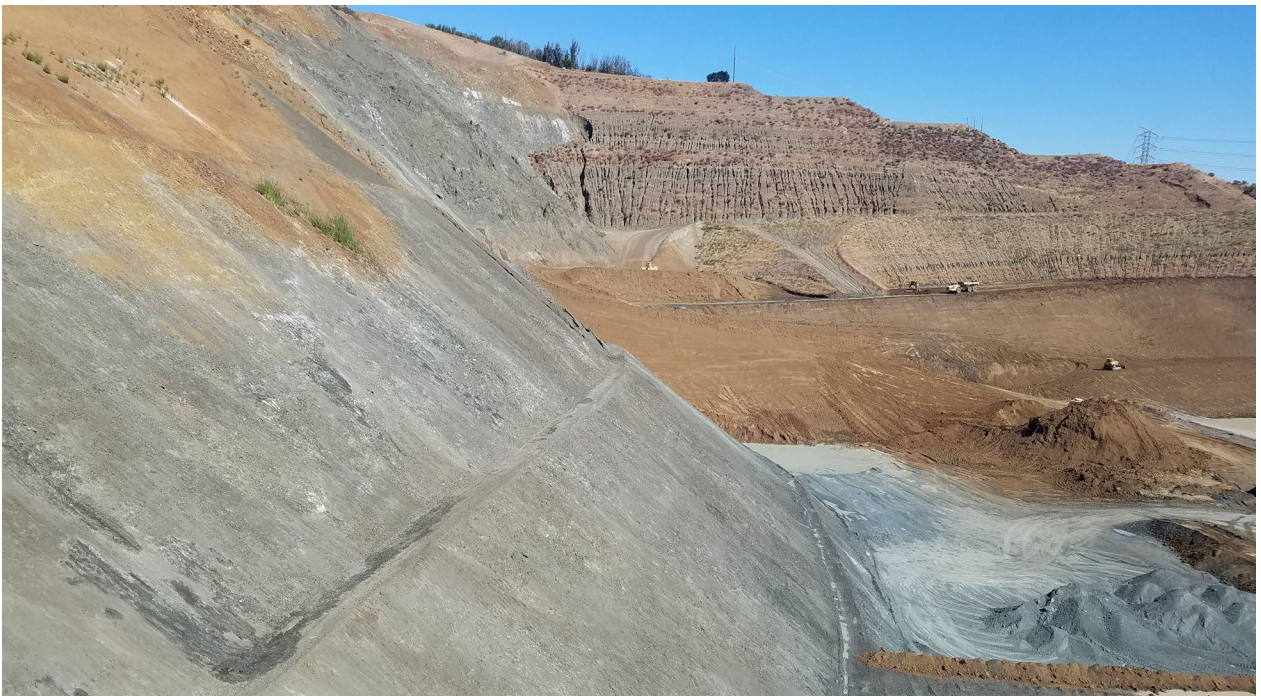
Photo 13: Buttress fill on north high wall.
