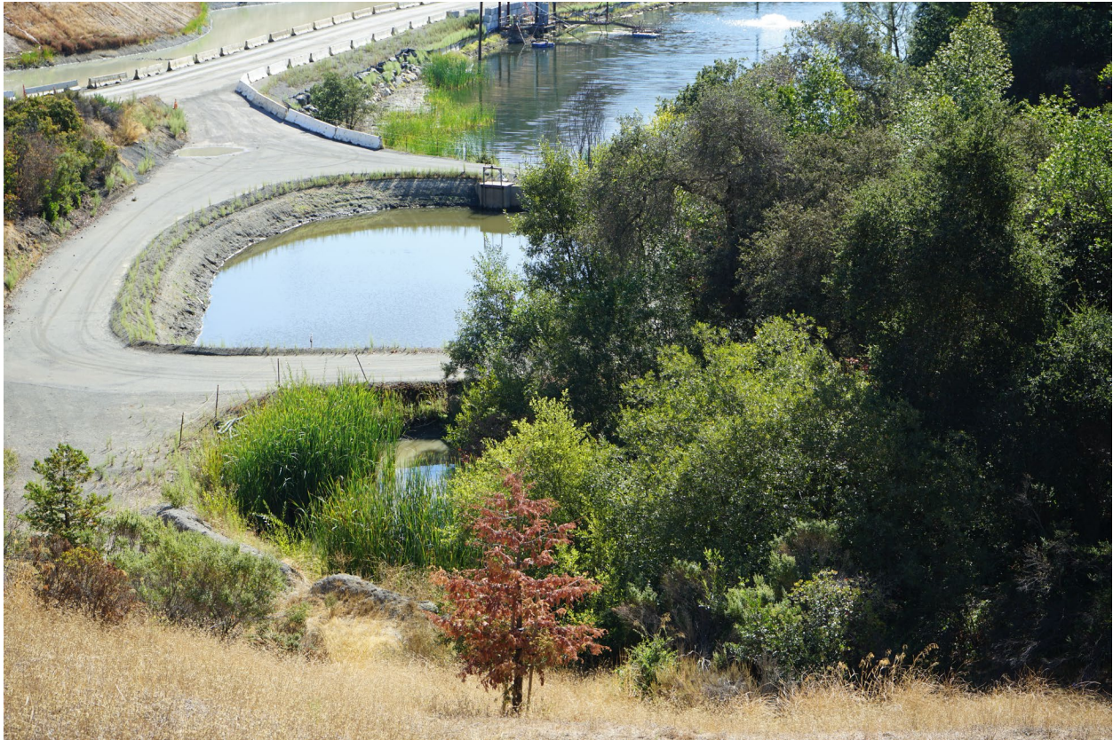
Photo 6: Face of dam between upper and middle settling basins.
