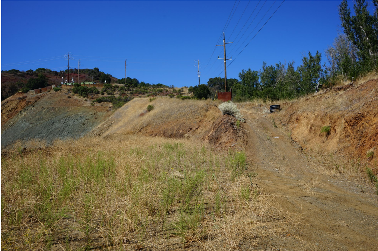
Photo 10: Area of former retaining wall above north high wall (buried)
