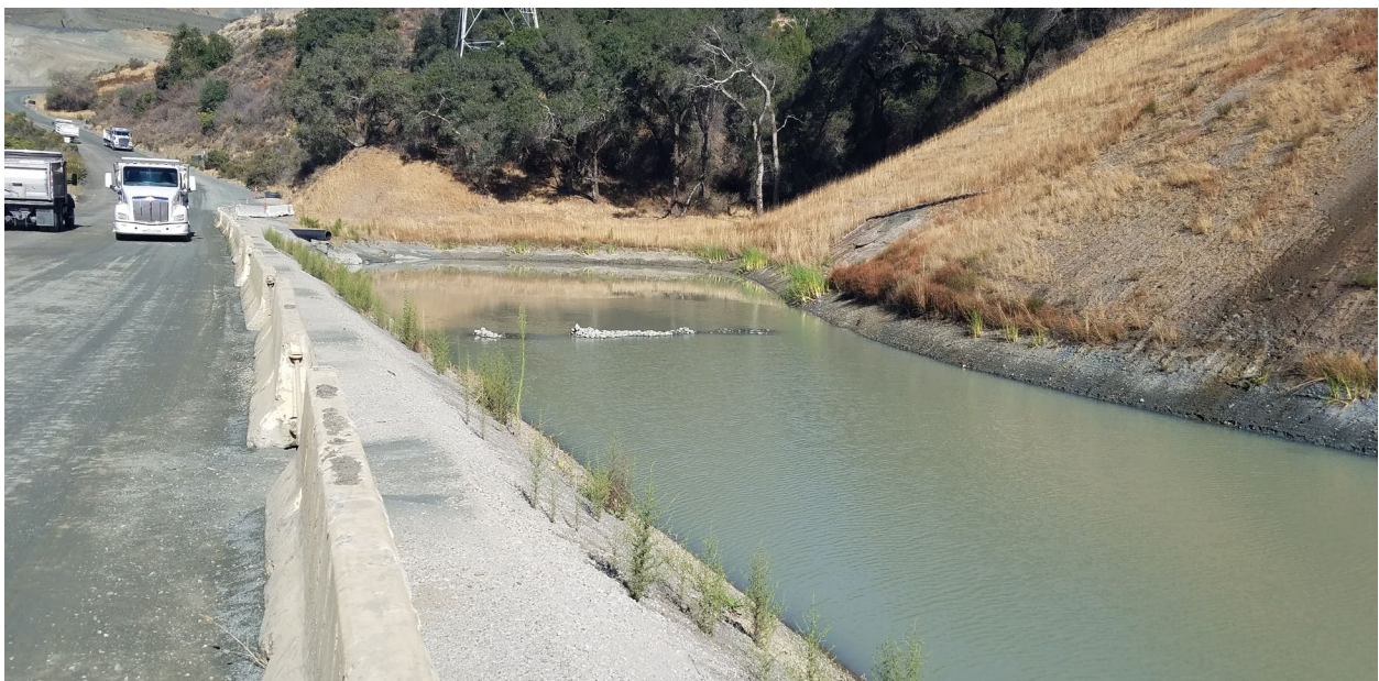
Photo 31a: West end of recently graded settling basin (known as BAGG basin) installed to comply with RWQCB requirements.
