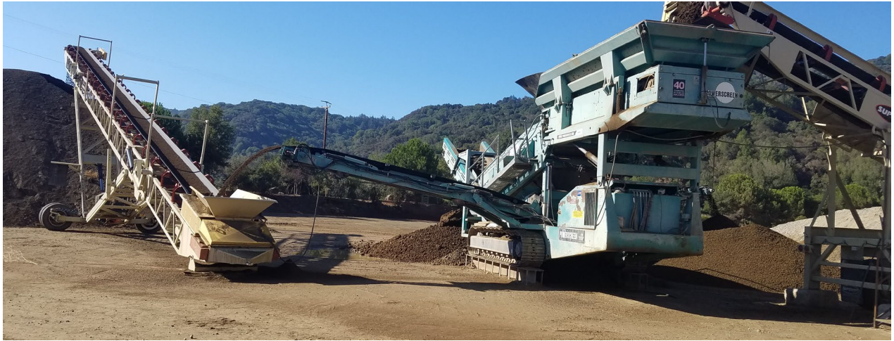
Photo 24: Soil processing equipment at eastern portion of Parcel A.
