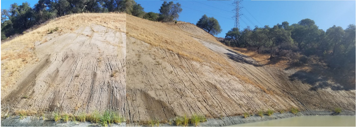
Photo 31b: Cut slope along north side of BAGG basin.
