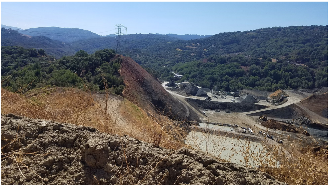
Photo 34: Looking south along cut slope on east side of pit.
