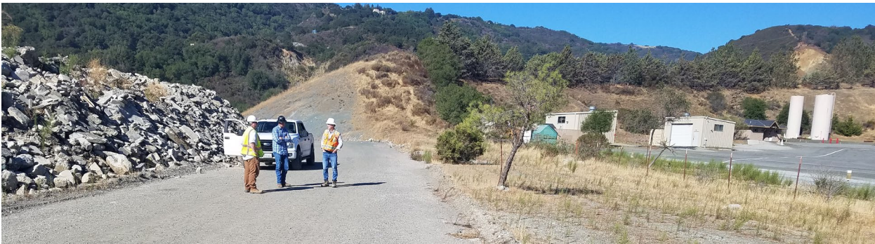
Photo 2: Repaired slope between Parcel A and gun club.
