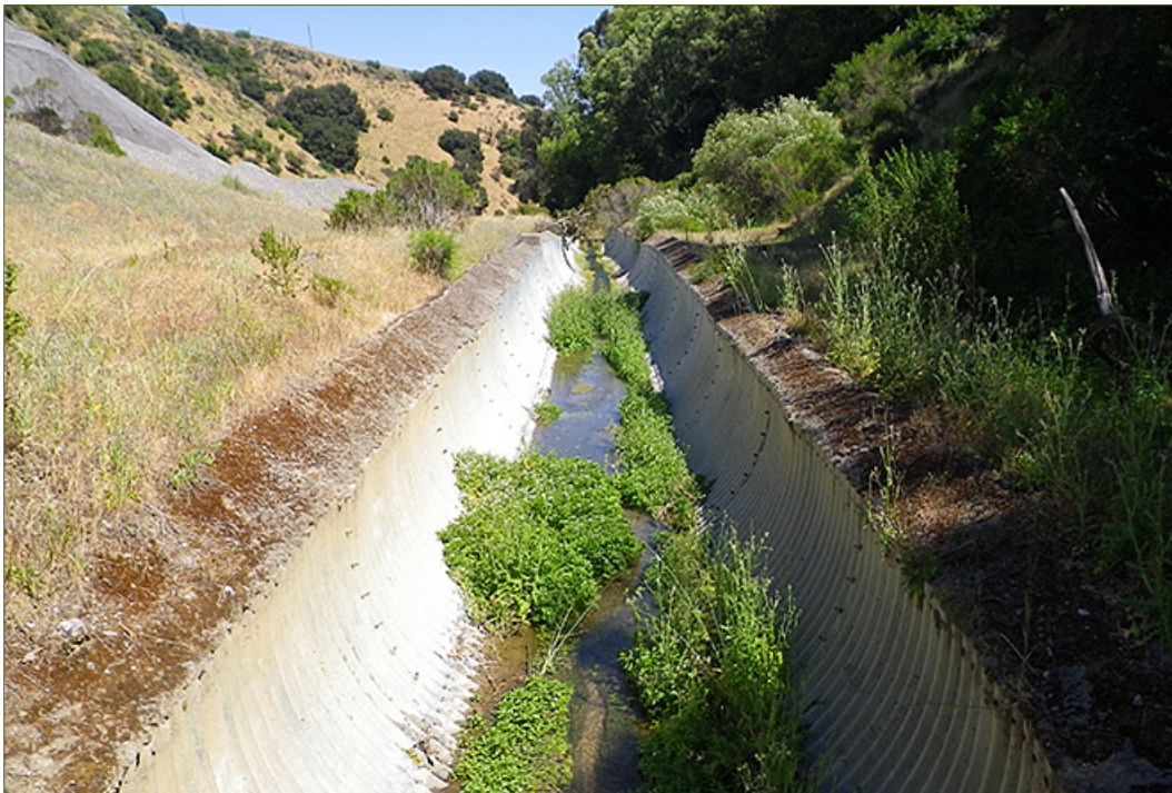
View of a channelized portion of Permanente Creek south of Pond 13.
