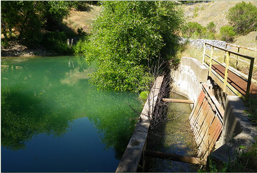
View of the downstream end of Pond 13.
