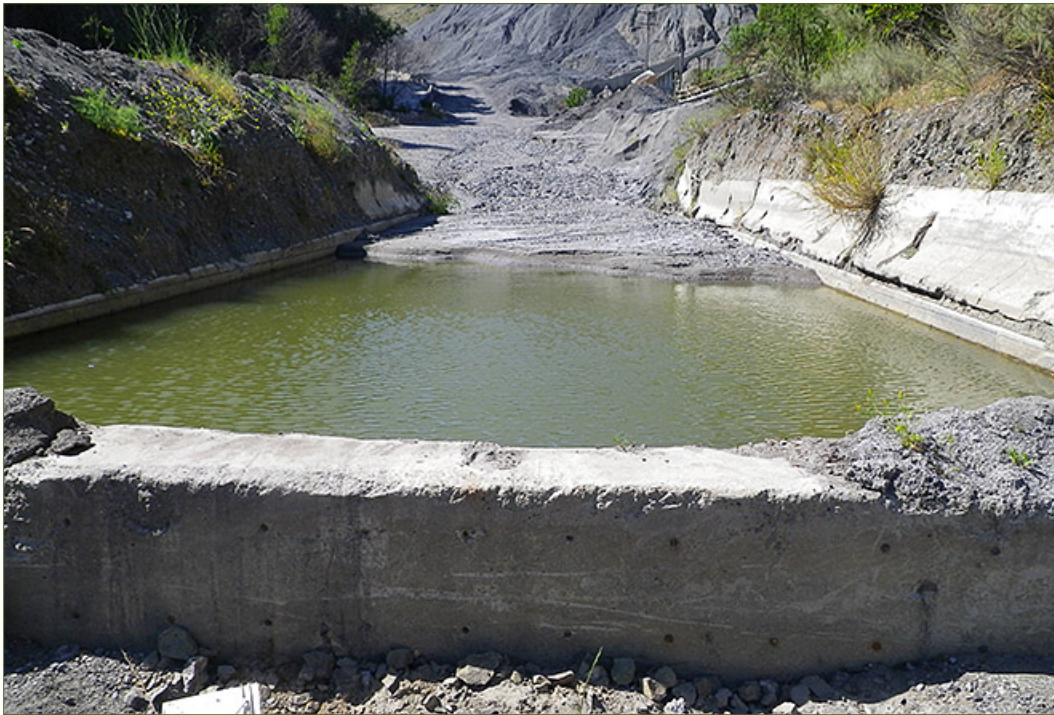
View of Rockpile Basin. Rockpile Basin is used as a settling basin for industrial purposes.
