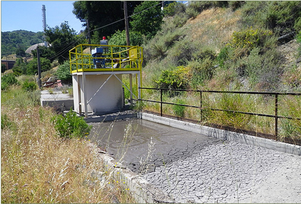
View of Pond 20. This feature is used as a settling basin for industrial purposes.
