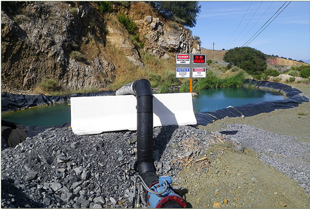
View of Pond 4A. Pond 4A is used as a water treatment basin for industrial purposes.
