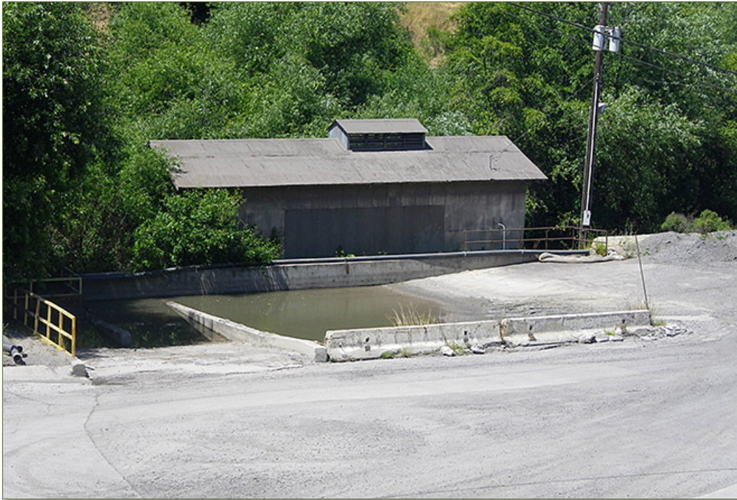
View of Dinky Shed Pond. This feature is used as a settling basin for industrial purposes.
