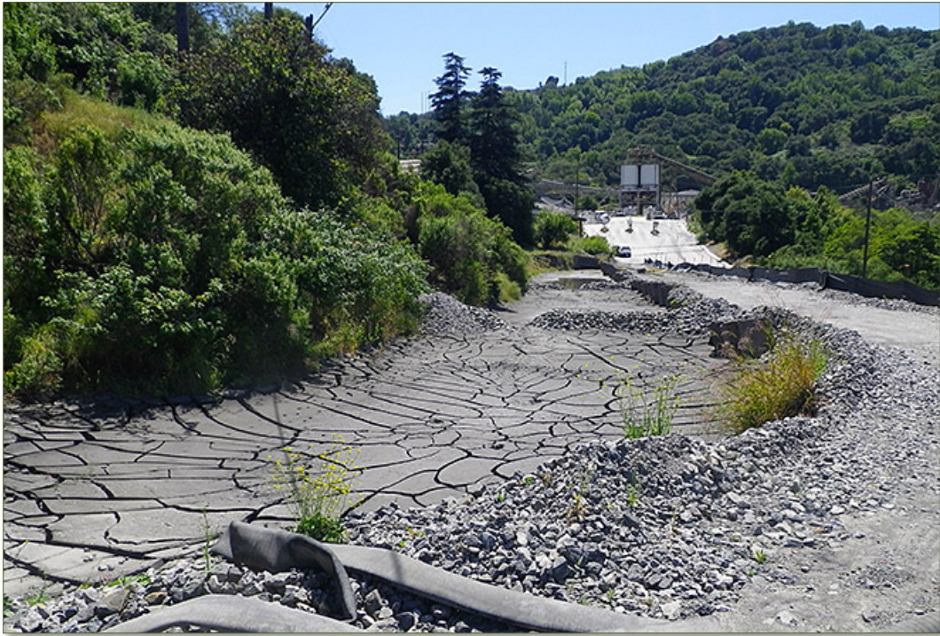
View of Pond 17. This feature is used as a settling basin for industrial purposes.
