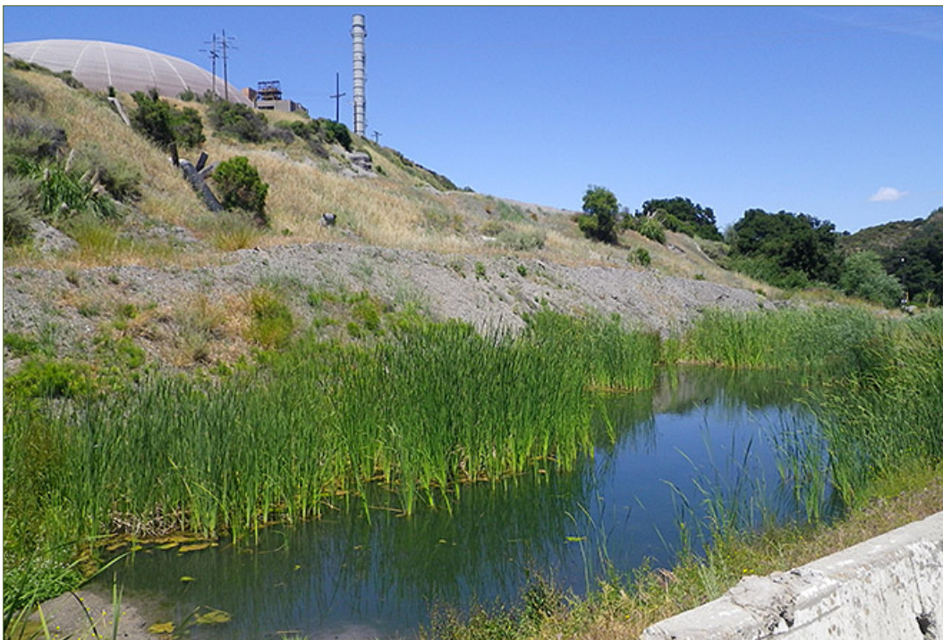
View of Pond 9. This feature is used as a settling basin for industrial purposes.
