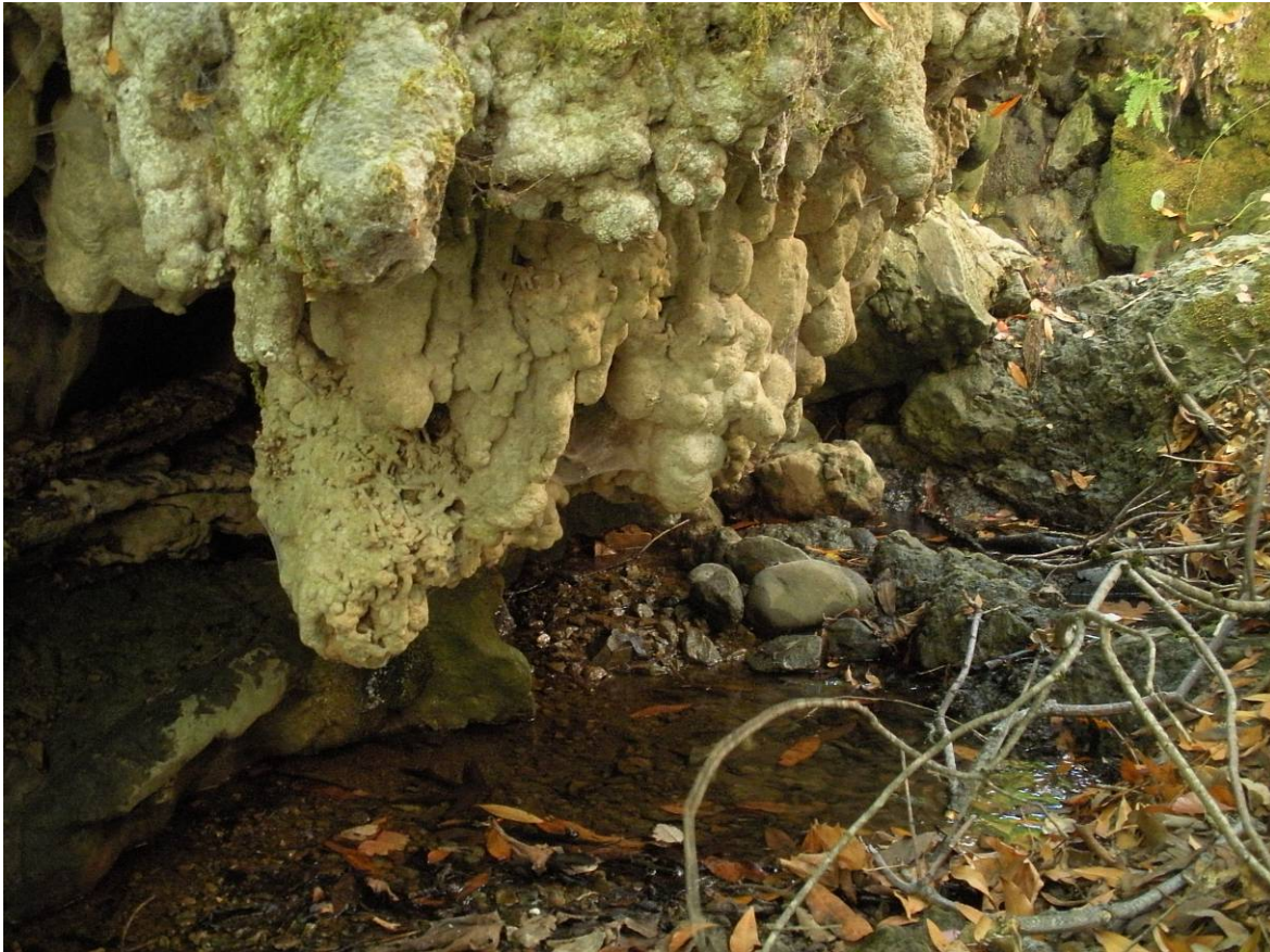
Figure 2-1 Calcium carbonate-encrusted roots and rock steps (right) within the ordinary high water elevation of the Creek
