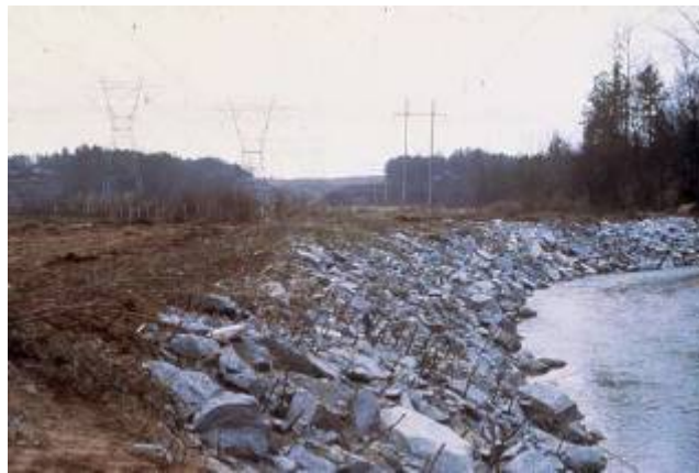
Figure E-11 Vegetated riprap installation
