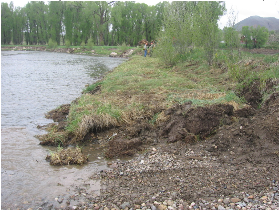
Figure E-2 Natural channel design installation with bankfull bench creation.
