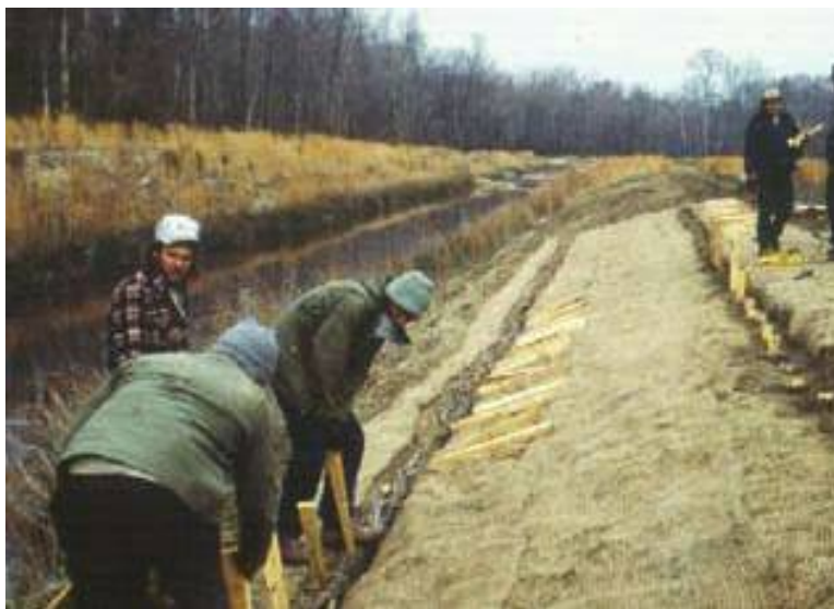
Figure E-9 Fascine installation.
