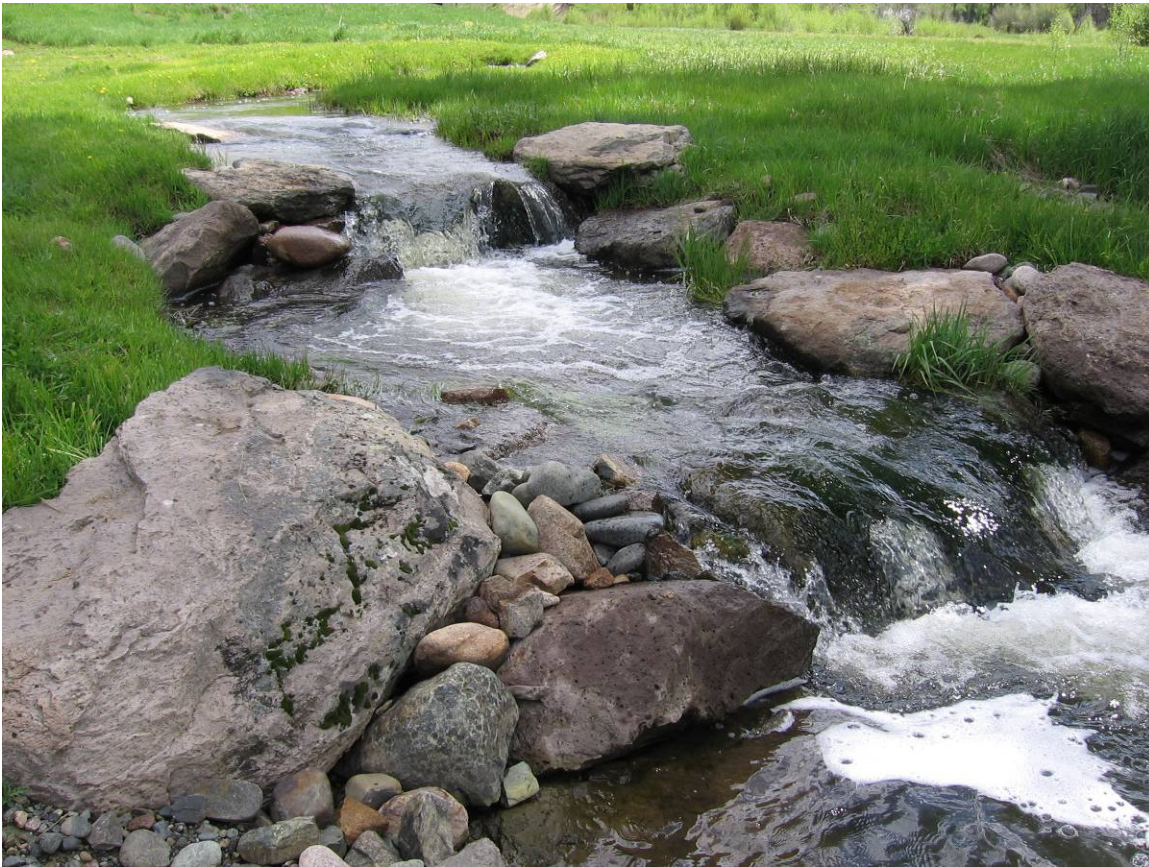
Figure E-4 Step-pool installation.
