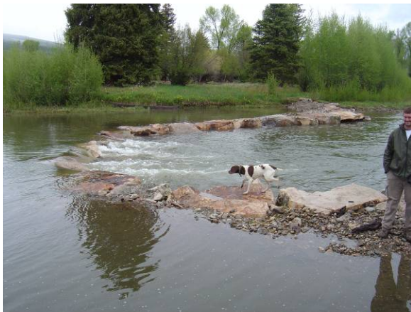
Figure E-3.1 Rock cross vane installation.
