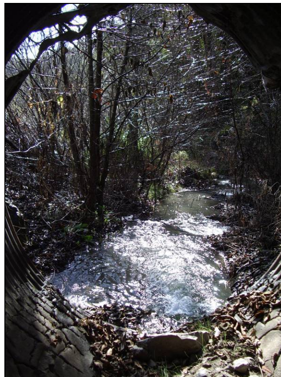
Figure 2-19 Looking downstream at Reach [9] from within the dry parallel culvert near Station 74+00
