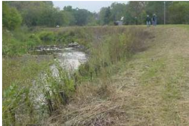
Figure E-10 Live stake installation after one growing season.
