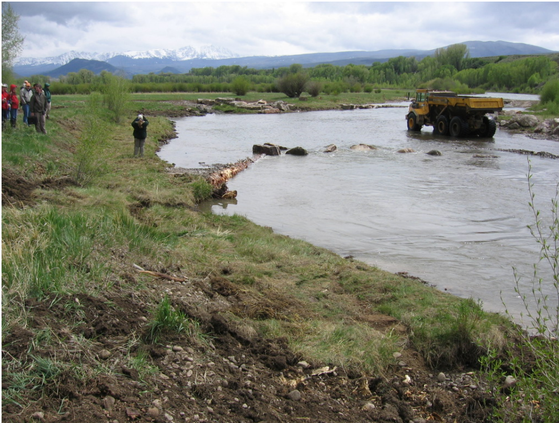
Figure E-5 Installation of a log/rock J-hook vane.
