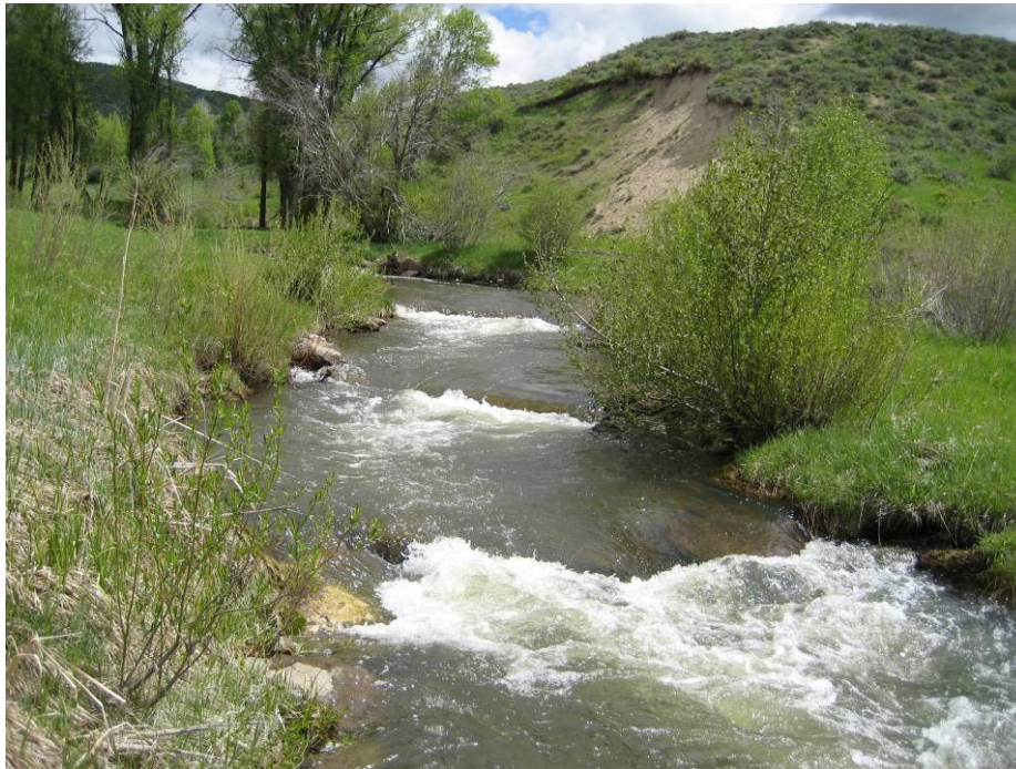
Figure E-1 Natural channel design installation with channel realignment.
