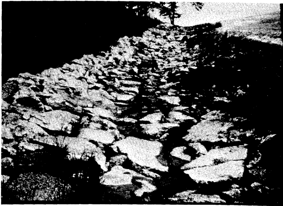
Figure 8. Broken concrete riprap.
