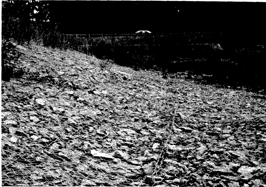
Figure 9. Rock and wire mattress revetment.
