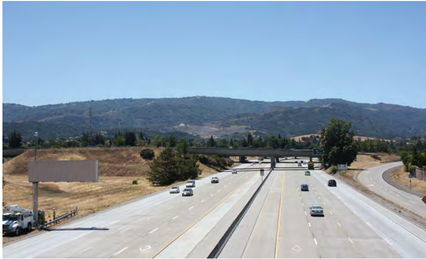
Photo 1: Mary Avenue Bicycle Footbridge looking southwest over Interstate-280
