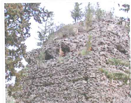
Opus caementicium lying bare on a tomb near Rome. In contrast to modern concrete structures, the concrete walls of Roman buildings were covered, usually with brick or stone.
