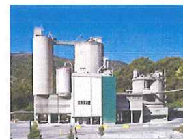
Lafarge cement plant in Contes, France.
