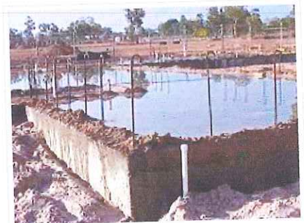
A concrete slab ponded while curing.
