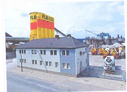
Concrete plant facility (background) with concrete delivery trucks.
