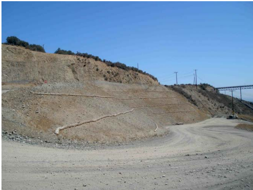
Photo 22: Slopes on roadway to new crusher area. Slope straw waddled and hydroseeded before last winter. Dated September 4, 2014.
