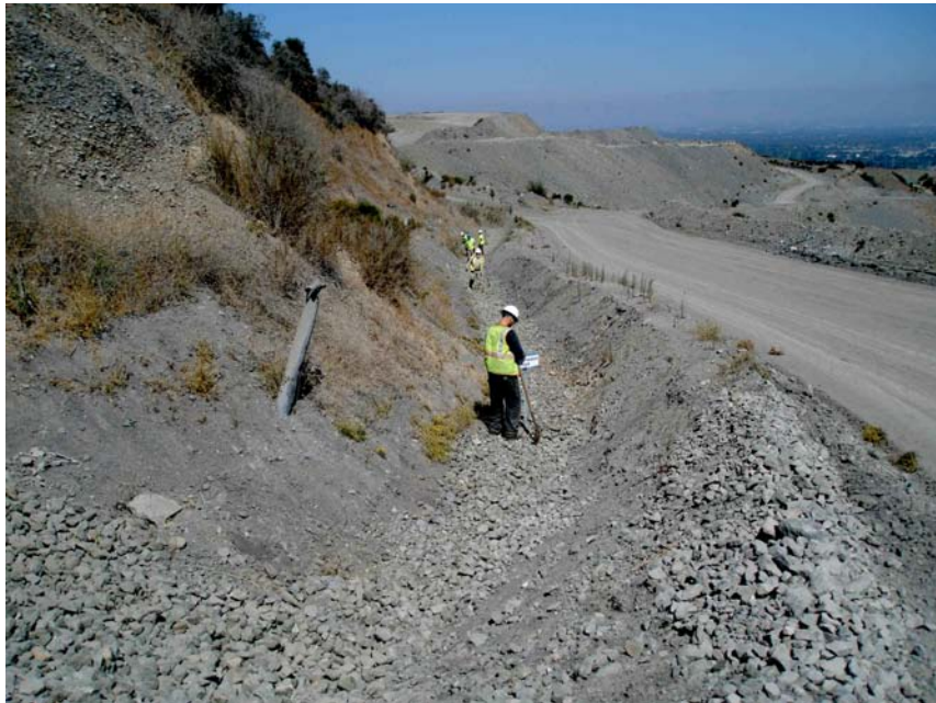
Photo 14: Western perimeter drainage ditch in EMSA. Ditch being cleaned out and greenstone rock lining bottom, looking northeast. Dated September 4, 2014
