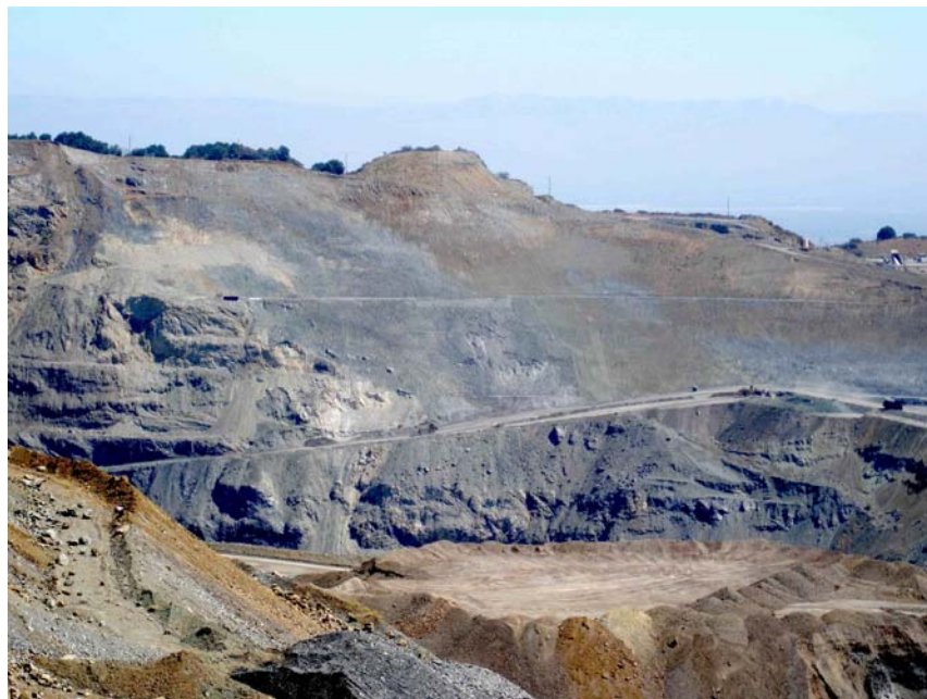
Photo 2: Upper portion of eastern highwall of North Quarry with slopes at final grade. Dated September 4, 2014.
