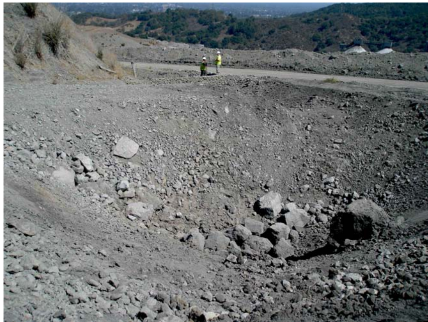
Photo 16: Second sediment catch basins constructed above western perimeter drainage ditch in background. Dated September 4, 2014.
