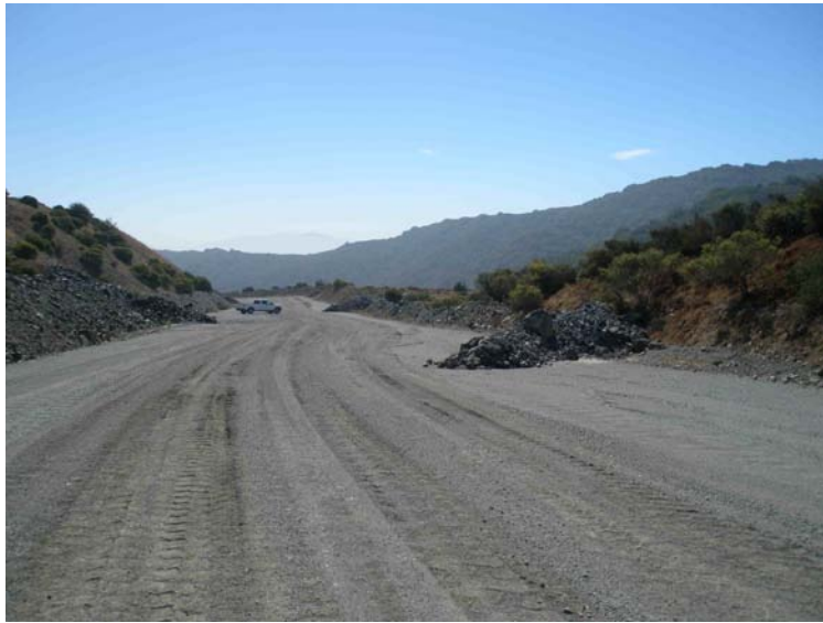
Photo 3: Check dams on WMSA haul road that were replaced with non-limestone materials, looking eastward. Dated September 4, 2014.
