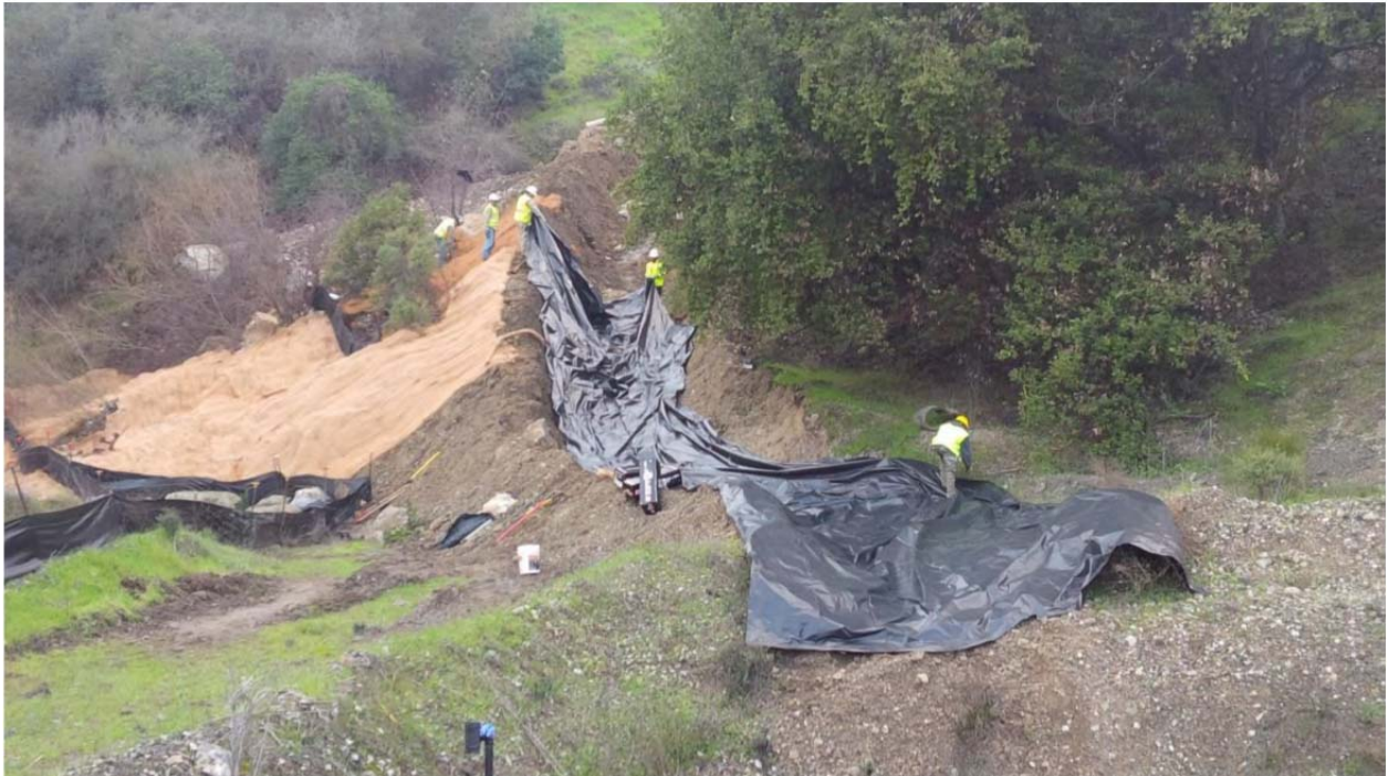
Installed drainage ditch and liner to redirect future storm flows
