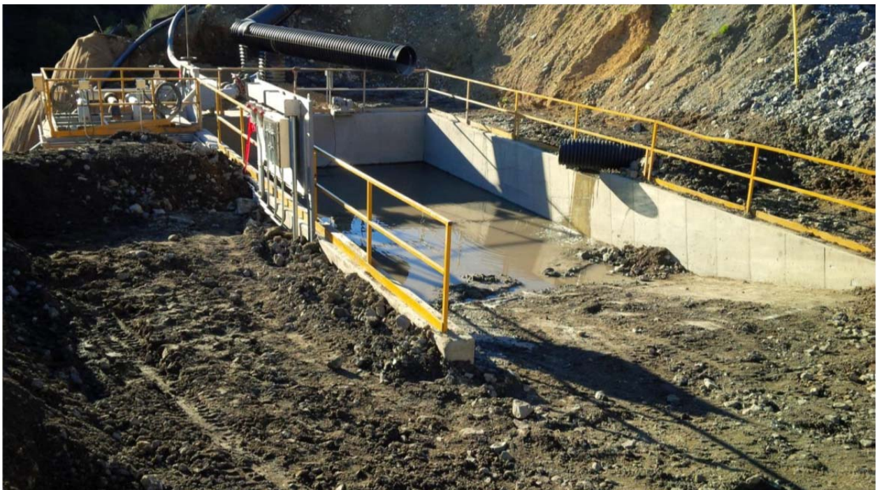
Regraded upper sump area and prepared for shotcrete application
