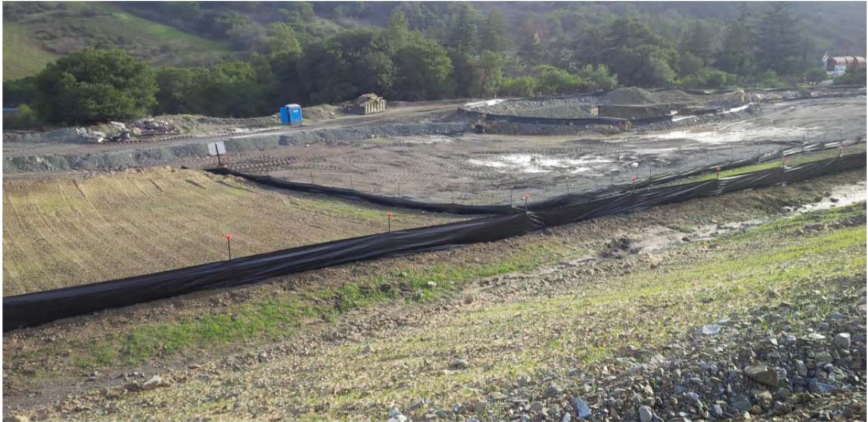
Installed berms and silt fencing in lower area
