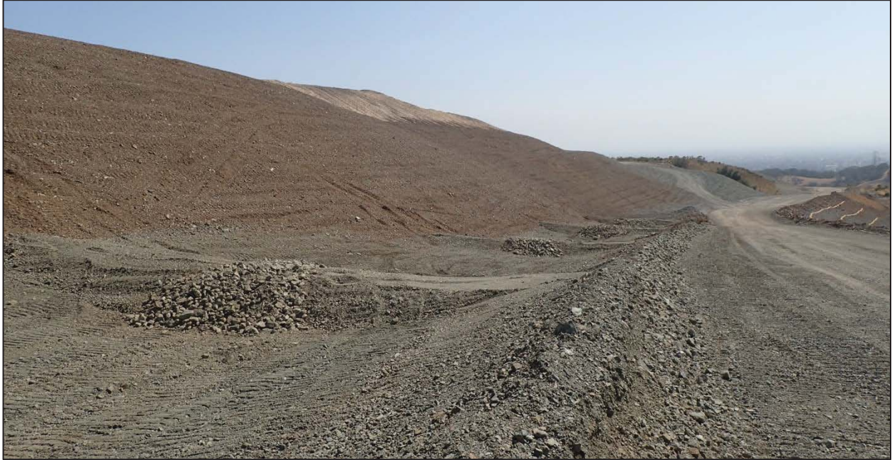
Photograph 5. New non-limestone lined stormwater conveyance ditch with checkdams along EMSA haul road. Bare soil shown in photograph will be hydroseeded in October 2015.
