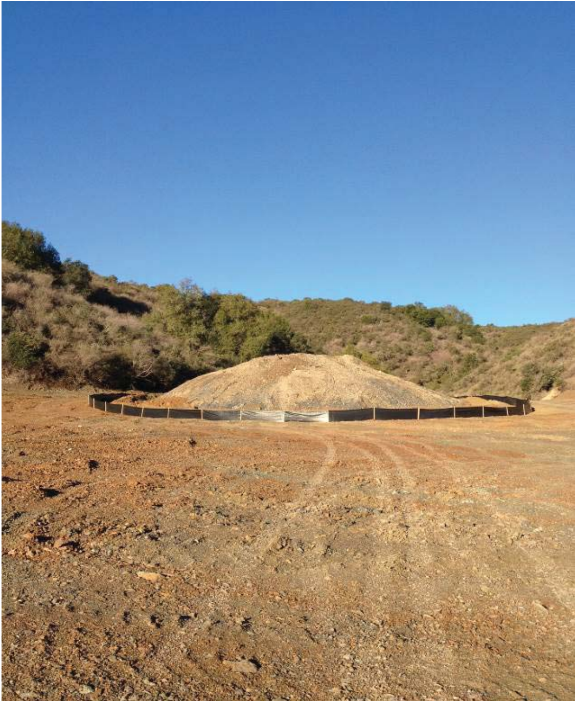
Photo 5: EMSA topsoil stockpile with silt fence BMP installed.
