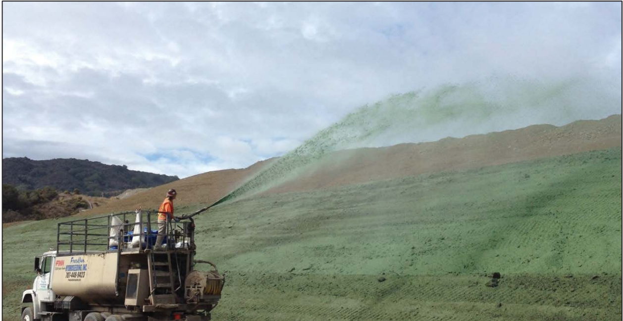
Photograph 7. Hydroseed application of hillside on interim reclaimed slopes in the lower EMSA near Pond 30.
