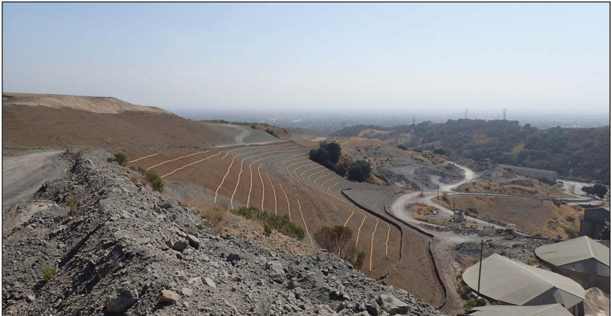
Photograph 6. Erosion control straw wattles and silt fences installed on interim reclaimed slopes in the EMSA. Bare soil shown in photograph will be hydroseeded in October 2015.
