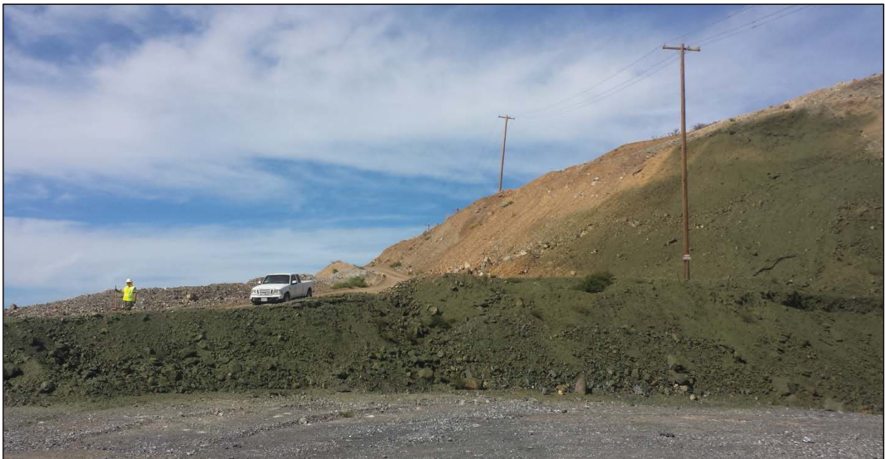
Photograph 4. Newly reclaimed slope above north wall in North Quarry Area hydroseeded with erosion control seed mix.
