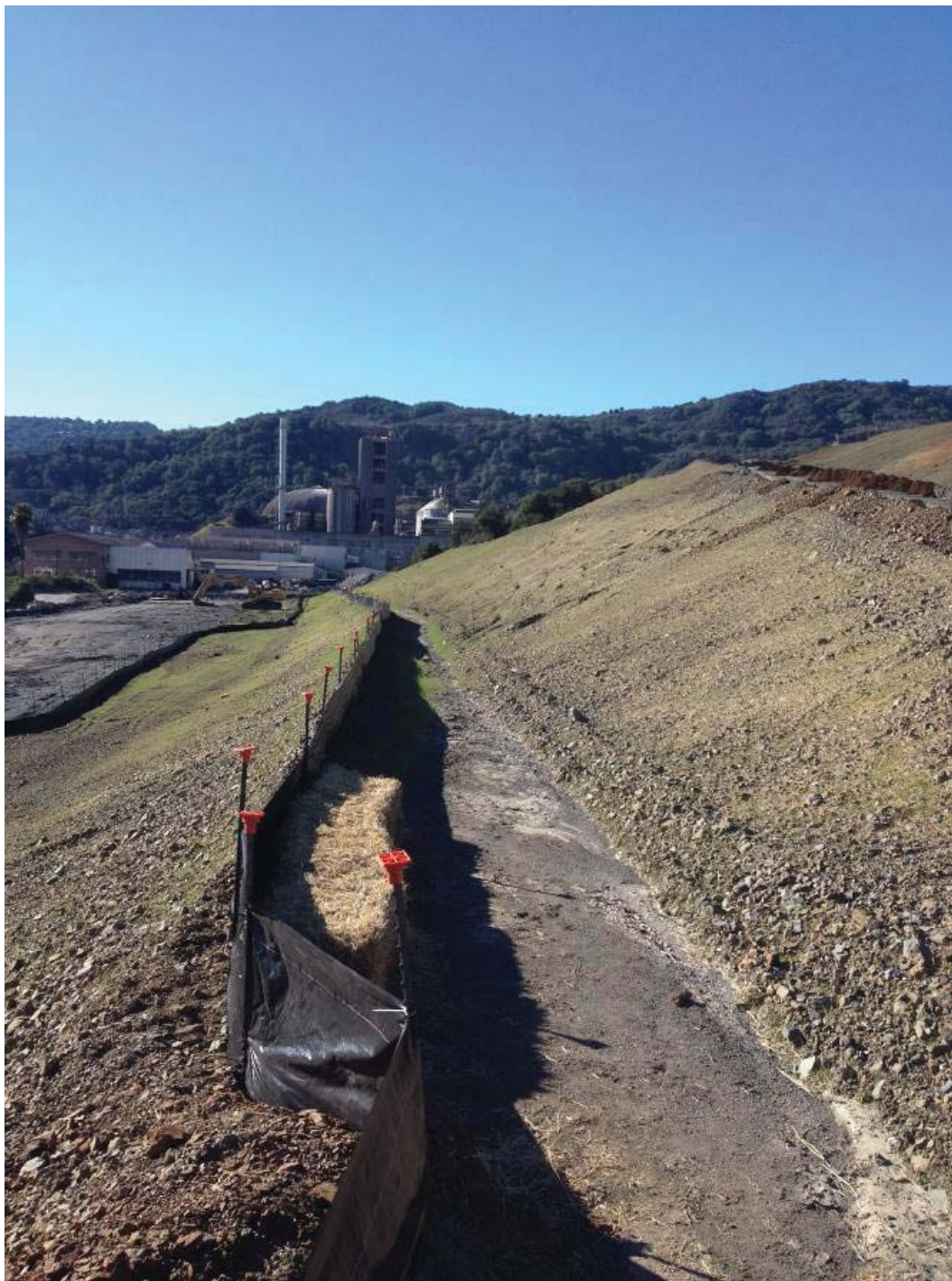
Photo 3: Stormwater containment ditch from EMSA haul road hairpin turn to Pond 31B with installed silt fence BMP.
