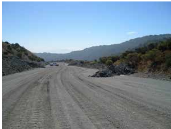
Check dams installed on haul roads, greenstone rock materials (photo taken Sept. 2015).
