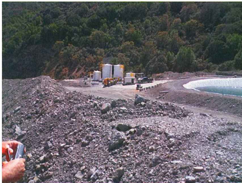
Photo 36: Holding tanks and new lined pond south of North Quarry that discharge to the interim treatment plant shown in Photos 33 and 34. Dated September 3, 2015.
