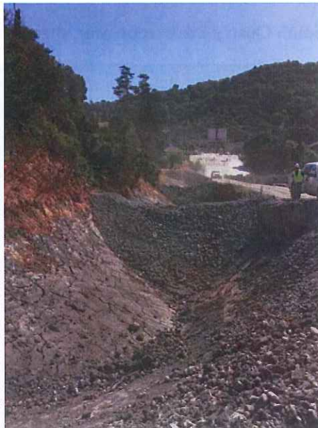
Photo 30: Pond 17 looking south at Rock Plant. Rock Plant was not in operation at the time of the 2015 inspection. Dated September 3, 2015.
