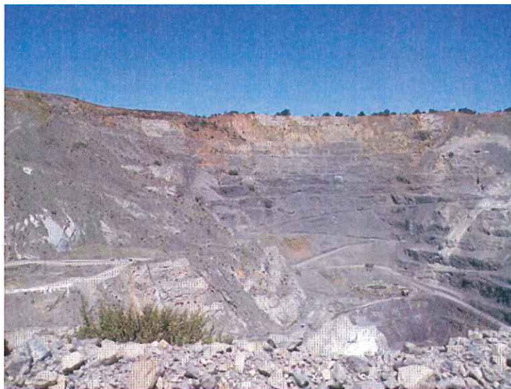
Photo 4: Looking north at the North Quarry. Main Rockslide on left, Scenic Easement Rockslide in center and remnants of Mid-Pen Rockslide on right. Compare to Photos 4, 5 and 6 in 2014 inspection report. Dated September 3, 2015.
