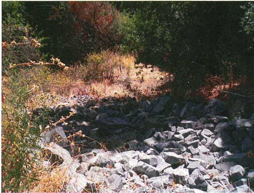
Photo 19: Pond 30 rocked outfall to Permanente Creek. Dated September 3, 2015.
