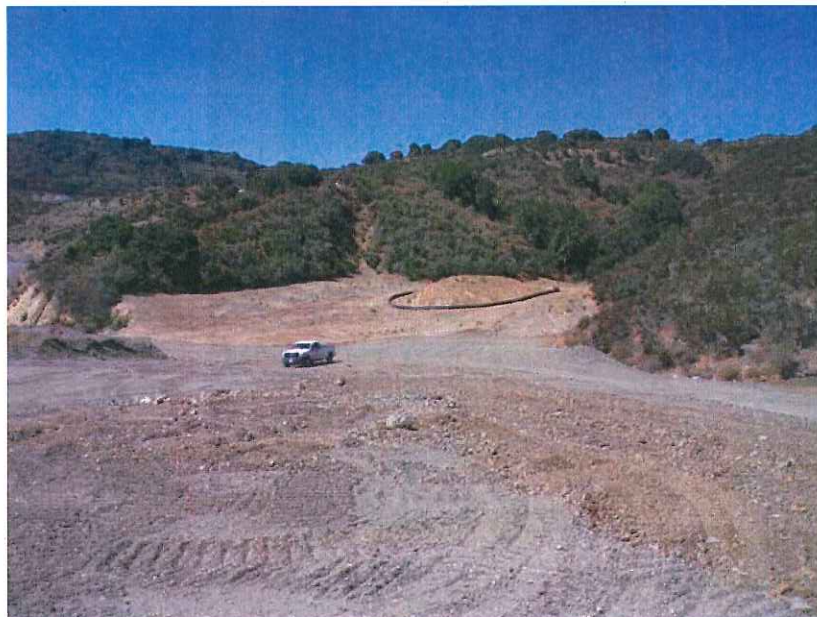
Photo 32: Topsoil stockpile in EMSA surrounded by silt fencing. Dated September 3, 2015.
