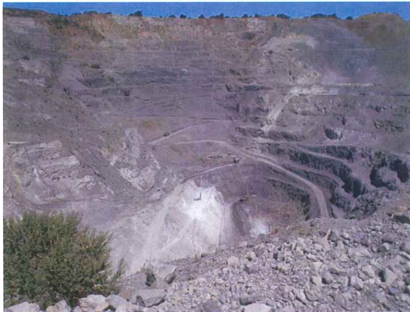
Photo 1: North Quarry, looking north. Waste rock material being placed at toe of western slope. Floor elevation of quarry at approximately 625 feet msl. Dated September 3, 2015.
