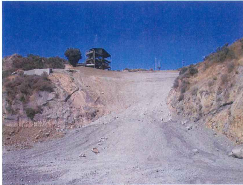
Photo 21: Looking west at fill placed in a drainage to mitigate past slope failures below conveyor that deposited limestone waste rock into EMSA drainage. Slopes will be hydroseeded before this winter. Compare with Photo 14 in 2013 Annual Inspection report. Dated September 3, 2015.
