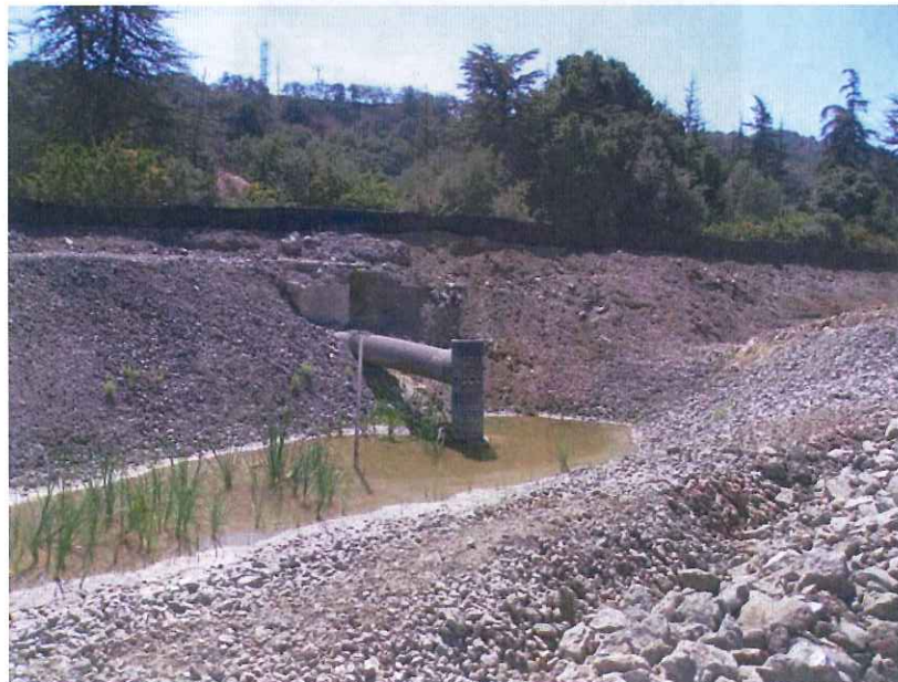
Photo 18: Pond 30 with outfall that discharges into Permanente Creek. Dated September 3, 2015.
