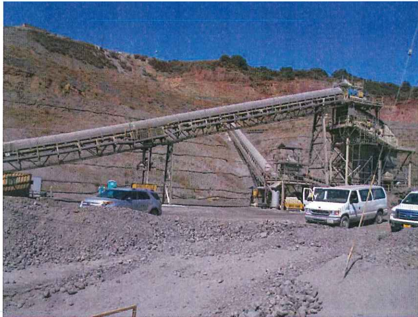
Photo 23: New crusher area conveyors looking northeast. Dated September 3, 2015.
