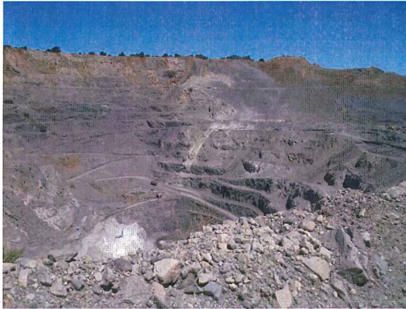
Photo 3: North Quarry eastern highwall at left side of photo. Upper portion near final reclamation grade. Mid-Pen Rockslide in right center of photo. Dated September 3, 2015.
