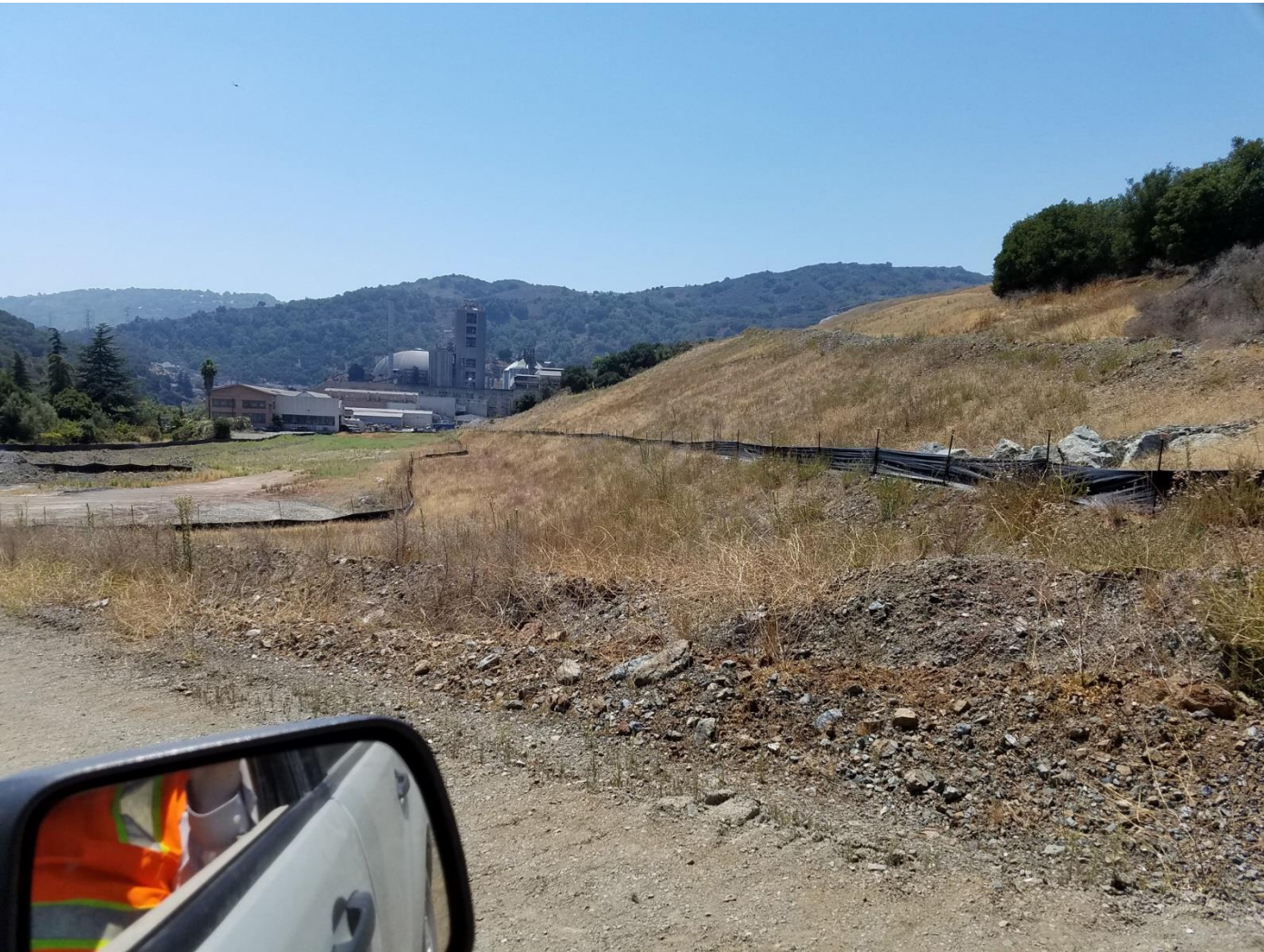
PHOTO #8 taken from Map Location 110 – EMSA bench with silt fence (looking west)
