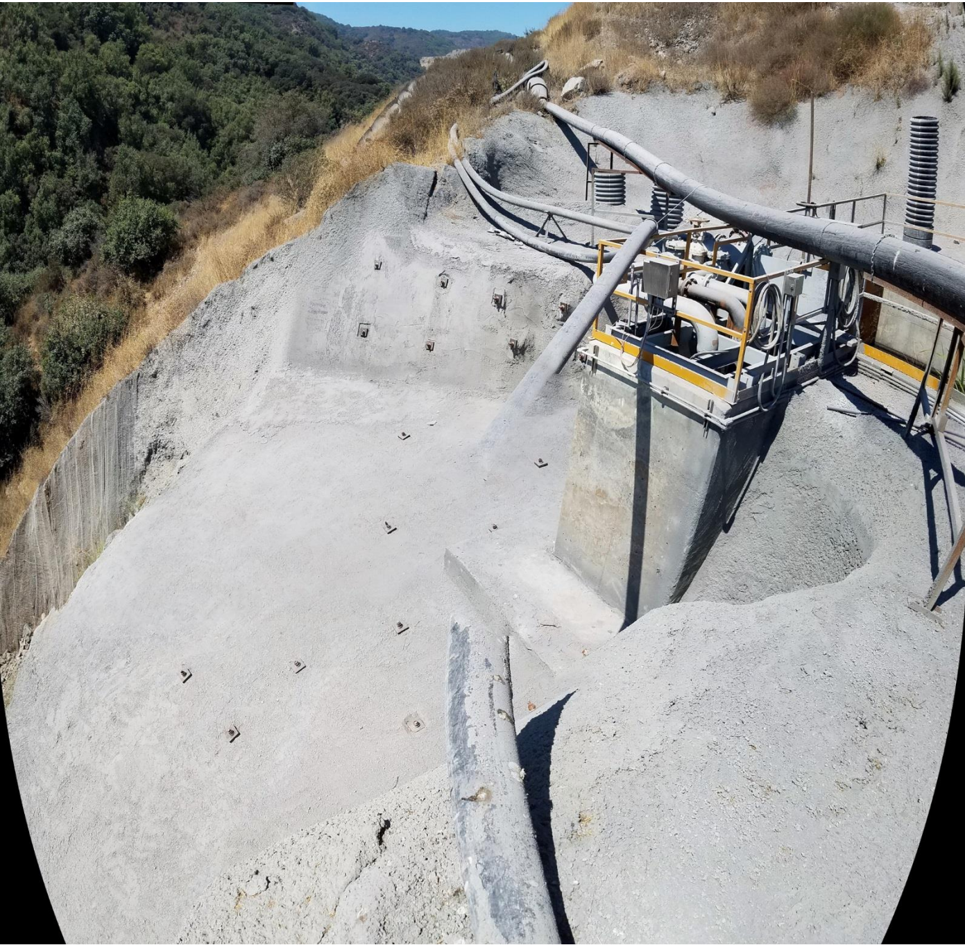
PHOTO #12 taken at Map Location 77 – Soil-nail wall in erosion scar below crusher sump
