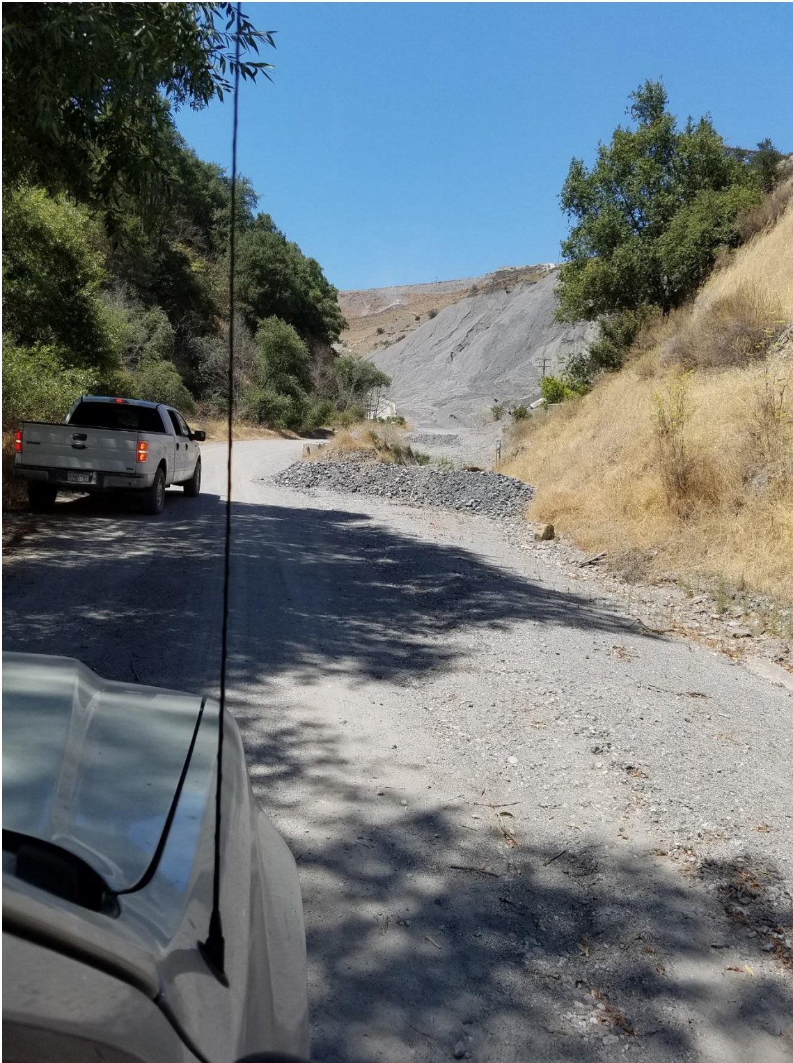
PHOTO #14 taken at Map Location 113 – Rock check dam on road below Surge Pile
