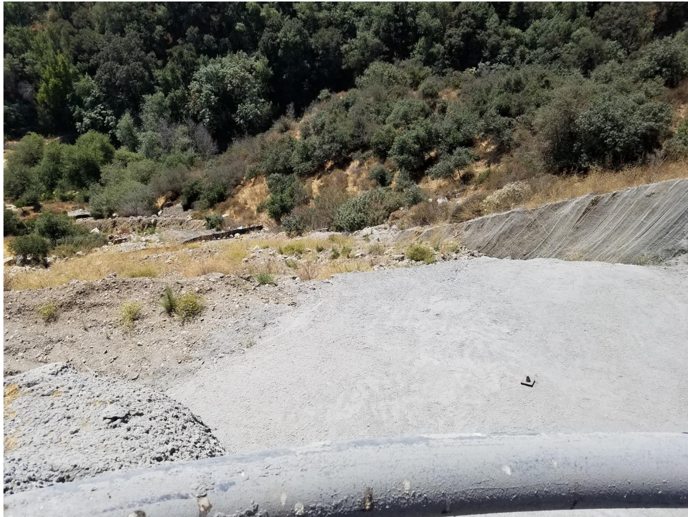
PHOTO #10 taken from Map Location 81 – Jute netting lined erosion gully below crusher sump
