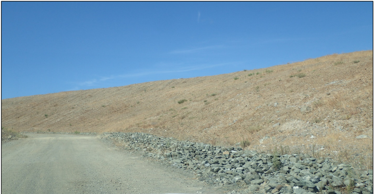
Photograph 4. Non-limestone lined stormwater ditch and previously hydroseeded slope along EMSA haul road. Photograph taken September 2, 2016.
