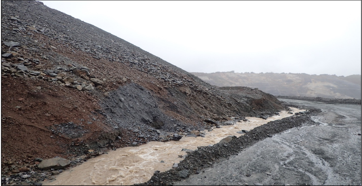
Photograph 5. Functioning stormwater ditch along the inside of the WMSA haul road.
