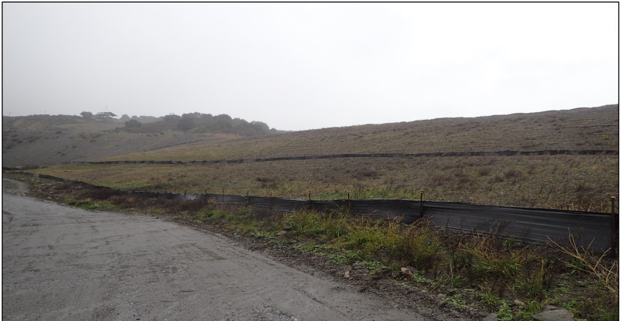
Photograph 6. Erosion control straw wattles and silt fences installed on interim reclaimed slopes in the EMSA.
