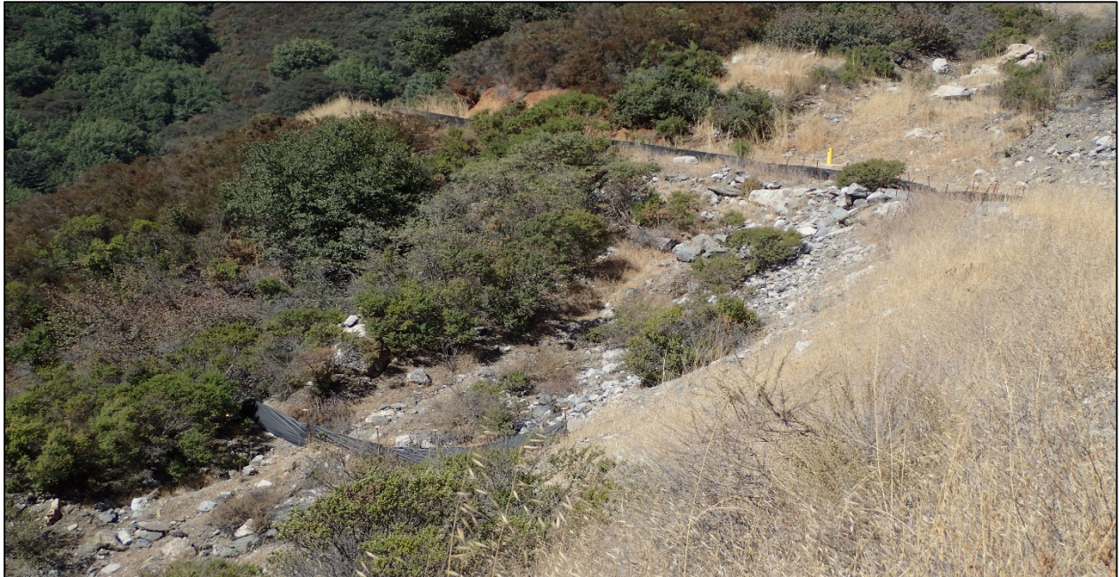
Photograph 1. Wire-backed erosion control silt fence installed on downhill side of access road in PCRA Subarea 1.
