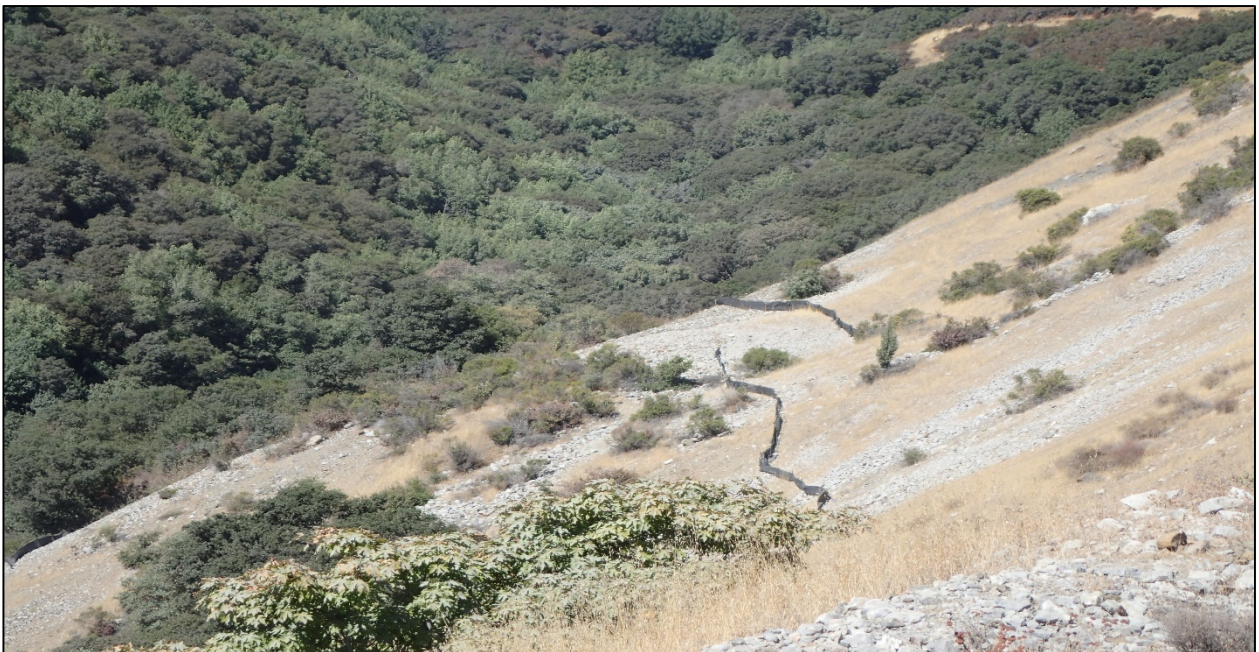
Photograph 2. Wire-backed erosion control silt fence installed below new mining activity in PCRA Subarea 2.
