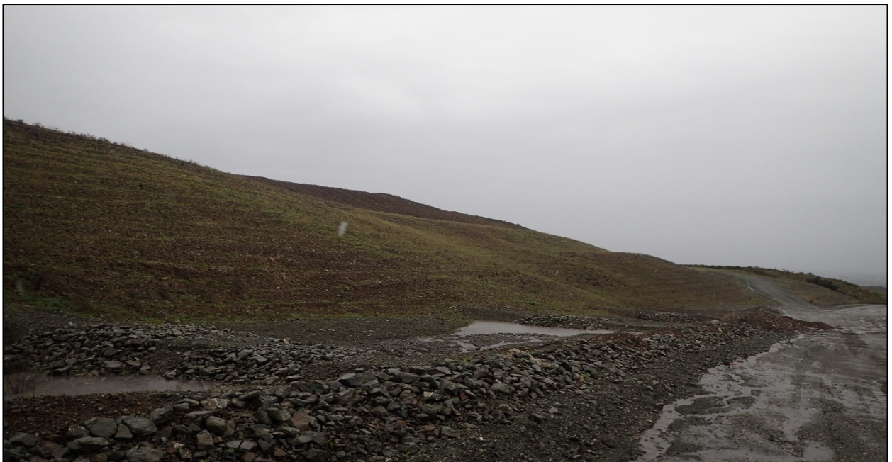
Photograph 8. Functioning check basins along EMSA haul road during a qualifying rain event.
