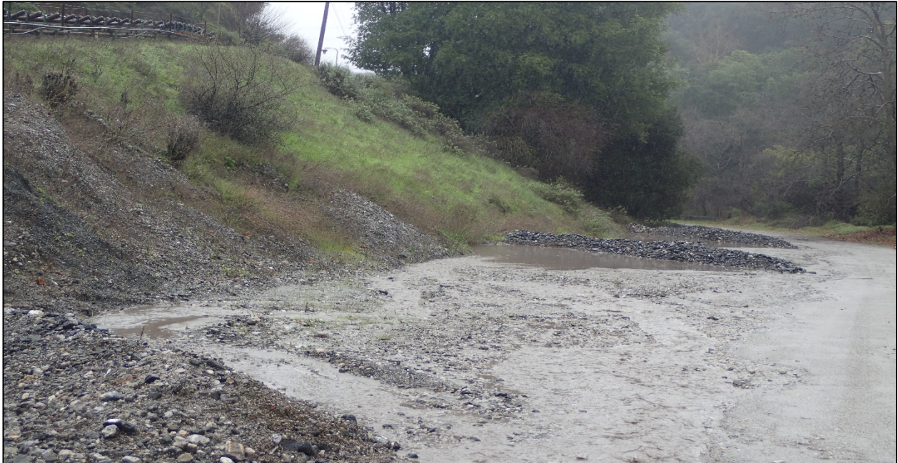
Photograph 7. Functioning check dams as see during a qualifying rain event
