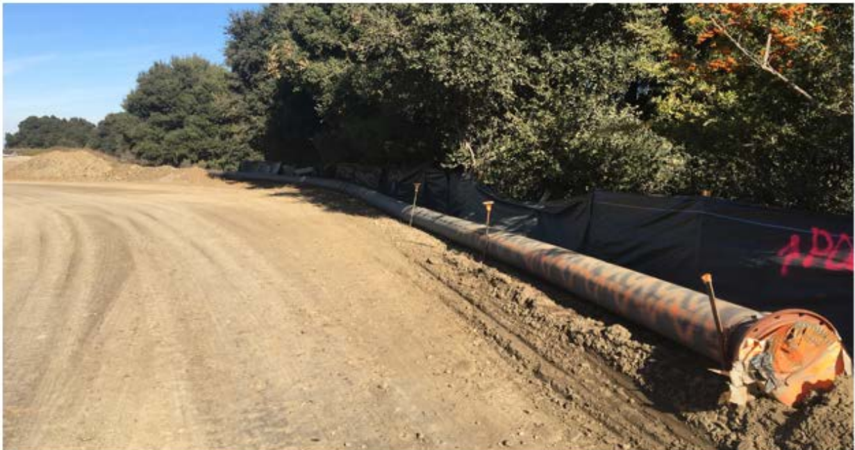
Picture 2: New 12" HDPE pipeline on the right at Pond 30 area
