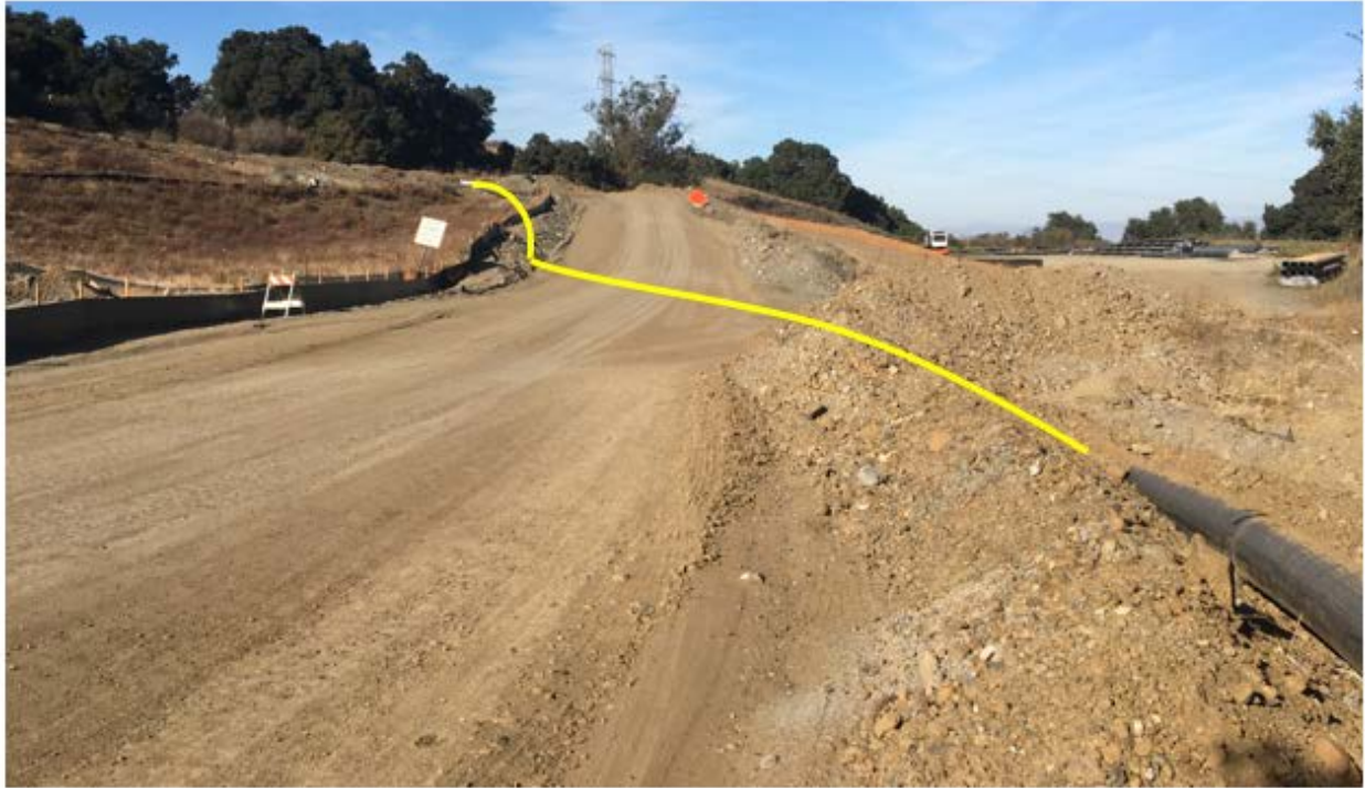
Picture 3: New 12" pipeline on the right going underground entering EMSA
