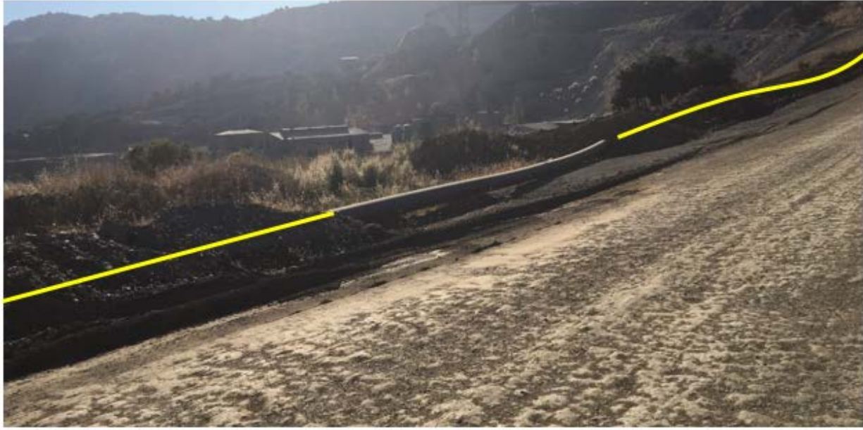
Picture 5: Exposed new 12" pipeline in EMSA by D10 ditch to allow Stormwater drainage
