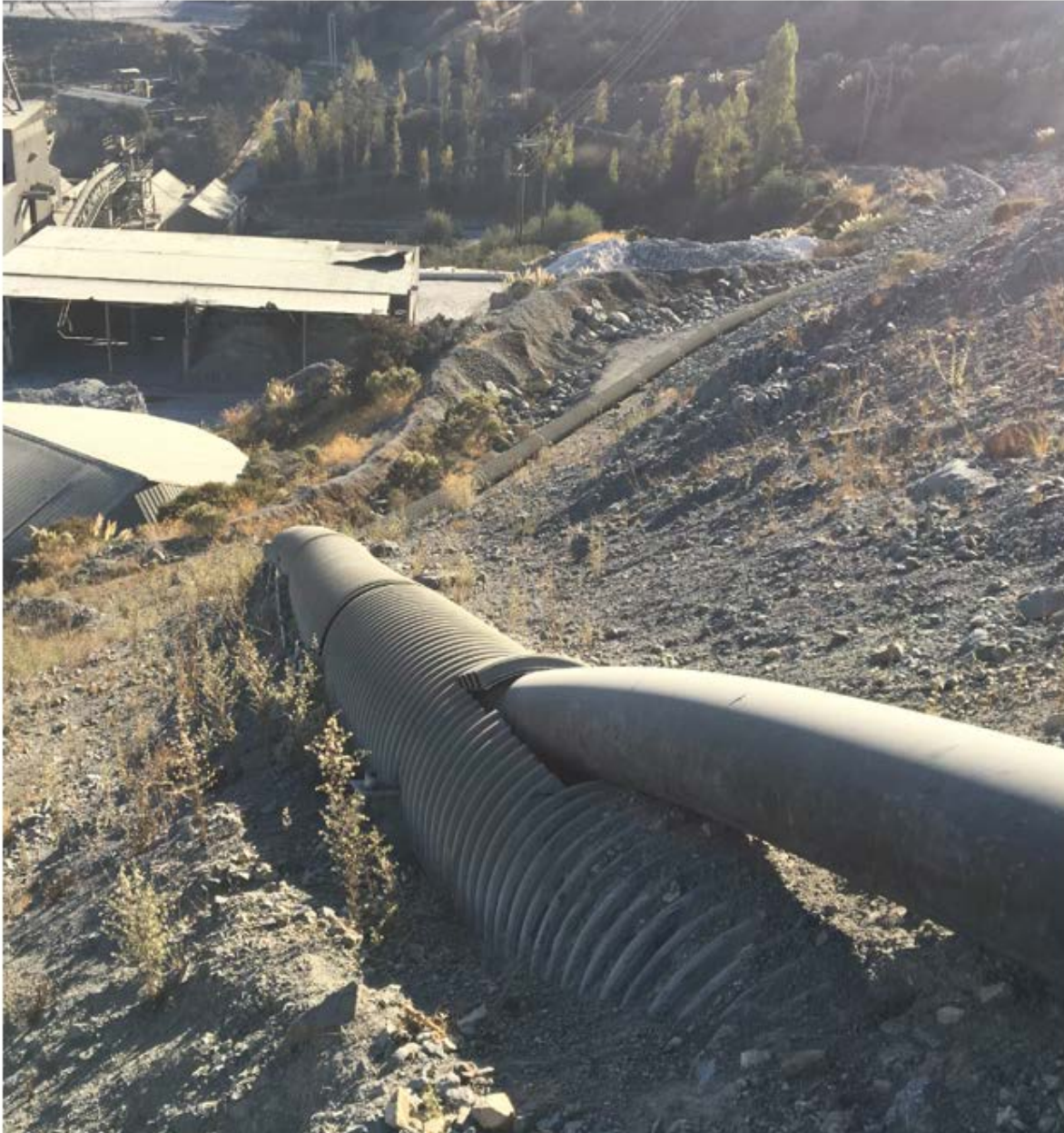
Picture 7: Close-up picture of the exposed new 12" pipeline from pond 30 area connecting 30" corrugated pipeline
