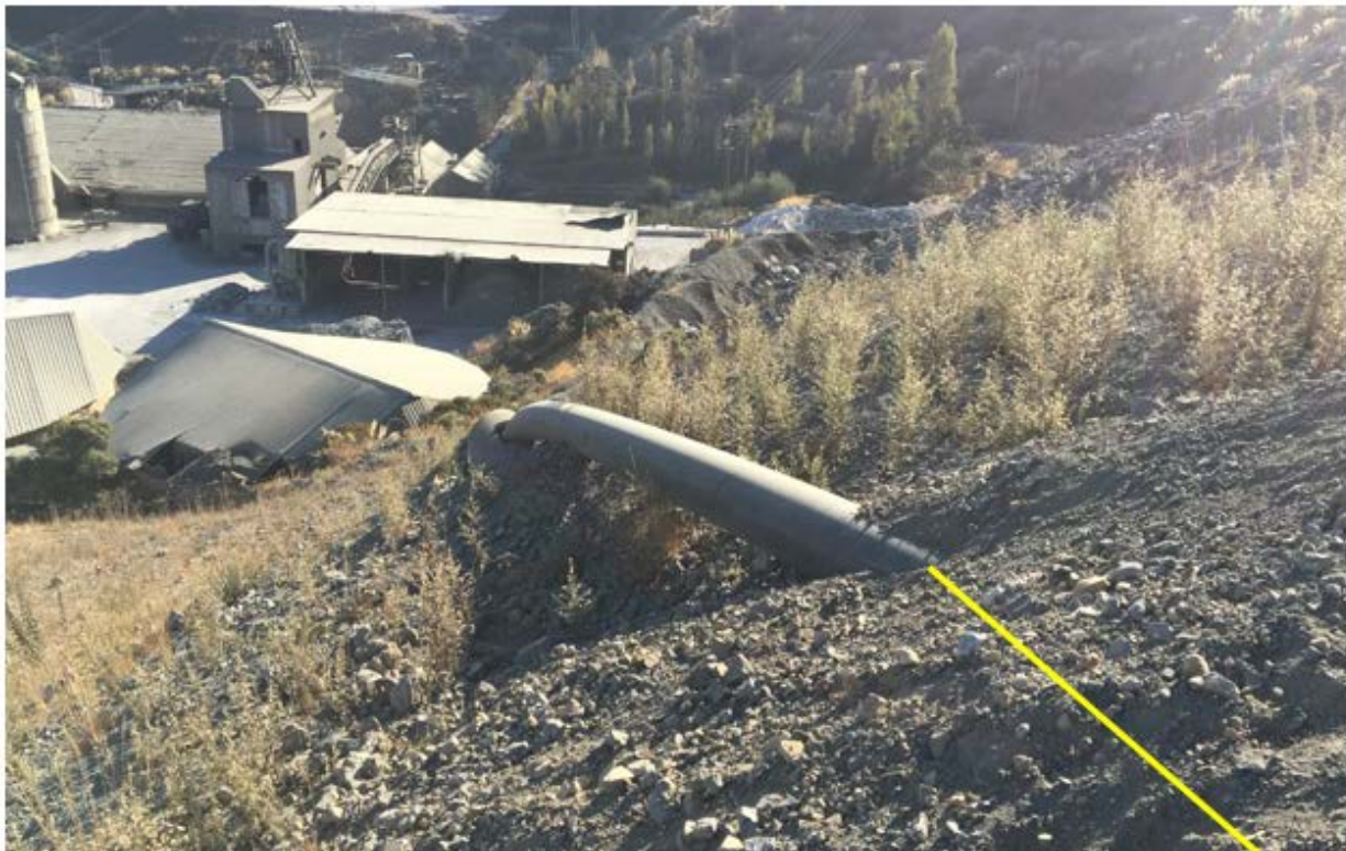
Picture 6: Exposed new 12" pipeline connecting 30" corrugated pipeline
