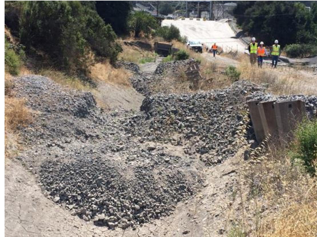
PHOTO #15 – Check dams and failing sheet pile wall leading to Pond 17
