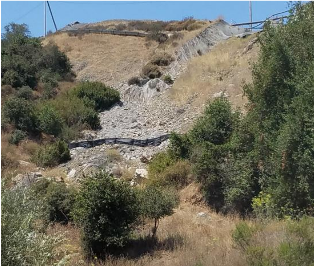
PHOTO #10 –Debris track below crusher sump
