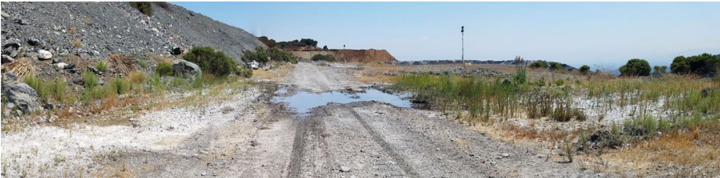
PHOTO #6 – Seep at top of haul road buttress
