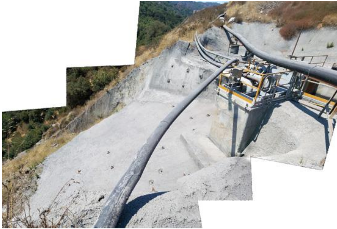
PHOTO #12 – Tie-back wall at crusher sump
