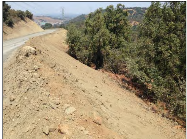
Figure 3 Utility Road Fill Profile
