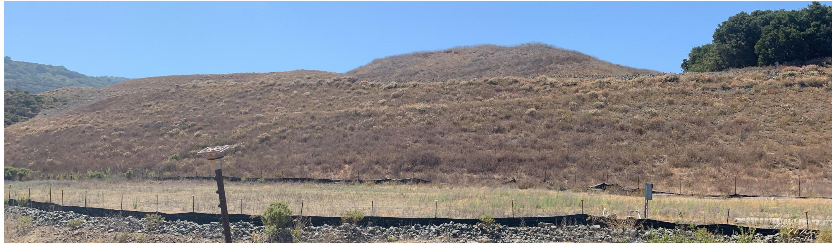
County inspectors observed substantial vegetation growth on the EMSA slopes. [See PHOTO #8 .]
