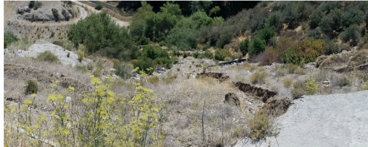
PHOTO #10A – Overflow scar below crusher sump
