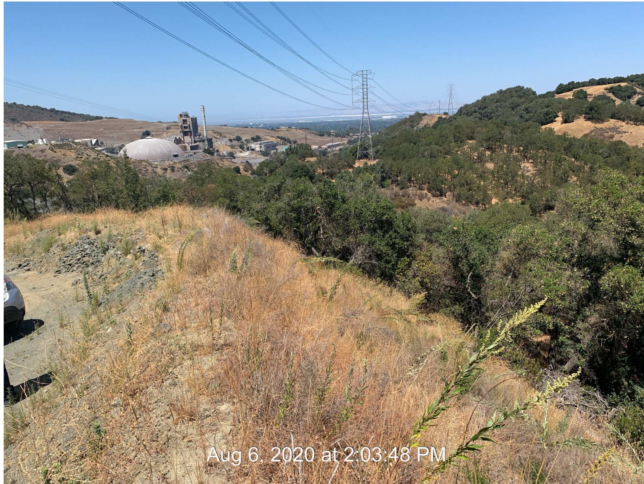
Photo #21B Fill slope below east side of illegally graded haul road
