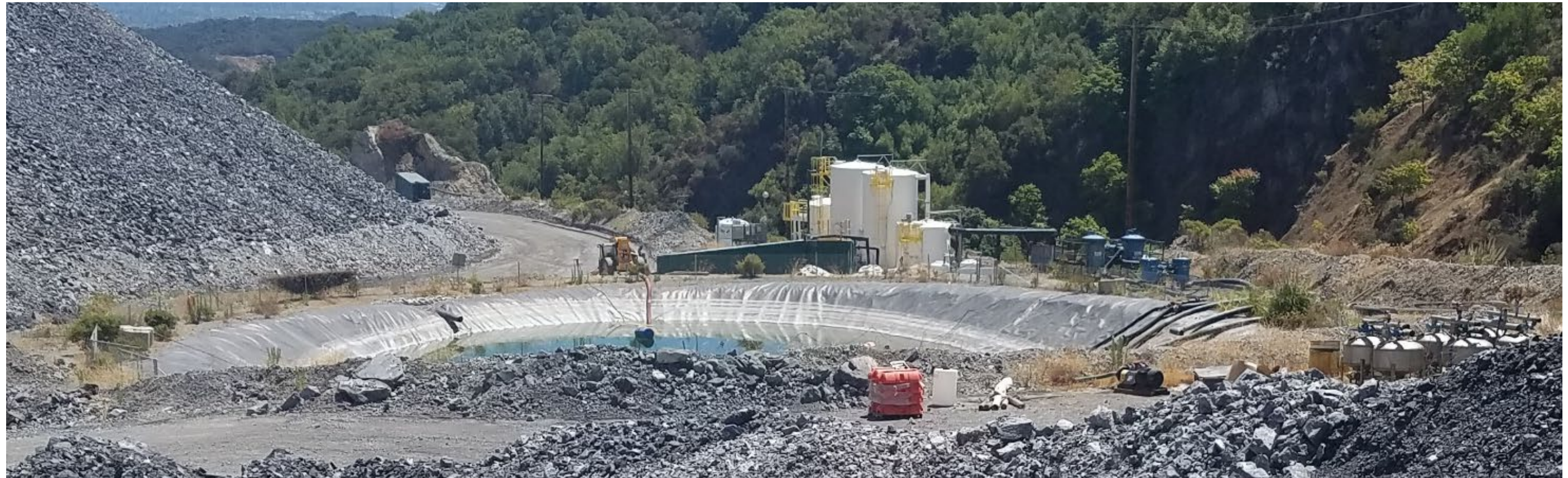
.Associated tanks are located adjacent to Pond 1250. [See PHOTO #19. ]
