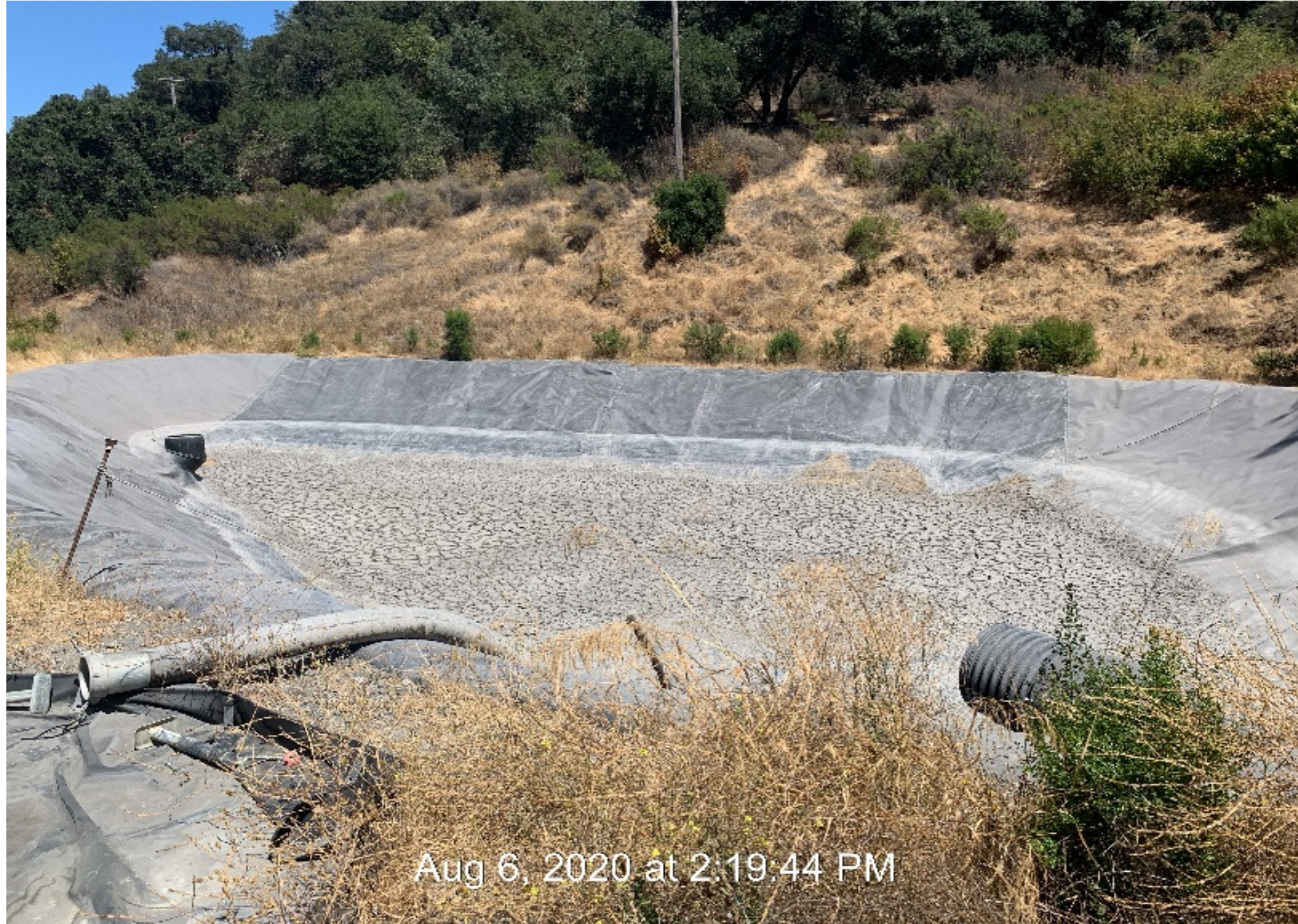
PHOTO #16 – Pond 17 with liner and sediment
