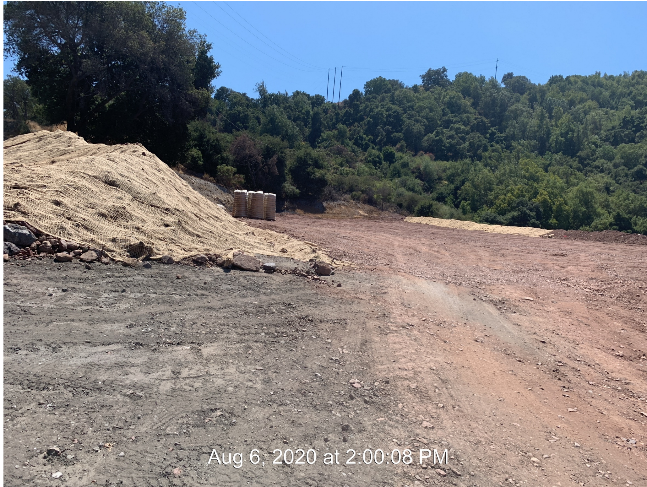
Photo #28B – recently cut pad near Rock Plant
