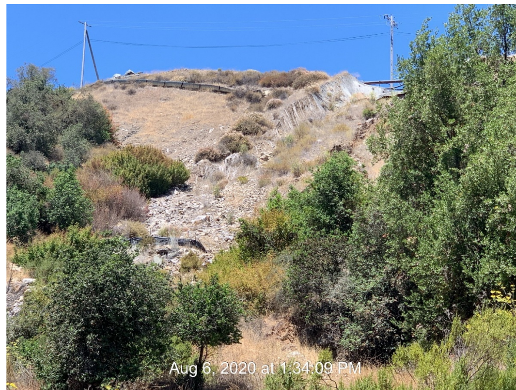
PHOTO #10B – Debris flow track below crusher
