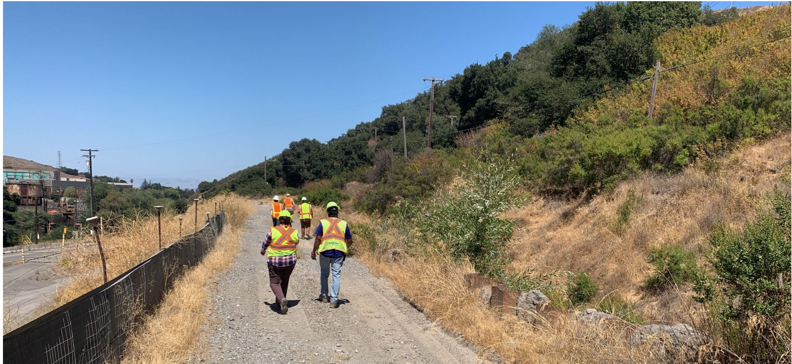
PHOTO #15 – In-flow to Pond 17 and failing sheet pile wall
