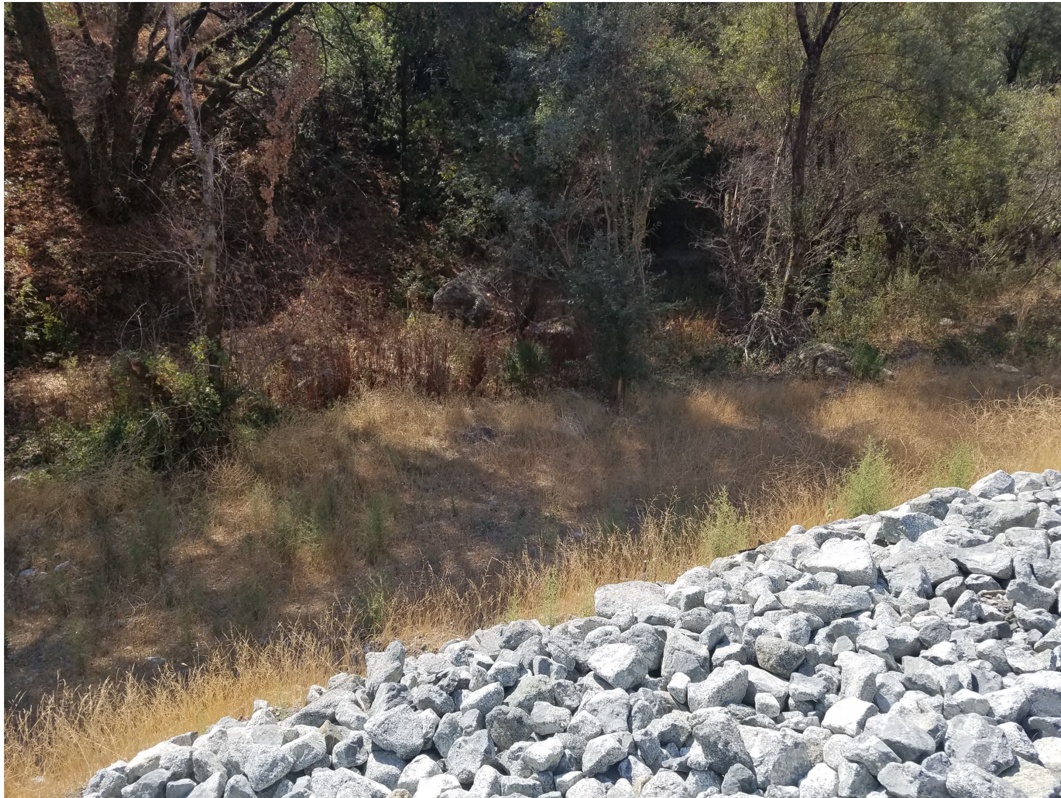
Photo #25 – Rock armor added to area where sediment was deposited into Permanente Creek from Yeager Yard slope
