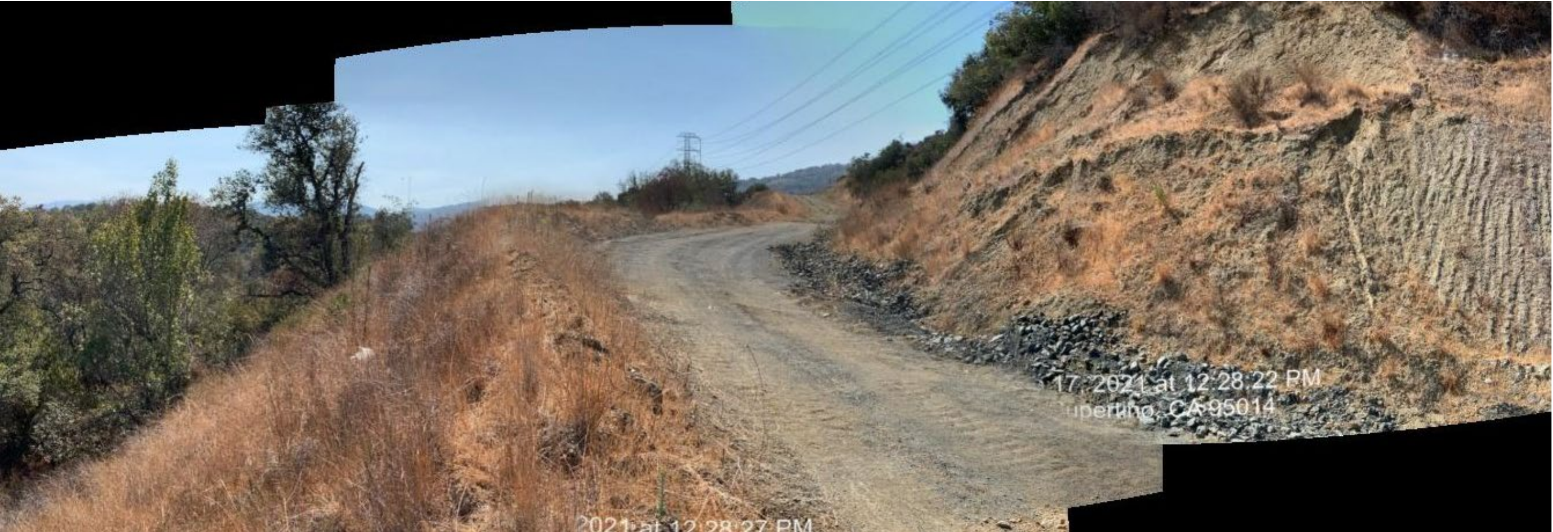
Photo #21A – Cut slope and drainage ditch on west side of unpermitted haul road
