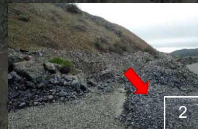
Water bars were re-established along the WMSA Access Road
