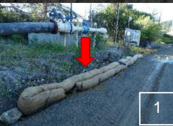
Straw wattles were replaced throughout the quarry.
