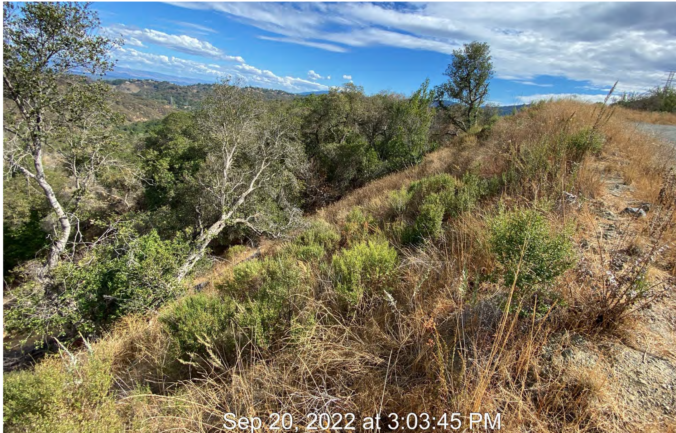
Photo #21B Fill slope below east side of illegally graded haul road
