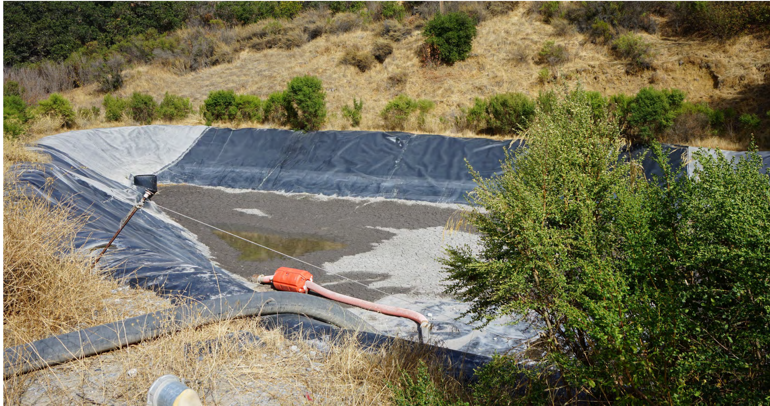
Pond 17 has been decommissioned and the runoff which was previously routed to Pond 17 now flows into a new basin in Permanente Creek installed at the direction of the San Francisco Bay Regional Water Quality Control Board.
