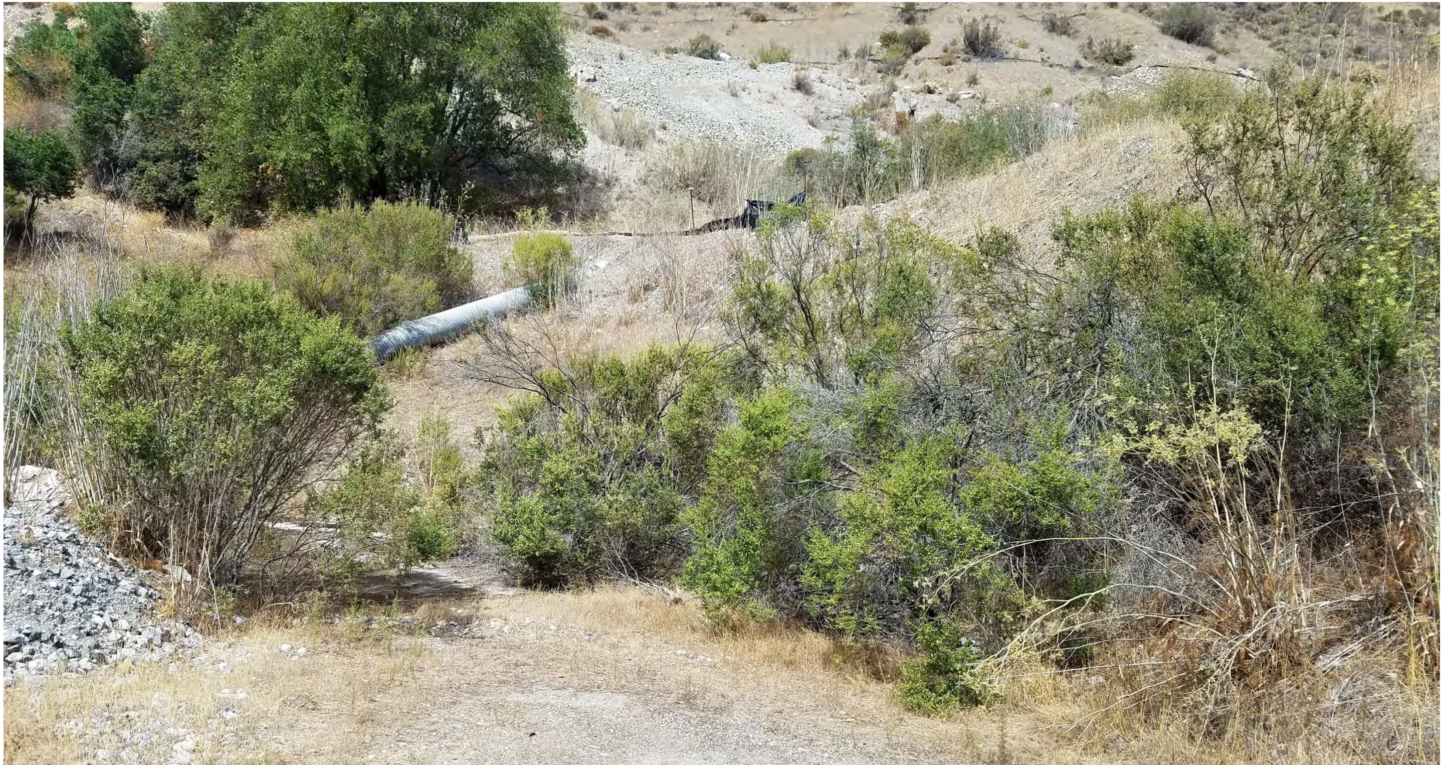
Sediment that erodes from the surge pile is detained in ponds. Next to the surge pile are slopes above Pond 13.
