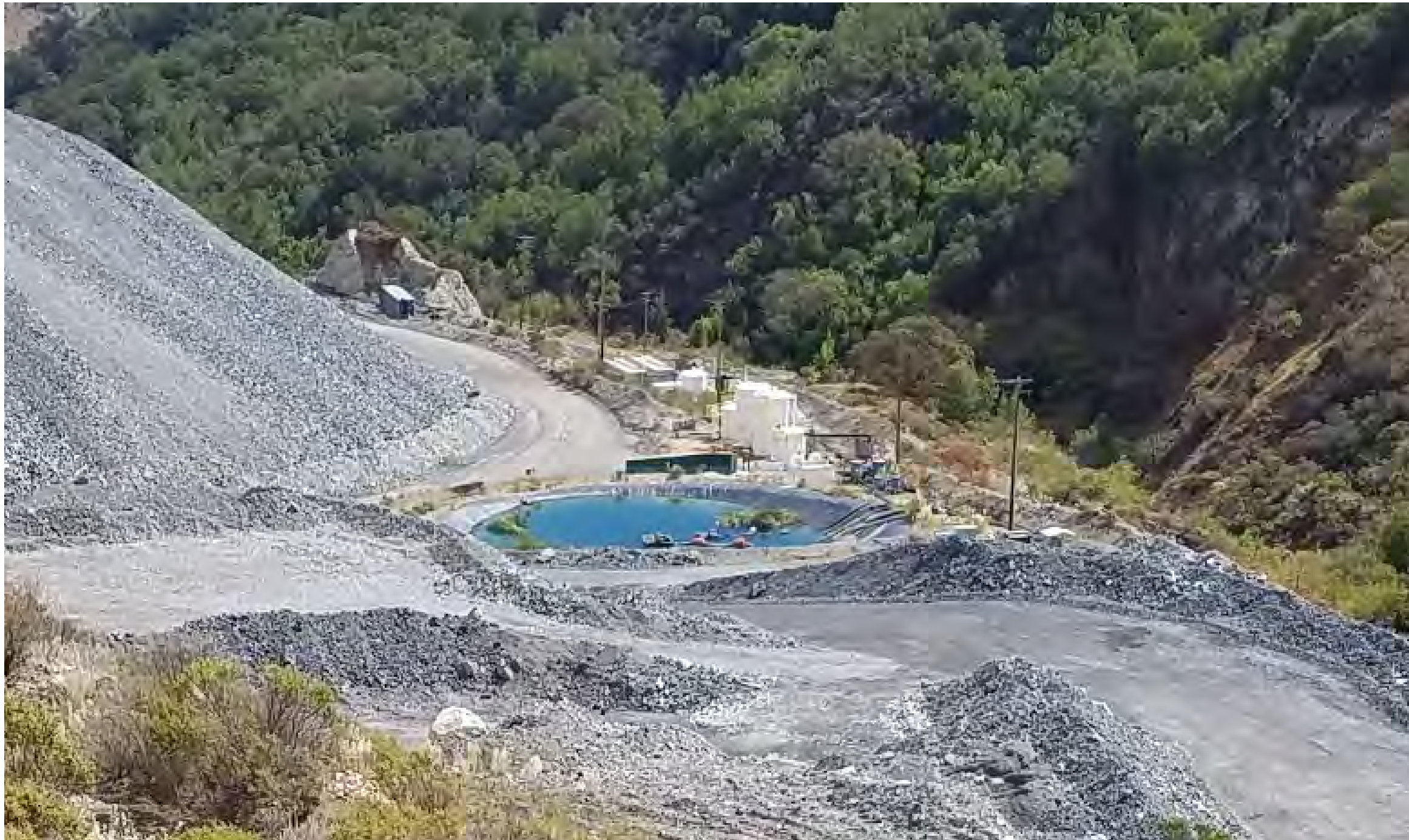
Associated tanks are located adjacent to Pond 1250.
