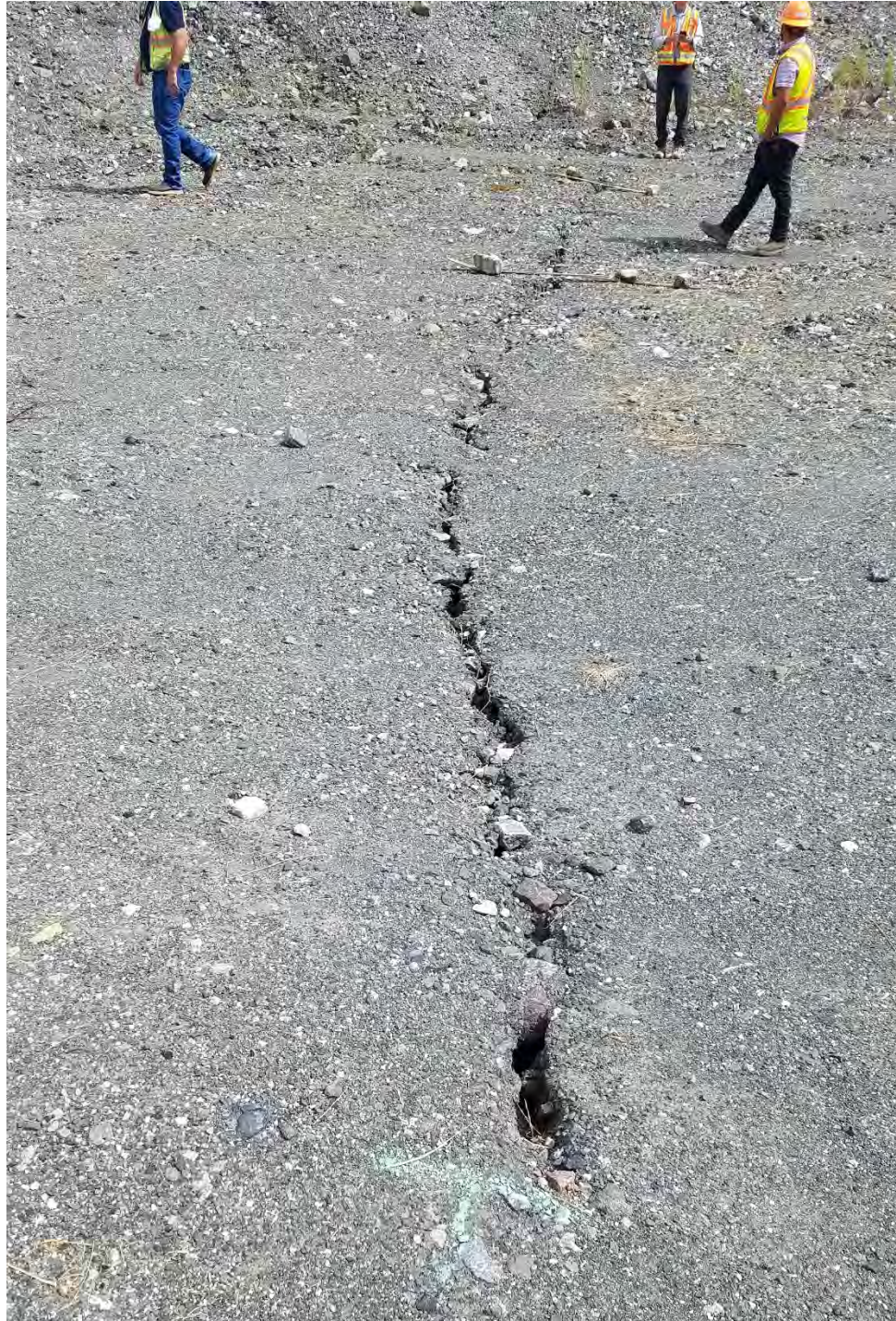
Photos #30A, B and C – Recently formed ground cracks near eastern portion of Yeager Yard slide. (Monitoring sticks placed by Operator.)
