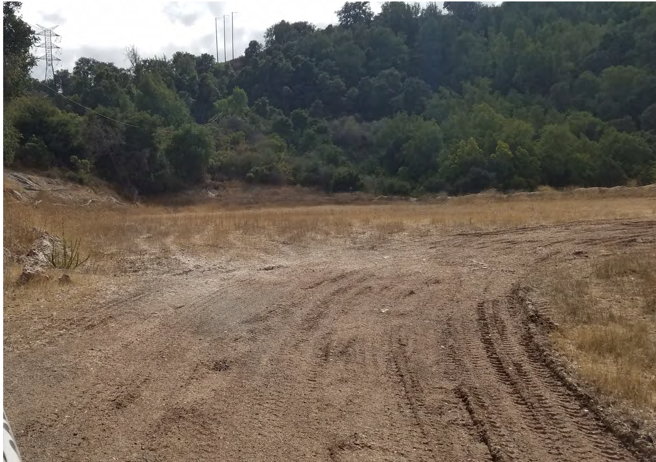
Photo #28B – recently cut pad south of Rock Plant
