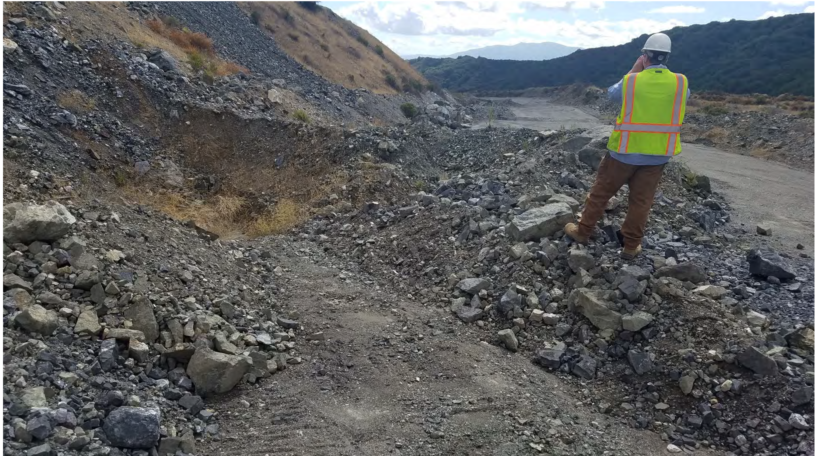
PHOTO #20 – Check dam on the WMSA road
