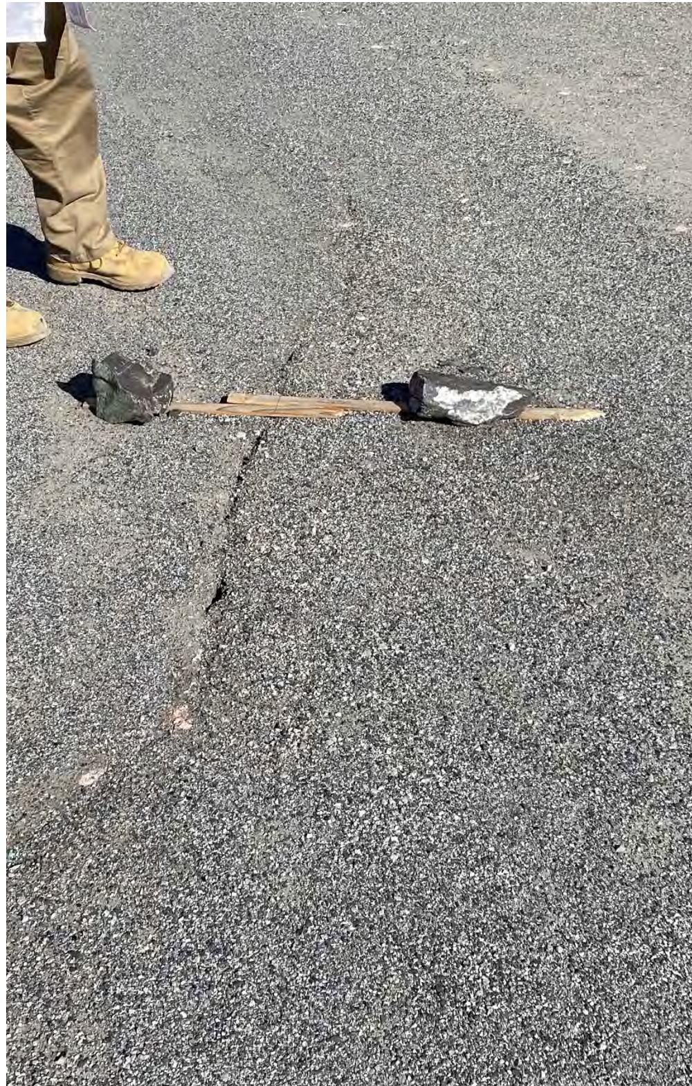
Photos #31A and 31B – Recently formed ground cracks along road to main pit observation deck. (Monitoring sticks placed by Operator.)
