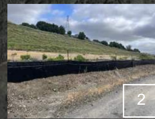
Silt fences were installed around Pond 30.
