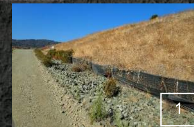
Silt fences were re-established along the Upper EMSA Access Road.
