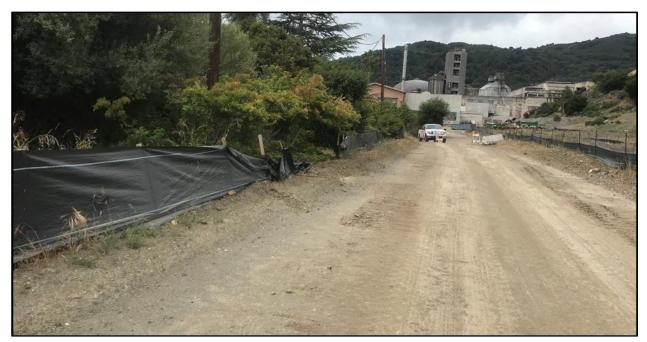
Missing silt fencing along the main road near Pond 30.
