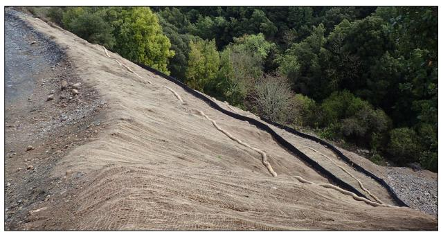
A large section of jute netting, wattles and silt fencing placed below the Yeager Yard along the hillslope to arrest any potential erosion during the rainy season.
