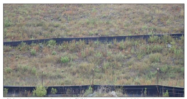
Silt fencing shown above (located in the EMSA) was recommended to be left in place, but no longer actively maintained. The fully vegetated hillslope shown in the photo is effectively holding topsoil in place.
