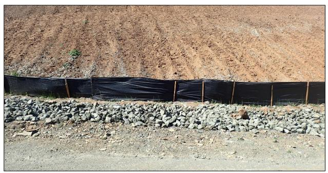
A section of silt fencing with hydroseeding on the topsoil pile within the EMSA were addressed and functional.
