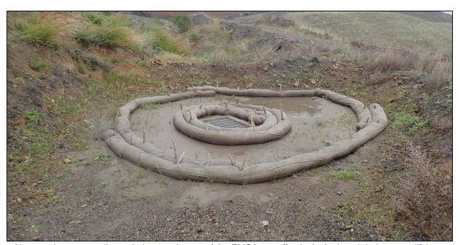
New wattles surrounding a drain near the top of the EMSA are effectively deployed during a qualifying event on April 6, 2018.
