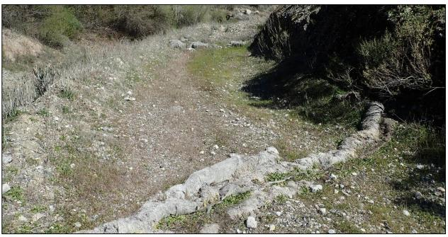
Degrading wattles were noted to be replaced near Pond 13. The WRA QSP/QSD also suggested that if this area was to become active in the future, wattles should be replaced by waterbars.
