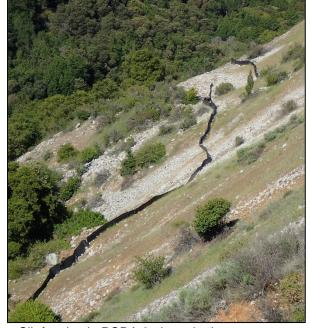
Silt fencing in PCRA 2 along the lower boundary of the slope.
