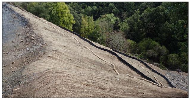
A section of jute netting, wattle and silt fencing along the hillside between the Yeager Yard and the Quarry Pit. Installation was completed before rain events occurred in March.
