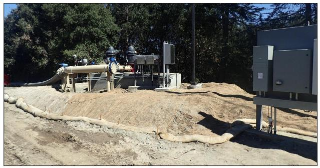
Following installation of new pumps around Pond 30, jute netting and wattle were installed around the new pump station to prevent erosion while seed takes hold.
