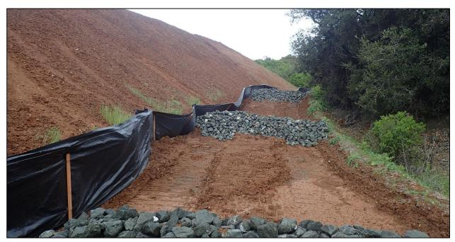
Rock check dams effectively slowing flow along a roadway in the EMSA.
