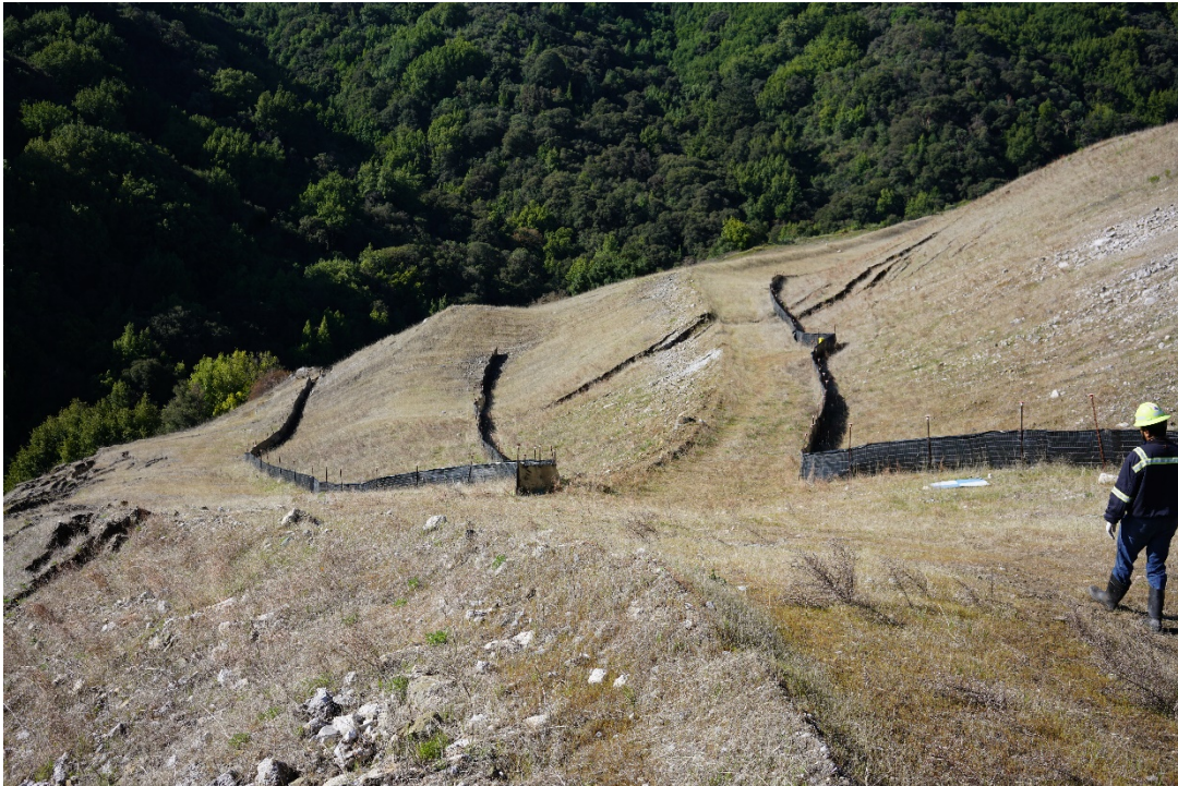
Photo 6. Silt fences on upper slopes of the Yeager Yard. All silt fences on the upper slopes of the Yeager Yard were repaired, or removed where no longer functional.
