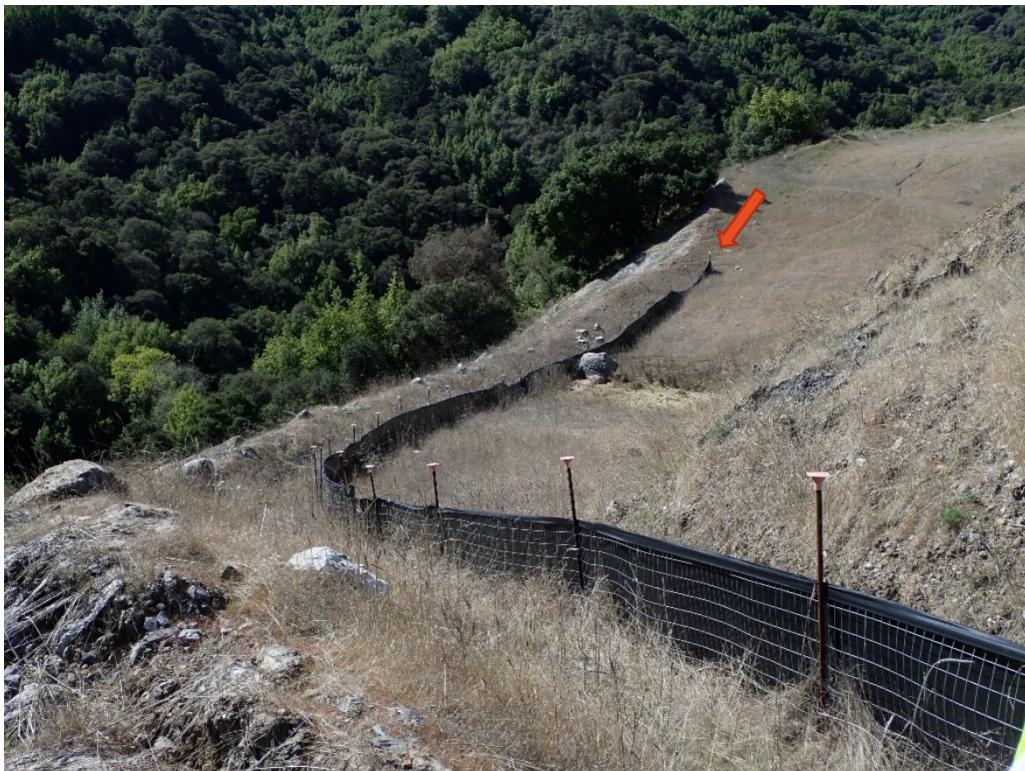
Photo 4. Silt fence on upper slopes of the Yeager Yard. Short segment of silt fence is down below hydroseeded slopes with established vegetation.
