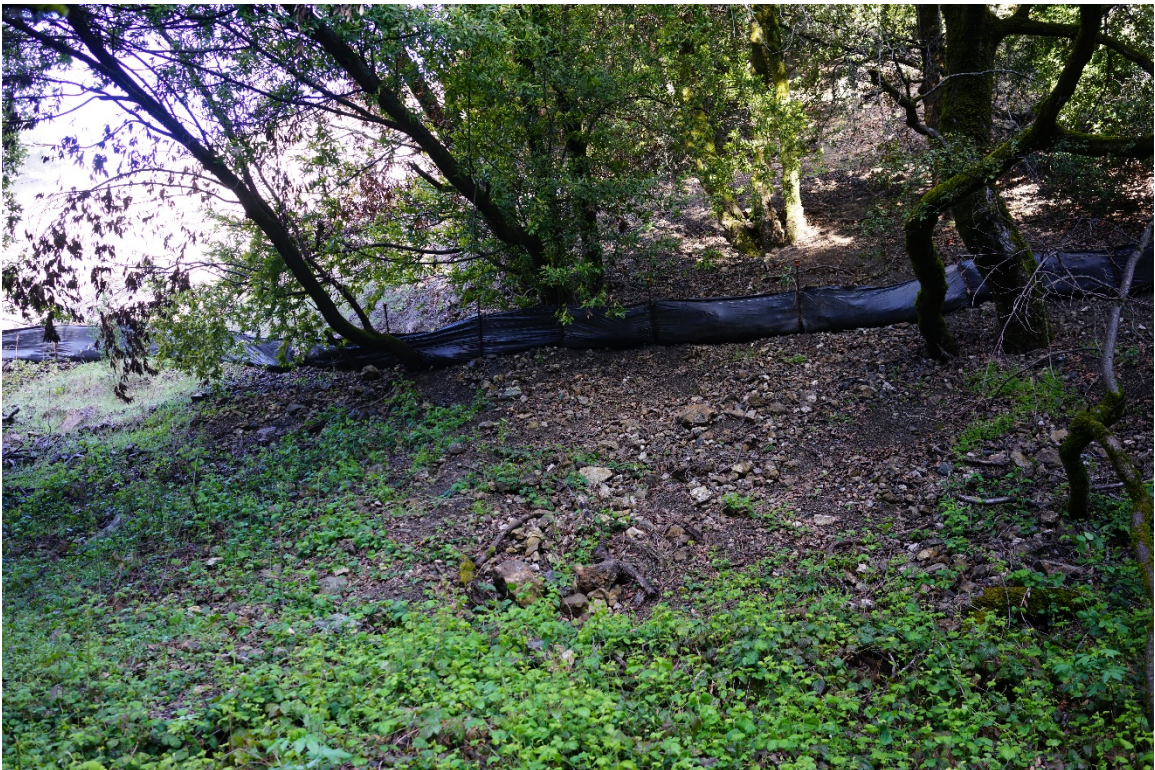
Photo 8. Silt fence above Permanente Creek on the lower slopes west of sediment capture basin.
