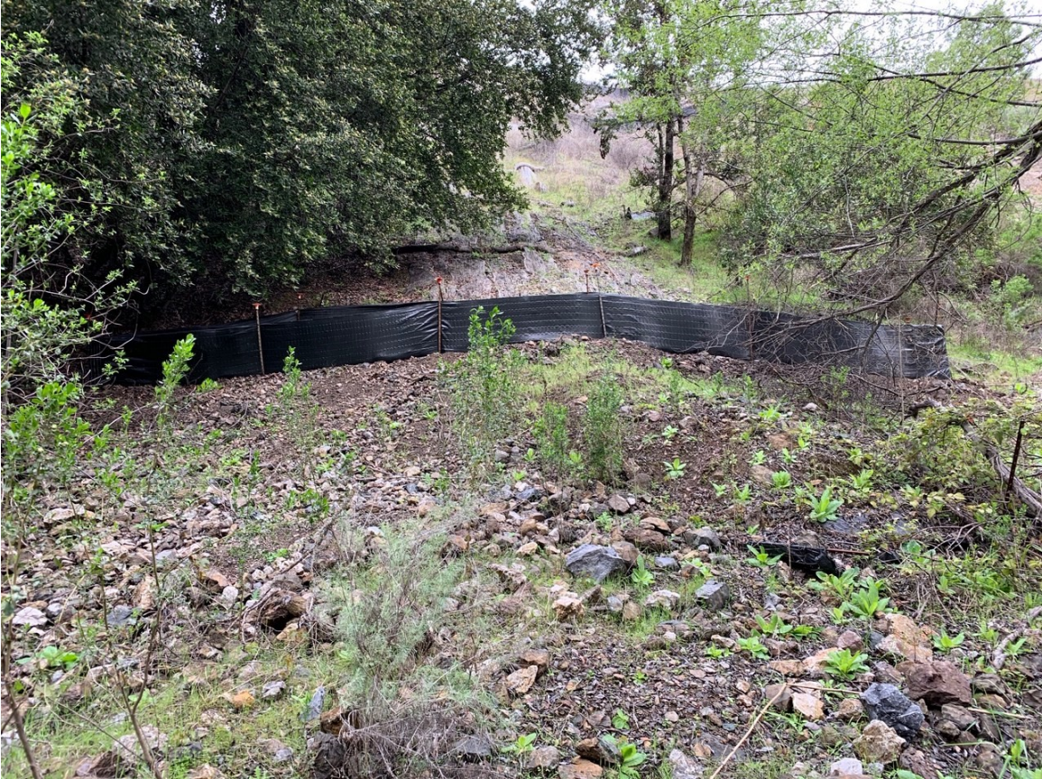
Photo 11. Detail of additional line of silt fencing installed upslope from the existing silt fence above Permanente Creek on the lower slopes west of sediment capture basin.
