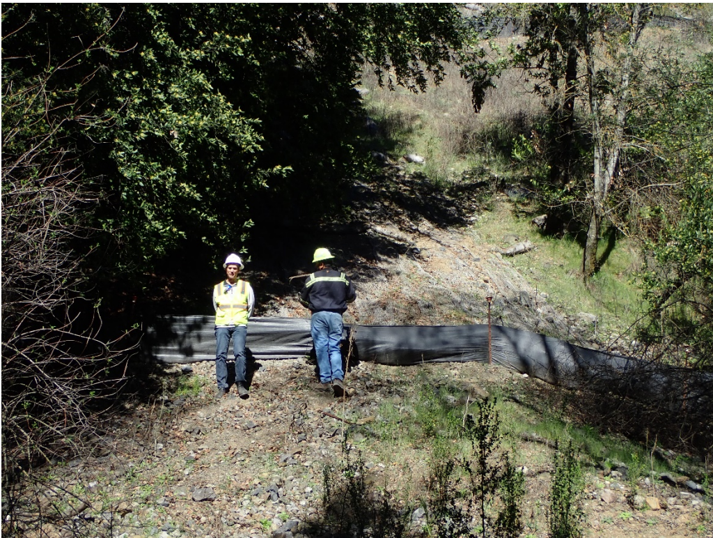
Photo 2. Detail of silt fence above Permanente Creek on the lower slopes west of sediment capture basin.
