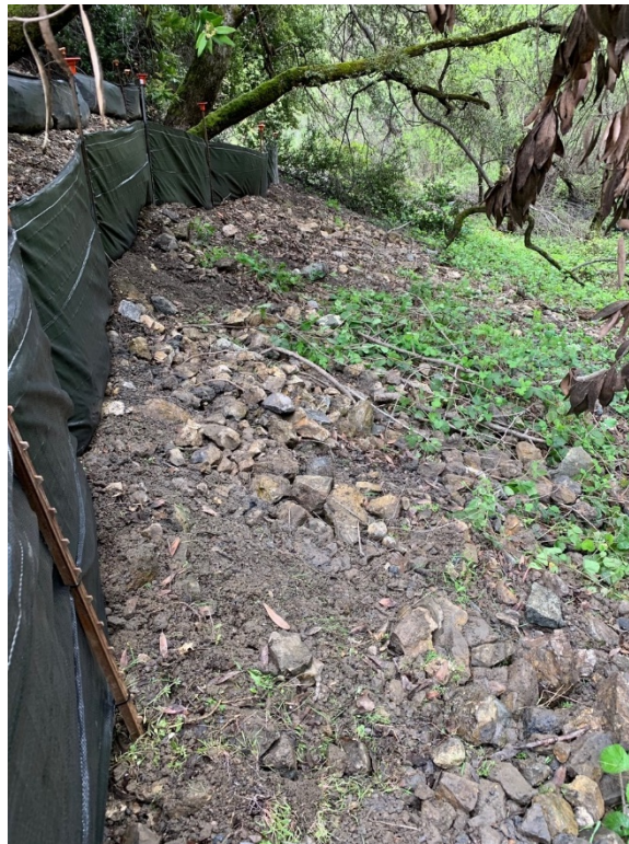
Photo 10. Detail of additional line of silt fencing installed downslope from the existing silt fence above Permanente Creek on the lower slopes west of sediment capture basin.
