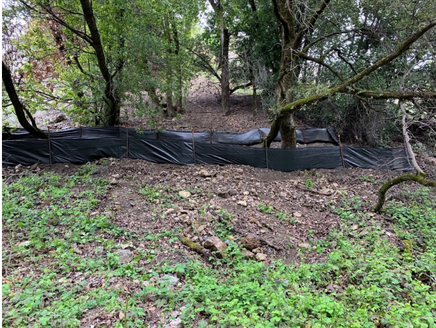
Photo 9. Additional line of silt fencing installed downslope from the existing silt fence above Permanente Creek on the lower slopes west of sediment capture basin.
