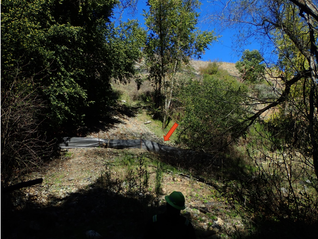
Photo 1. Silt fence above Permanente Creek on the lower slopes west of sediment capture basin.
