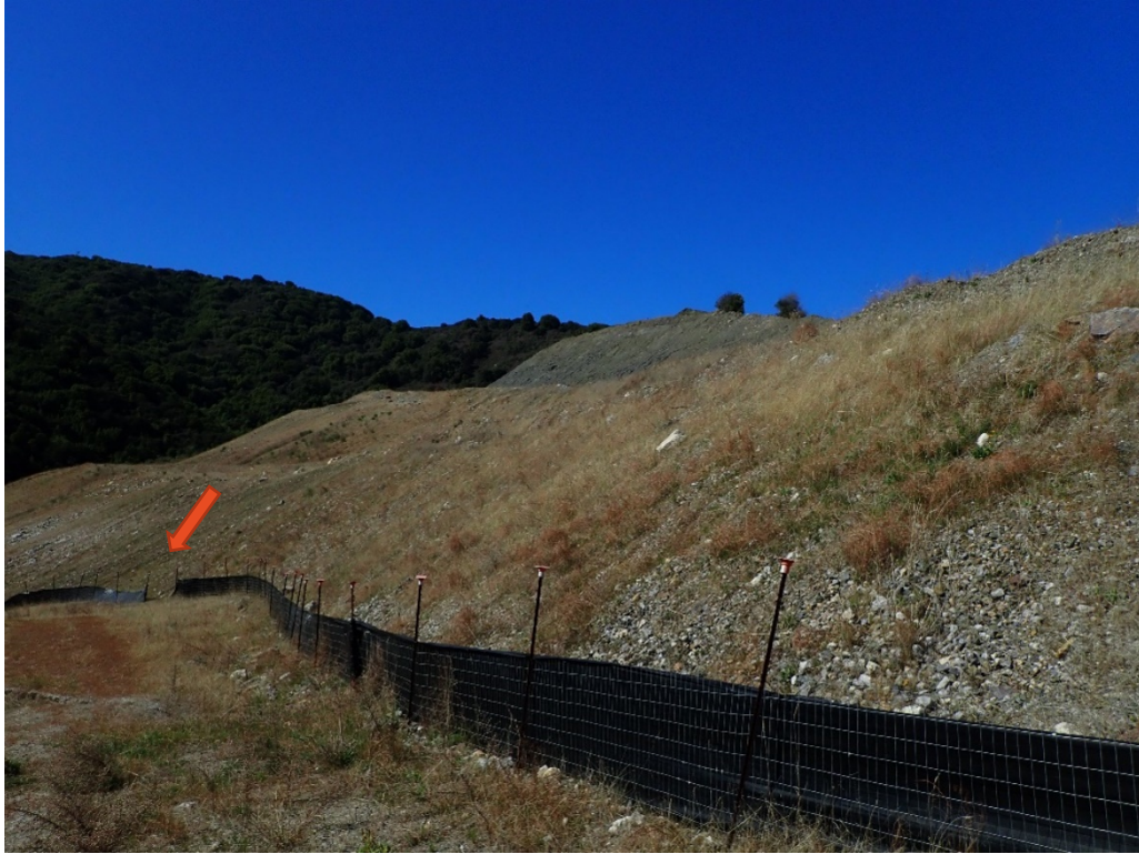
Photo 3. Silt fence on upper slopes of the Yeager Yard. Short segment of silt fence fabric is down below hydroseeded slopes with established vegetation.
