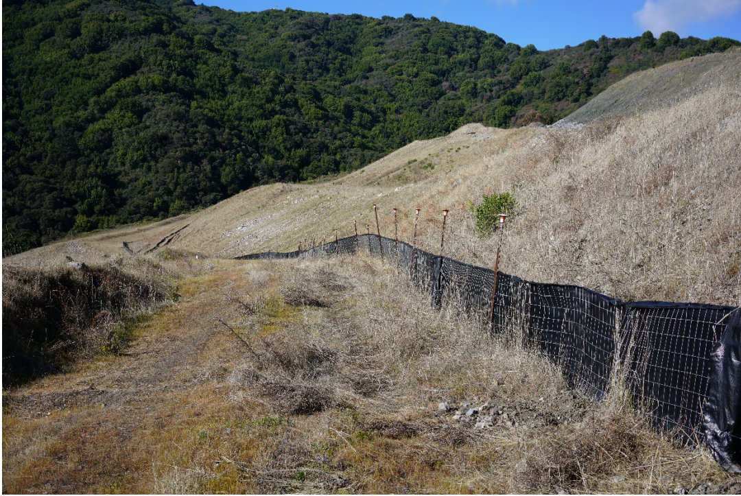
Photo 5. Silt fence on upper slopes of the Yeager Yard. Short segment of silt fence fabric is down below hydroseeded slopes with established vegetation.
