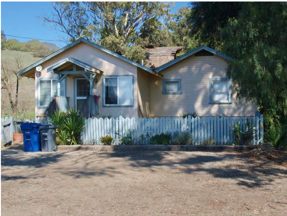
Front elevation of house, viewed facing northeast.
