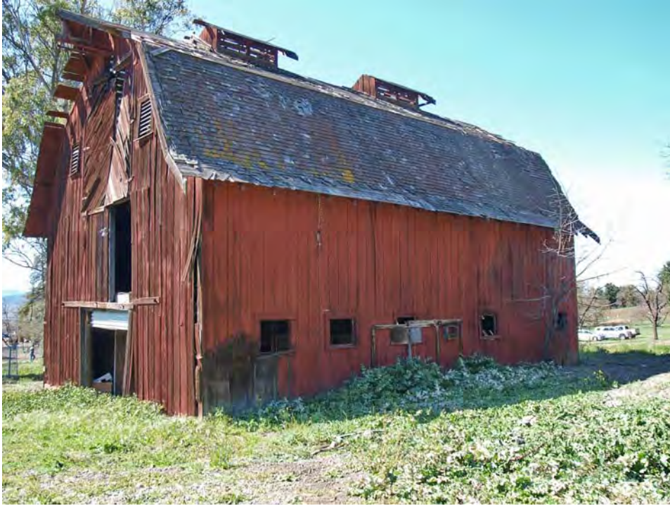
Barn, viewed facing northwest.
