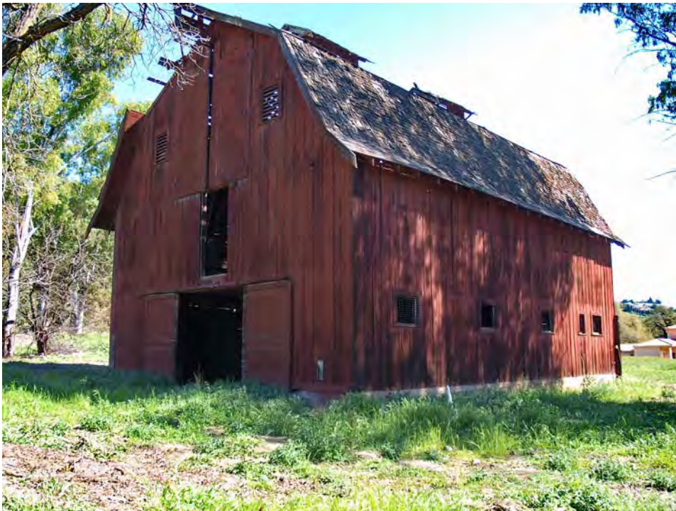
Barn, viewed facing southeast.
