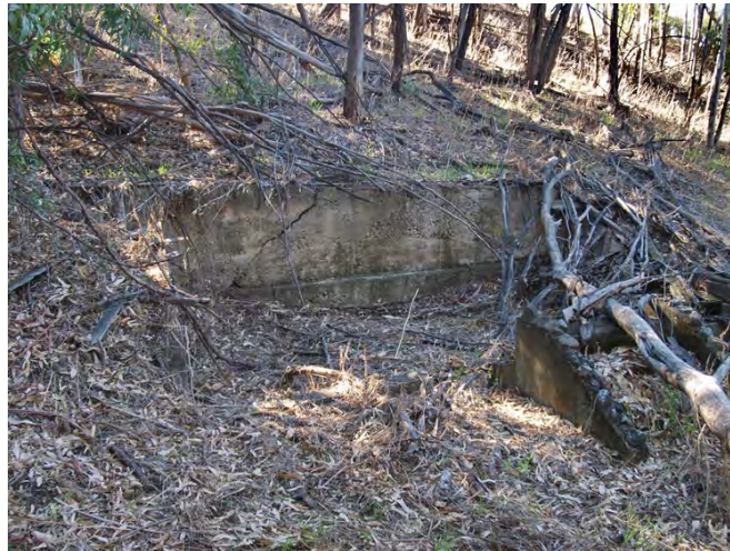
Concrete footings in canyon above Santa Catharina Avenue.
