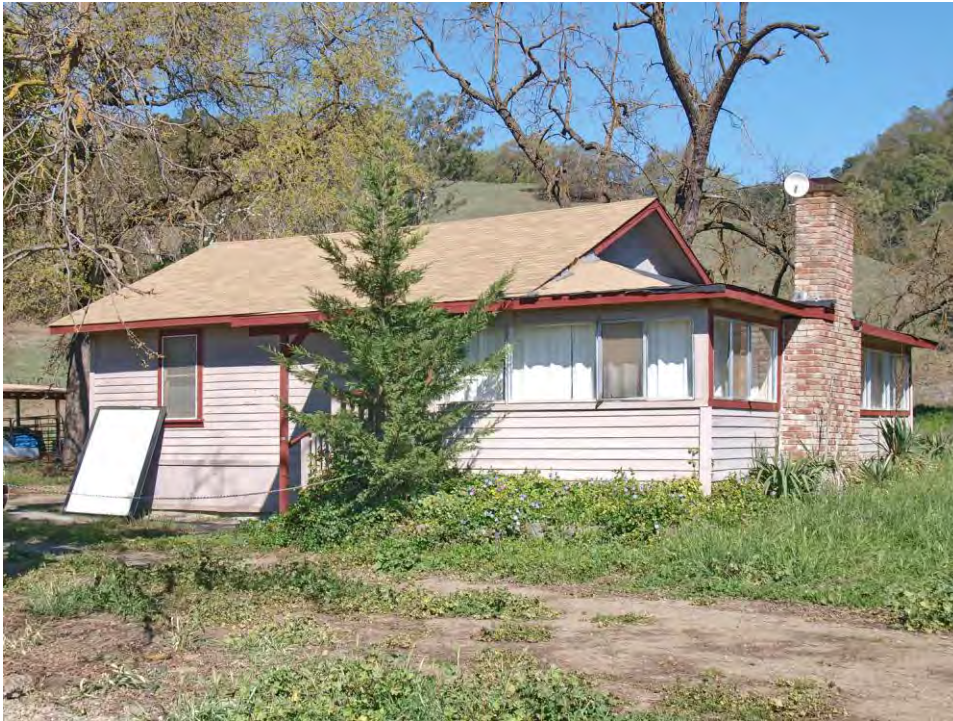
Front elevation of house, viewed facing northeast.
