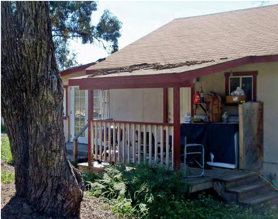
Rear elevation, viewed south.
