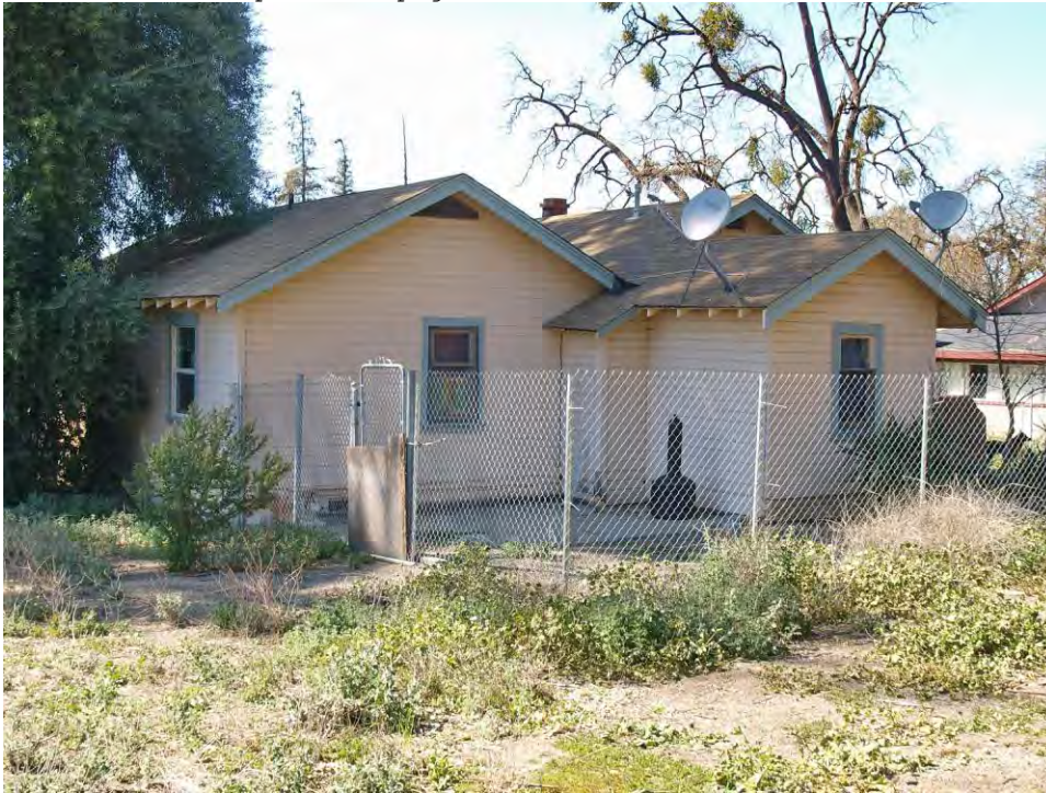
Rear of house, viewed facing west.
