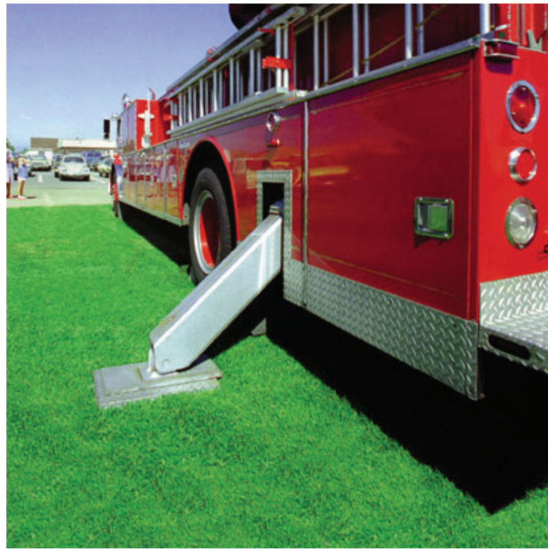
GC-1: LAWN OVER “GRASSPAVE” WITHIN FIRE LANE. (PHOTO BY INVISIBLE STRUCTURE INC.)
