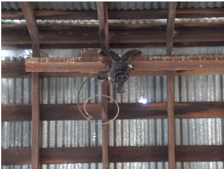
Figure 16. Remnants of hay pulley system (Garavaglia Architecture, Inc., April 2018)
