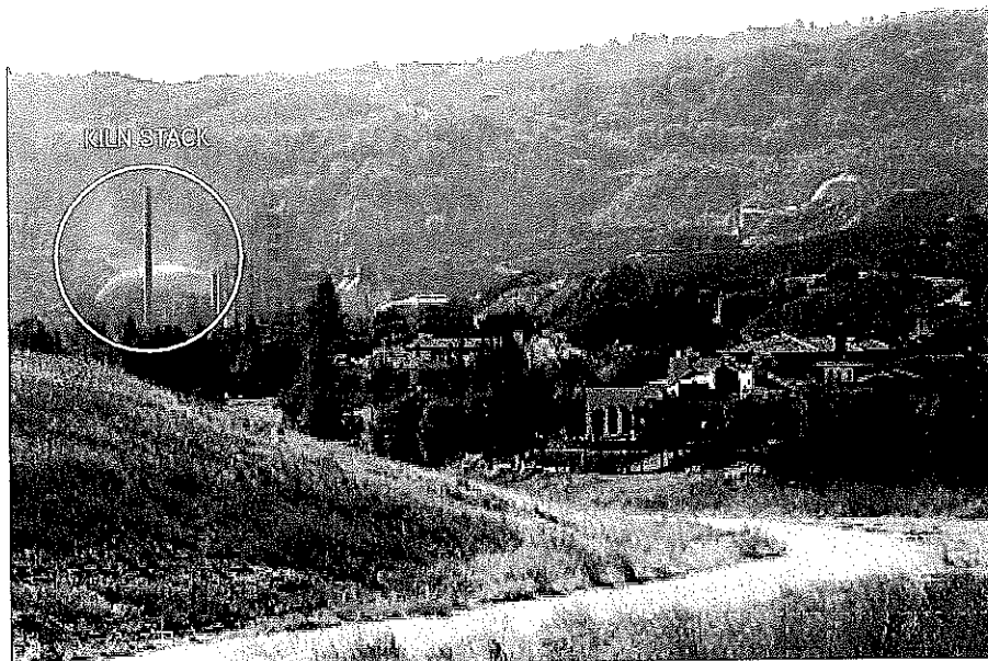
After Cooler and Kiln Stacks
