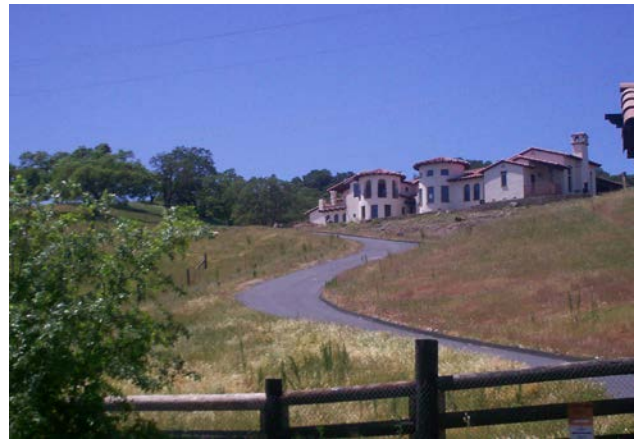
PHOTOS 3, 4: Design access roads and driveways to follow natural grade, contour and topography.
