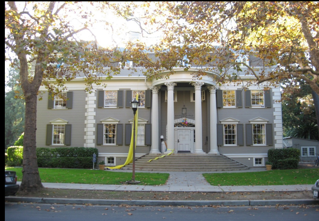
Rehabilitation 2013 Photo Credits: Stanford University
