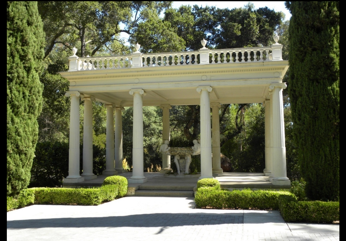
Love Temple after Restoration: Photo Credits: Montalvo Arts
