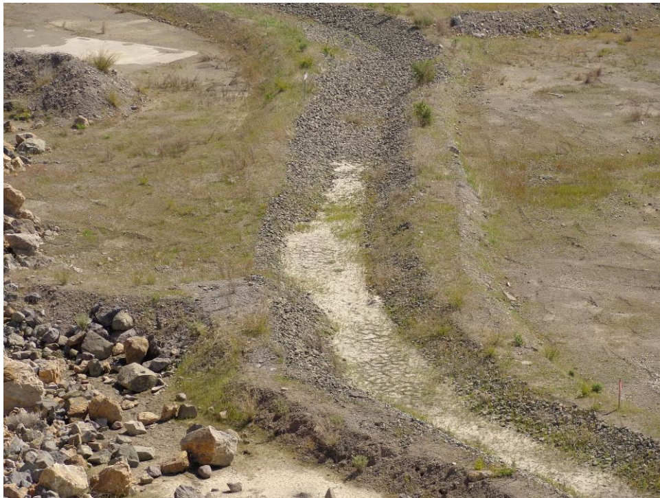
Above: Photo 5; deficiency 6. Water ponding on access road north of Pond 13. Map 2a.
