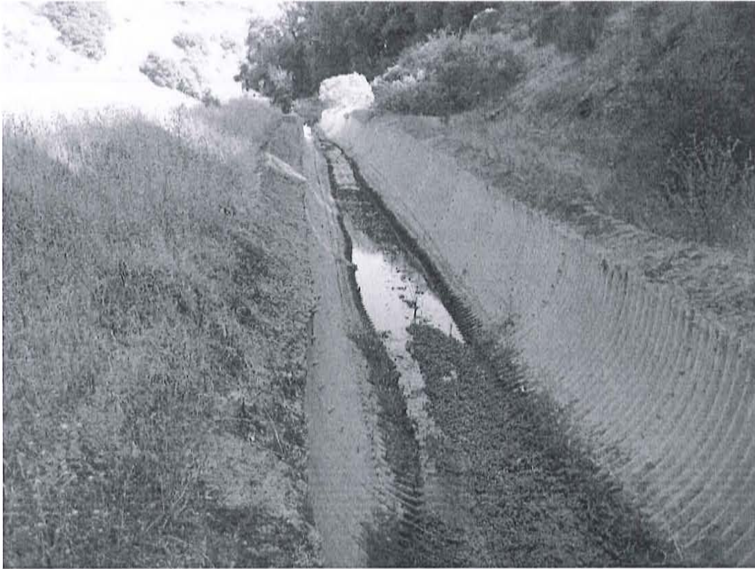
Photo 9: Discharged area from Pond 13 into Permanente Creek (open culvert).
