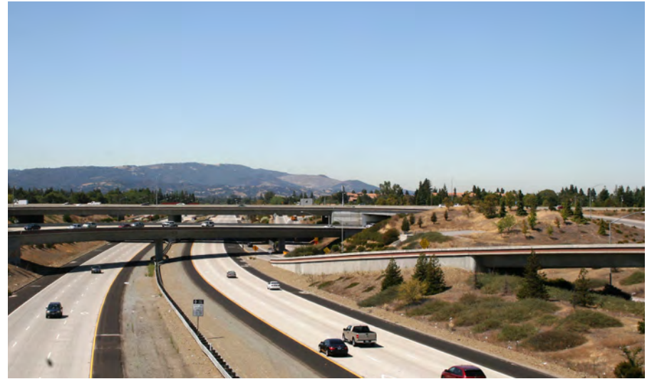
Photo 2: Bascom Avenue overpass looking northwest over State Route 85
