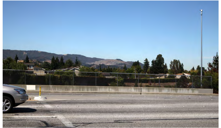
Photo 6: Northbound De Anza Boulevard on the State Route 85 overpass, looking west
