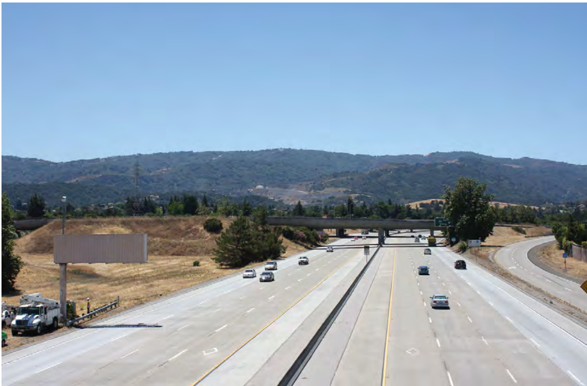
Existing view from Mary Avenue Bicycle Footbridge looking southwest over Interstate-280
