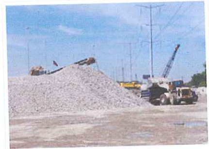
Recycled crushed concrete being loaded into a semi-dump truck to be used as granular fill.
