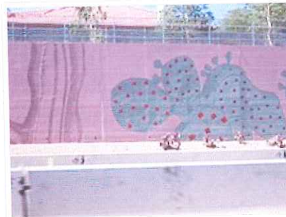
40-foot cacti decorate a sound/retaining wall in Scottsdale, Arizona
