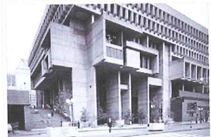
A modern building: Boston City Hall (completed 1968) is constructed largely of concrete, both precast and poured in place.
