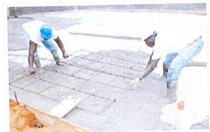
Installing rebar in a floor slab during a concrete pour.
