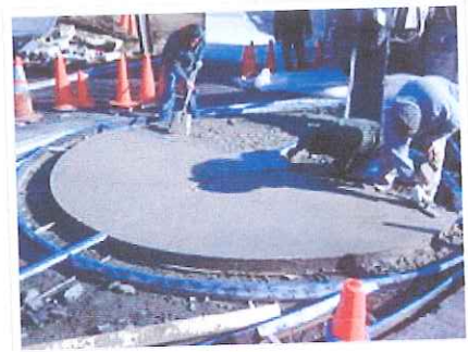
Pouring and smoothing out concrete at Palisades Park in Washington DC.
