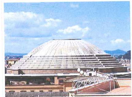
Outer view of the Roman Pantheon, still the largest unreinforced solid concrete dome. [1]
