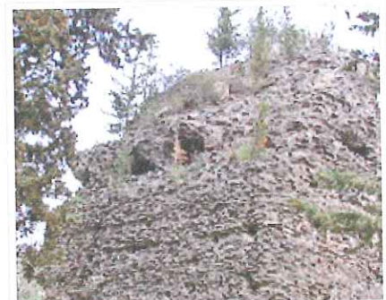
Opus caementicium lying bare on a tomb near Rome. In contrast to modern concrete structures, the concrete walls of Roman buildings were covered, usually with brick or stone.
