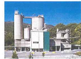
Lafarge cement plant in Contes, France.
