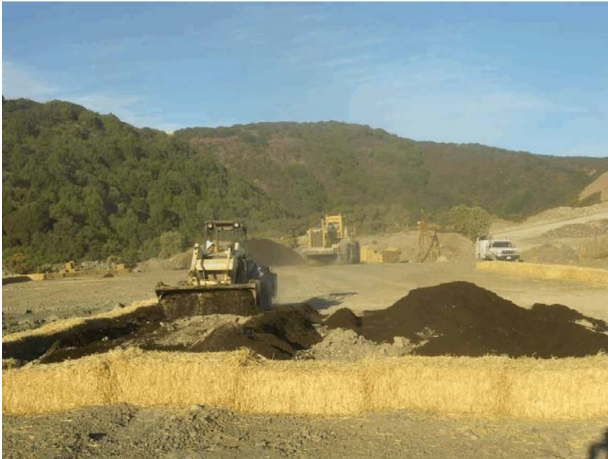
Top: Test Plot Construction at Yeager Yard Site: Applying Compost
