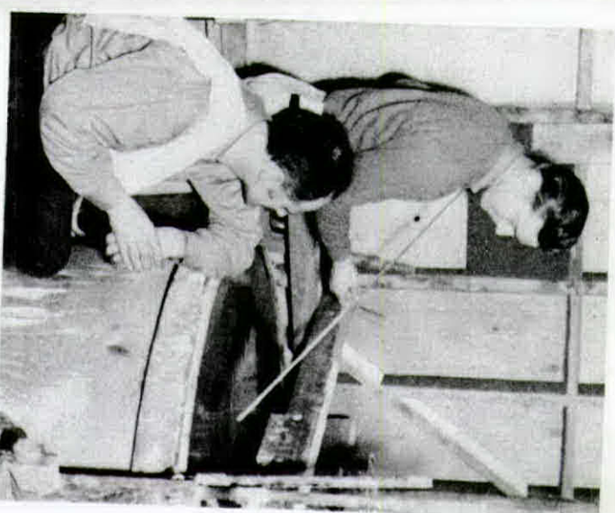
In the Moss Landing pilot plant, where operating conditions are duplicated in miniature, Fred DeMaestri draws a sample from the bottom of the tank for "Woody" Woodward of the Engineering and Development Division of Oakland. "Woody" is doing special research at Moss Landing.
