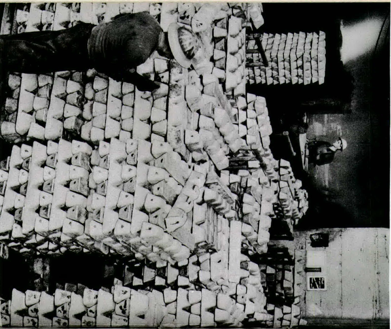
Headaches for Hitler: The camera's eye catches a portion of a day's production stacked in a corner of the ingot handling room of the Permanente foundry. After laboratory analysis, this magnesium will be shipped by boxcar and truck and soon will be transformed into airplane parts or into incendiary bombs. Joe Baltrun daubs varicolored spots of paint on the ingots to indicate different types of alloys, as Lawrence Schroyer , jeep operator, warps another stack onto the scale platform.
