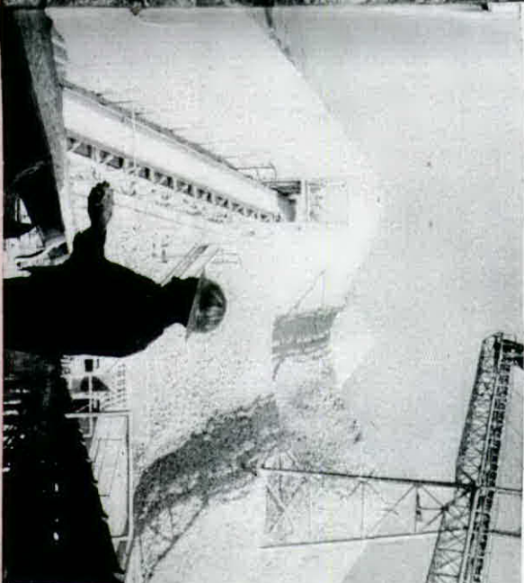
SILHOUETTED against the plant background, a Natividad employee checks the endless procession of crushed dolomite. From the kiln feed bins, the white rock is fed to the plant's two kilns and calcined at a temperature of 1800 degrees. F.
