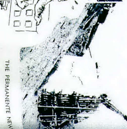
August 15, forms are ripped off first kiln block.
