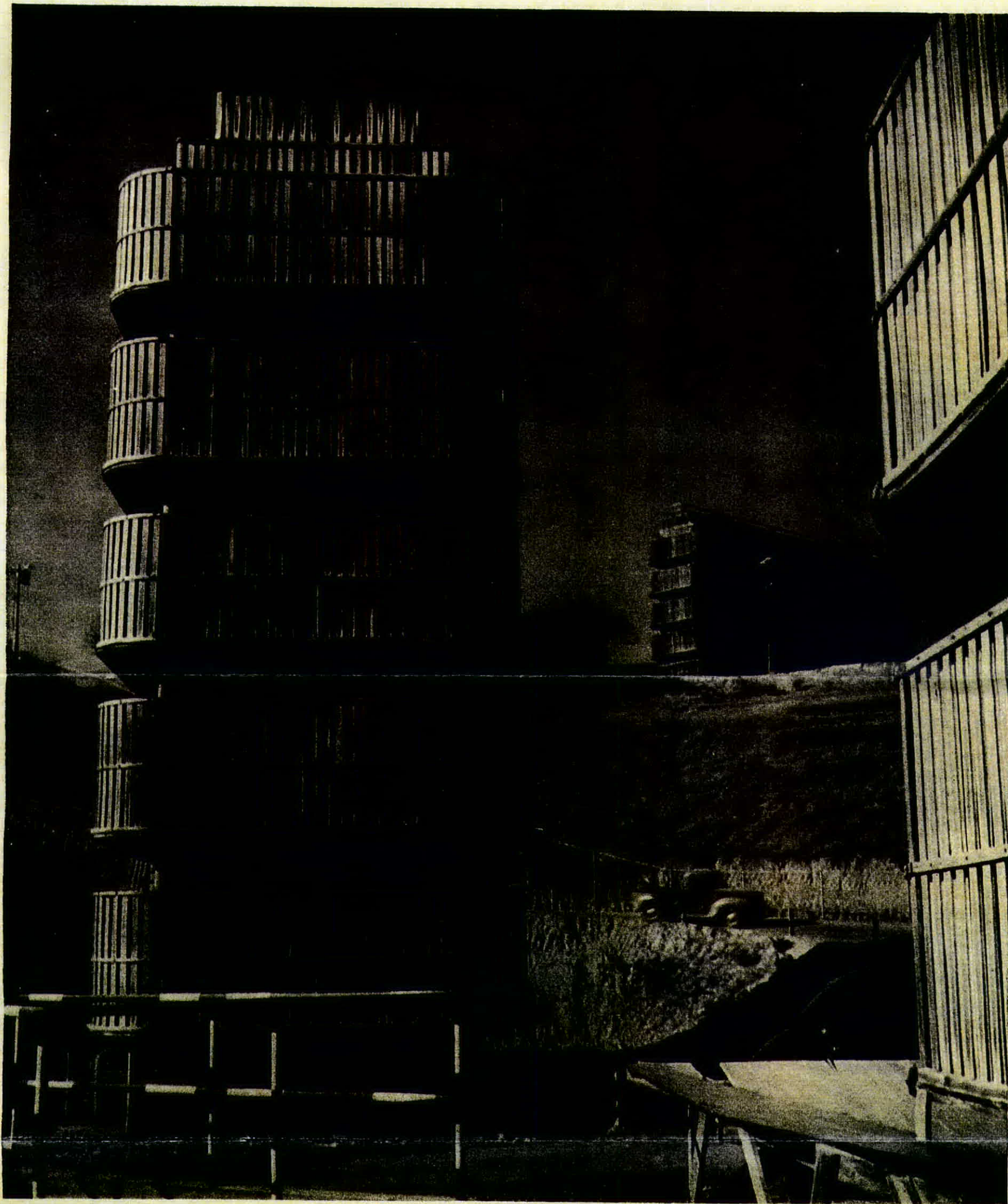
CONDENSER TOWERS COOL NATURAL GAS WHICH CHILLS MAGNESIUM VAPOR INTO DUST AS IT EMERGES FROM FURNACE. GAS, AFTER SEVERAL CYCLES, IS BURNED IN CEMENT KILNS
