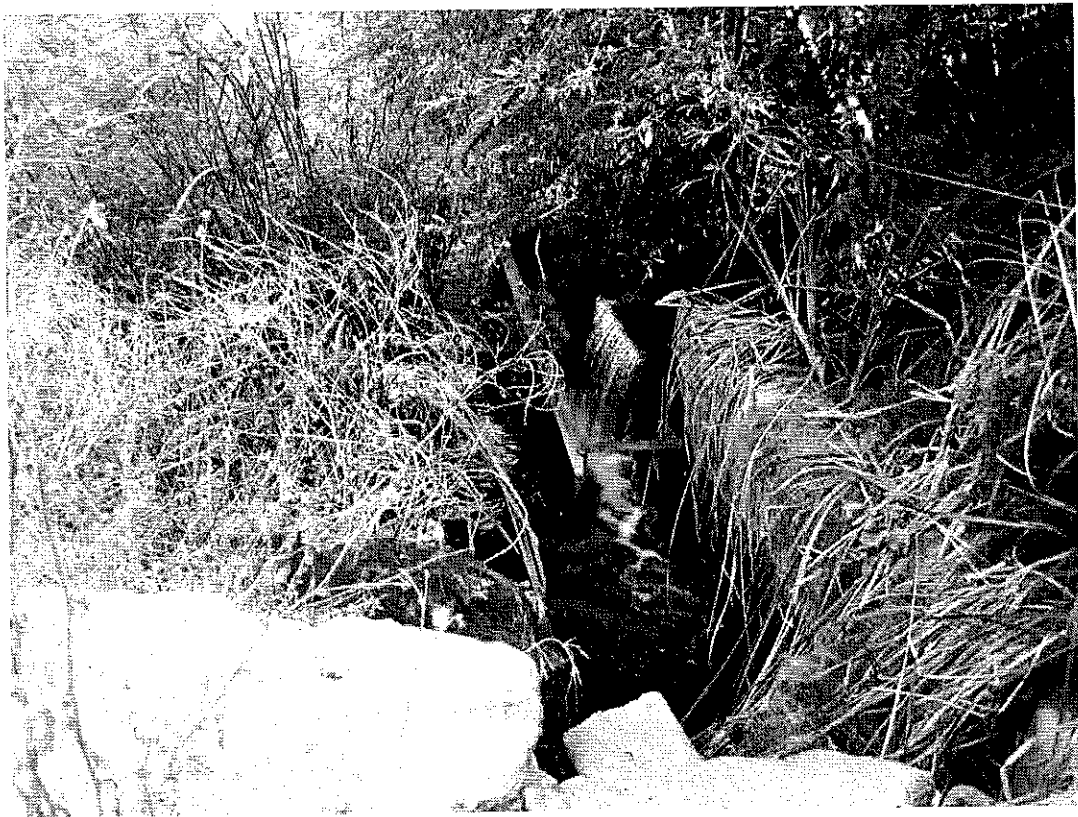
Photo 10: View of Pond 14 and the diversion structures which allows water to flow to Pond 22.
