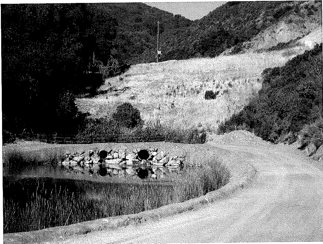
Photo 2: View of outfall from Rattlesnake Creek.
