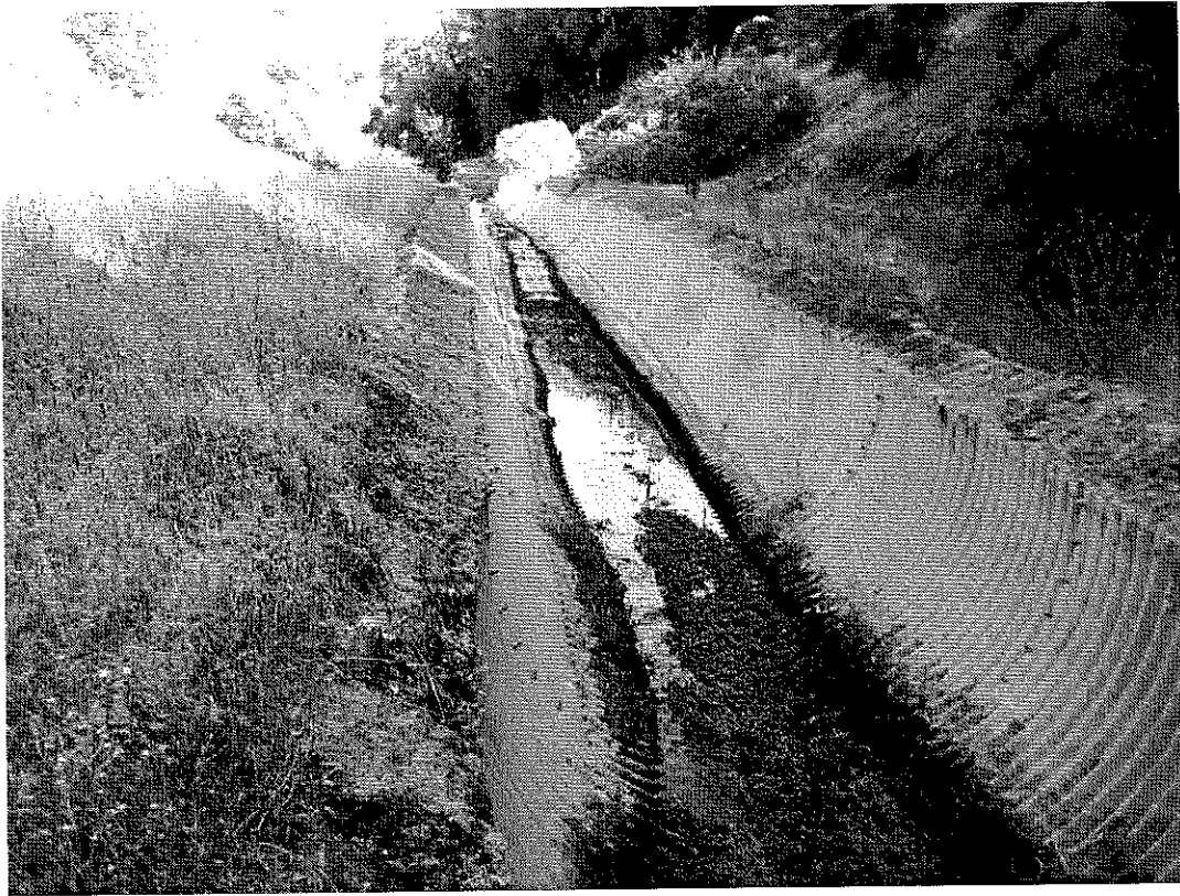
Photo 9: Discharged area from Pond 13 into Permanente Creek (open culvert).
