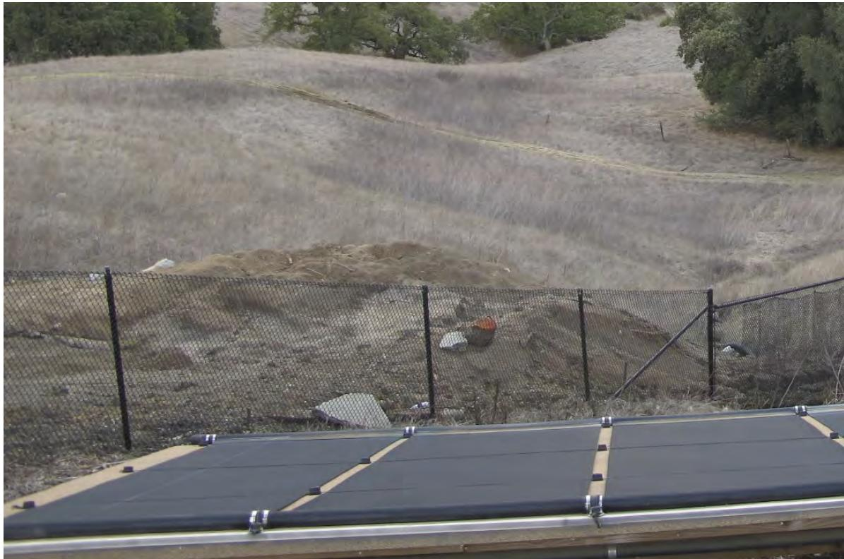
Photo showing the recent mudslide on the subject property that occurred where soil was added, and where the previously installed drain pipe is above grade and detached.
