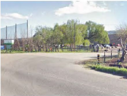
② View looking towards main project site entrance from SR 25
