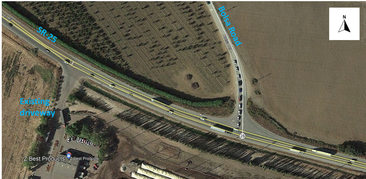
Figure 1: Existing 3-leg intersection of Bolsa Road and SR-25.
