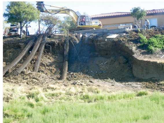
Example of a Stitch Pier Wall under construction
