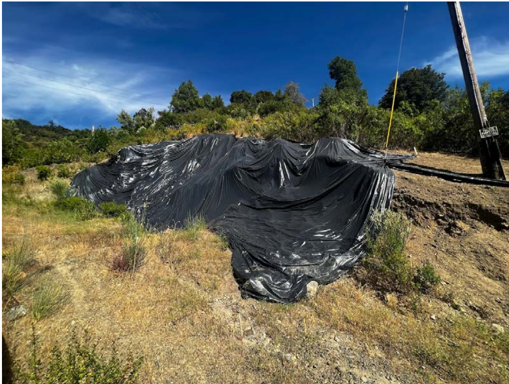
Photo 2 and 3. Representative photos of some of the areas where there appears to have been vegetation removal and grading activities. These areas have been affected by erosion and much of this area is covered with plastic sheeting.
